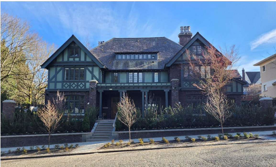
Figure 2: The Bloch Residence today, 2022. (Author's photo.)
