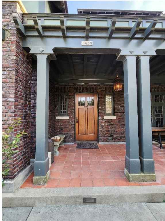
Figure 19: Primary entrance, 2023. (Author's photo.)
