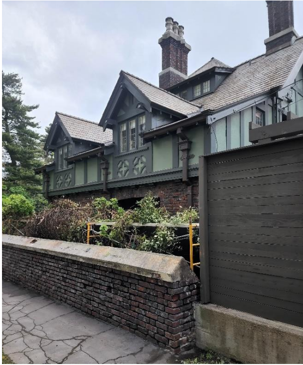
Figure 29: West elevation viewed from the southwest, taken during site construction, 2022. (Author's photo.)
