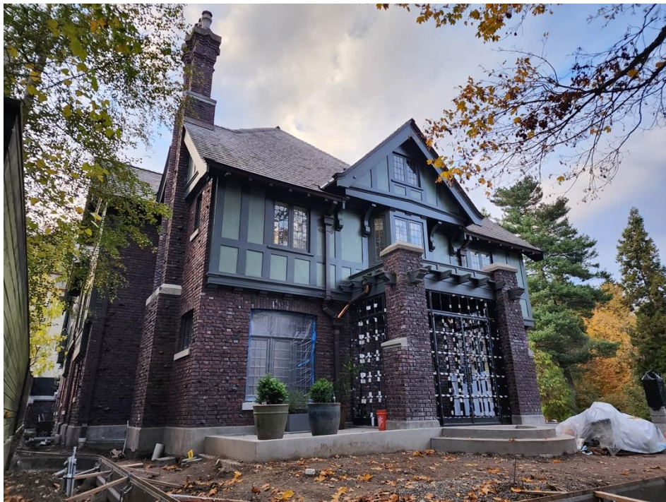
Figure 22: Southeast corner of the house, 2022. (Author's photo.)
