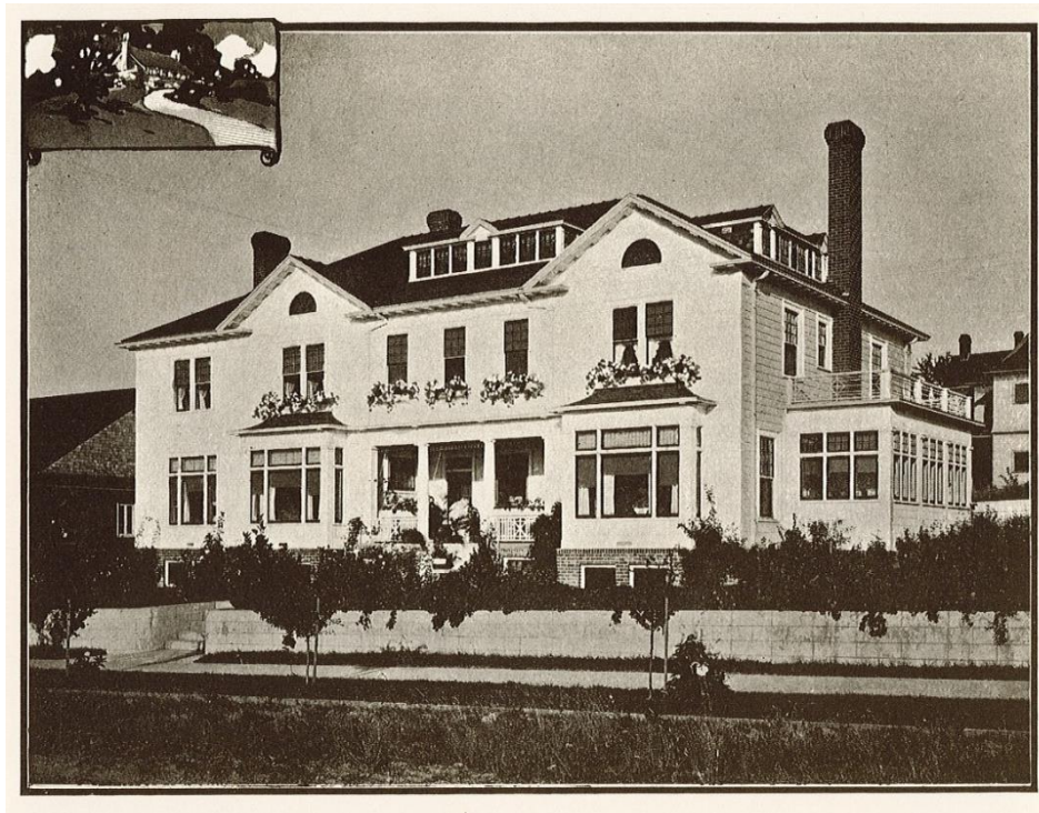
Figure 84: Wilson & Loveless, Kennedy Residence, 1909 (existing). (Frank Calvert editor, Homes and Gardens of the Pacific Coast , v. 1, Beaux Arts Village, Lake Washington, 1913.)
