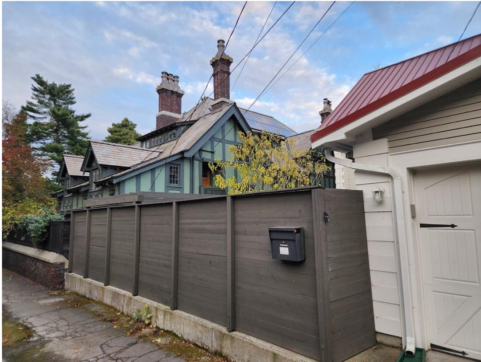
Figure 26: Southwest corner of the house, 2022. (Author's photo.)
