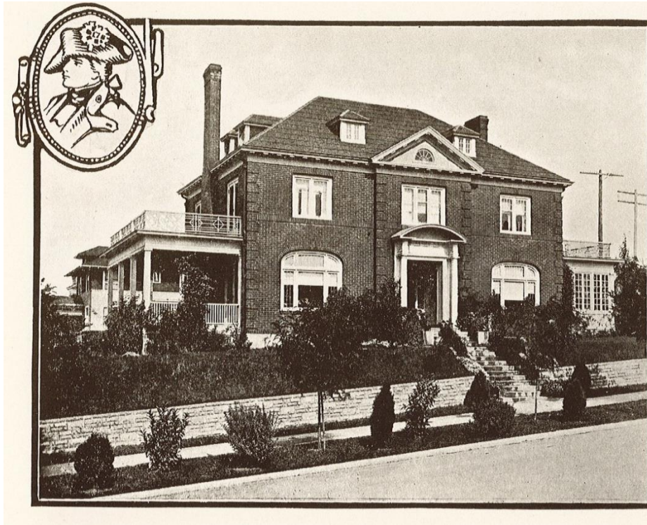
Figure 85: Wilson & Loveless, Sparkman Residence, 1909 (existing). (Frank Calvert editor, Homes and Gardens of the Pacific Coast , v. 1, Beaux Arts Village, Lake Washington, 1913.)
