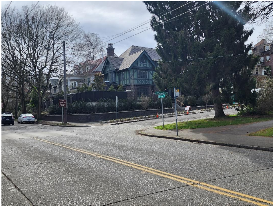
Figure 11: The Bloch residence is very prominent when viewed from the southeast corner of Fifteenth Avenue East and East Prospect Street, 2023. (Author's photo.)
