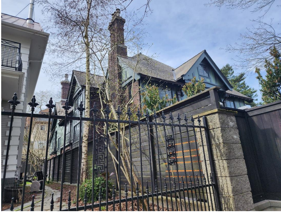
Figure 25: Southeast corner of the house, 2023. (Author's photo.)
