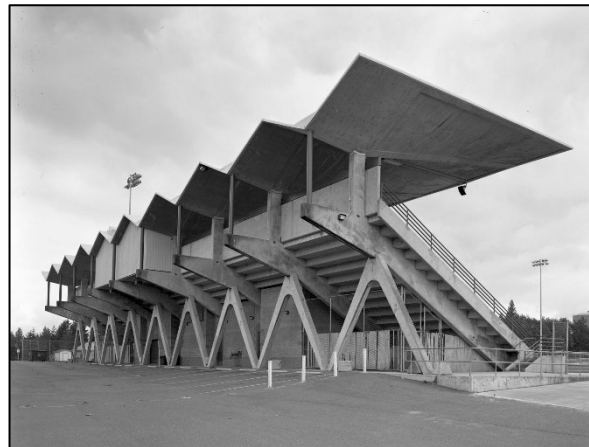
Innovative examples of thin-shell concrete stadiums in Washington State include the Grant County Stadium (1963), below left, designed by Jack Christenson, structural engineer, and his Bainbridge Island High School Stadium (1990).
