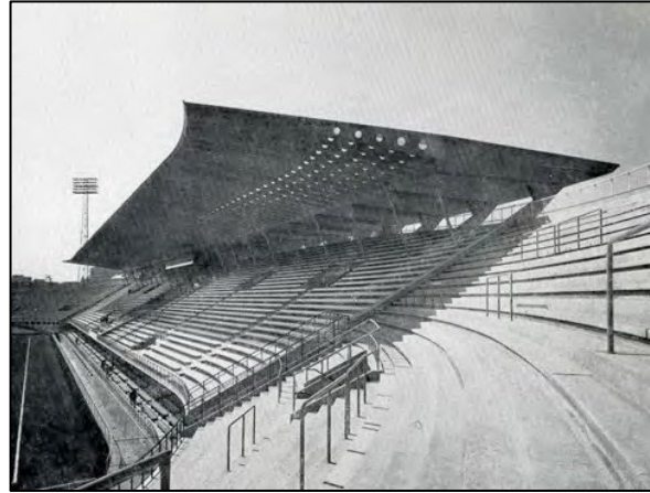
Left, Florence Municipal Stadium, 1930-1931, 35,000 seat facility, with reinforced concrete bifurcating cantilevered beams. Right, the Olympic Flaminio Stadium, Rome (1957-1959), with 45,000 seats, with prefabricated concrete beams and corrugated cantilevered concrete roof. Both were influential designs by Pier Luigi Nervi.
