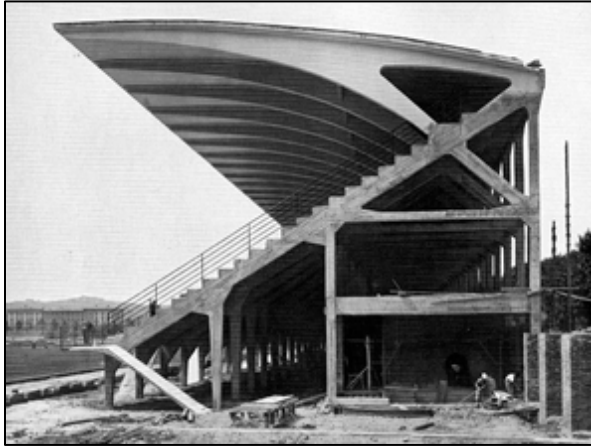
Left, Florence Municipal Stadium, 1930-1931, 35,000 seat facility, with reinforced concrete bifurcating cantilevered beams. Right, the Olympic Flaminio Stadium, Rome (1957-1959), with 45,000 seats, with prefabricated concrete beams and corrugated cantilevered concrete roof. Both were influential designs by Pier Luigi Nervi.
