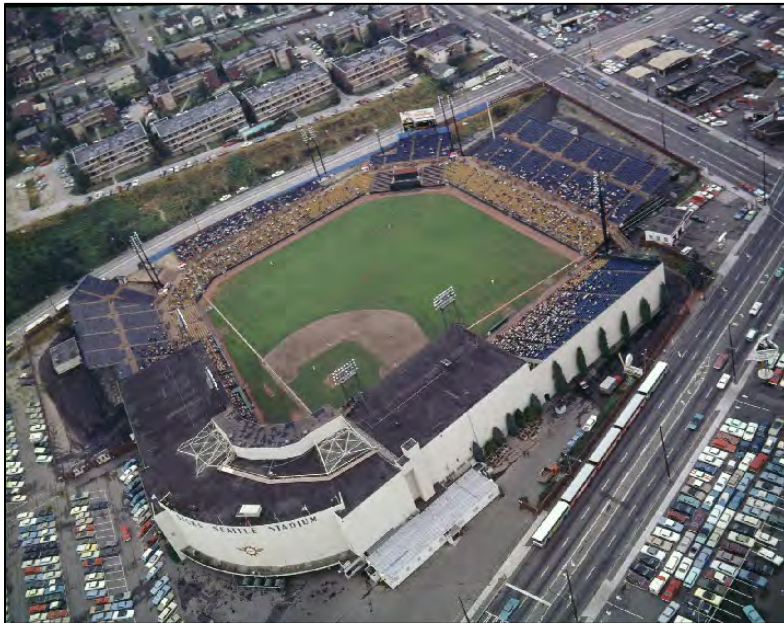
The composite structure of Sick's Stadium (1938-79)
