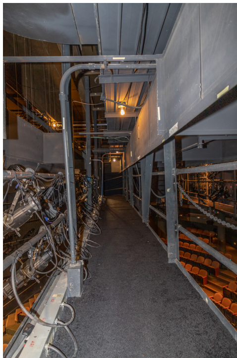
Figure 56. Playhouse Theater, added catwalk looking north, with the original catwalk visible above.
