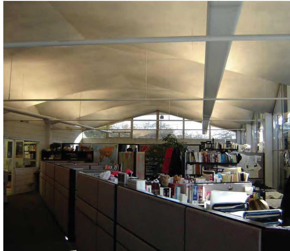
INTERIOR VAULTING OF THIN SHELL CONCRETE ROOF
