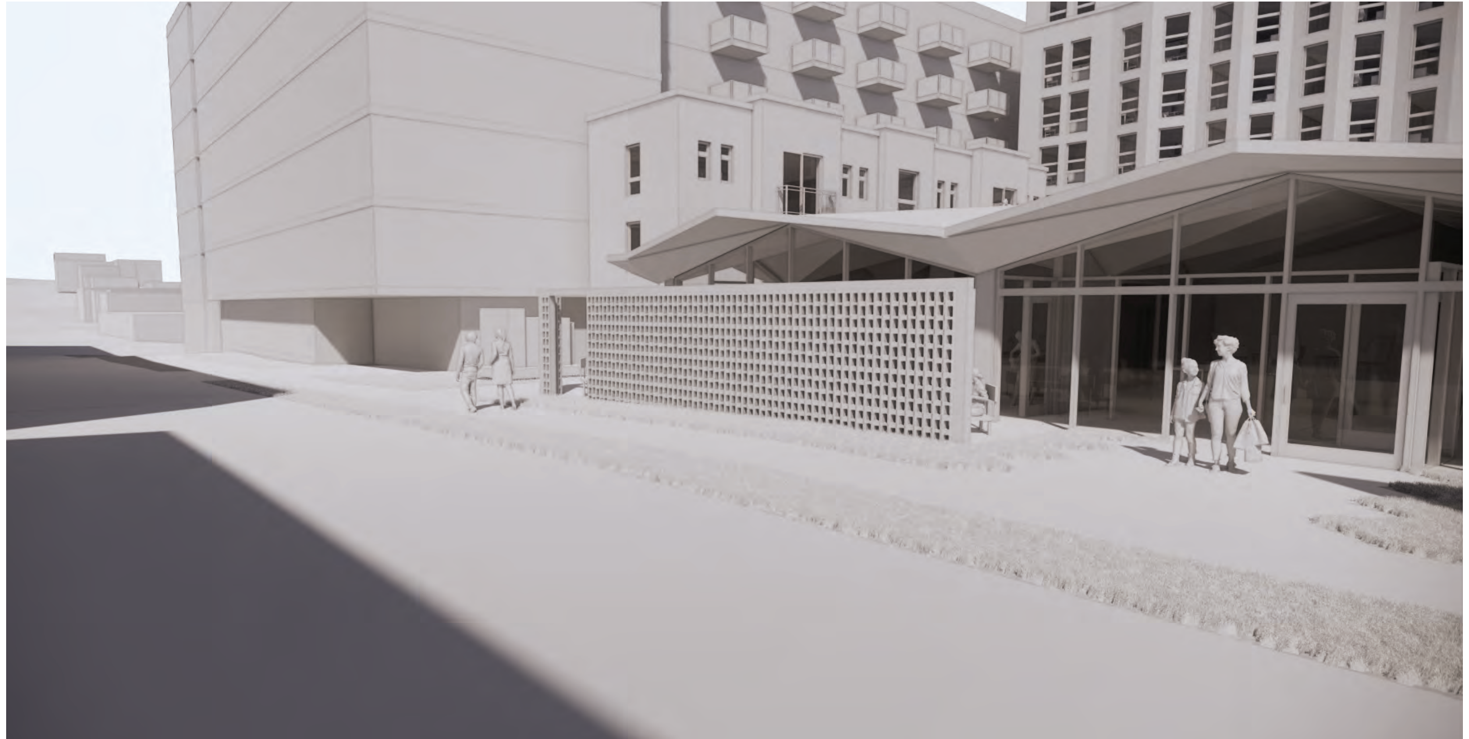
RENOVATIONS IN THE 90S REMOVED A PORTION OF BREEZEBLOCK ALONG 38TH STREET, BUT THE SCREEN WALL PRESENTS A PRONOUNCED BARRIER TO THE STREET.
