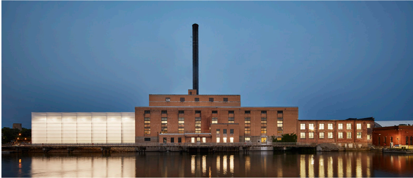
Beloit College Power House Wisconsin
