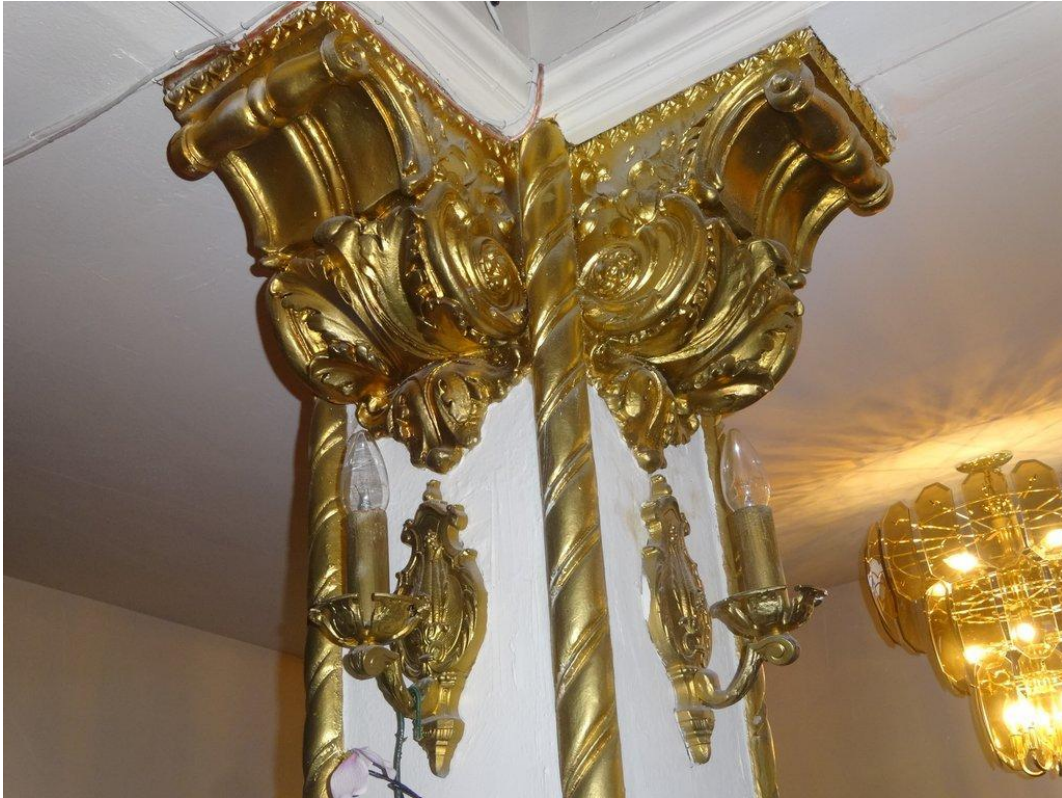
B25. Detail of a column capital in the sanctuary. May 7, 2021.
