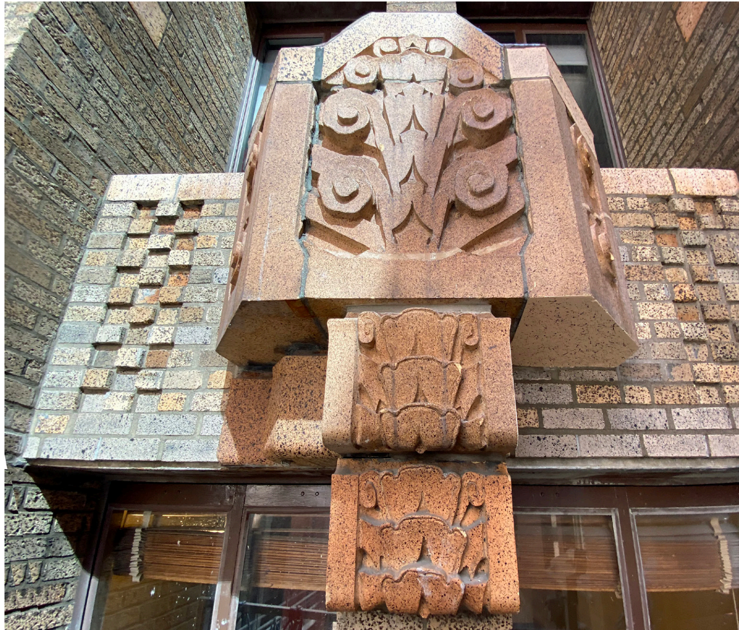
DETAIL OF LINTEL WITH TERRACOTTA ACCENT PIECE REMOVED AND PATCHED WITH BRICK TO MATCH EXISTING SURROUNDING FIELD BRICK. LEFT SIDE SHOWS ORIGINAL ACCENT PIECE FOR COMPARISON.
