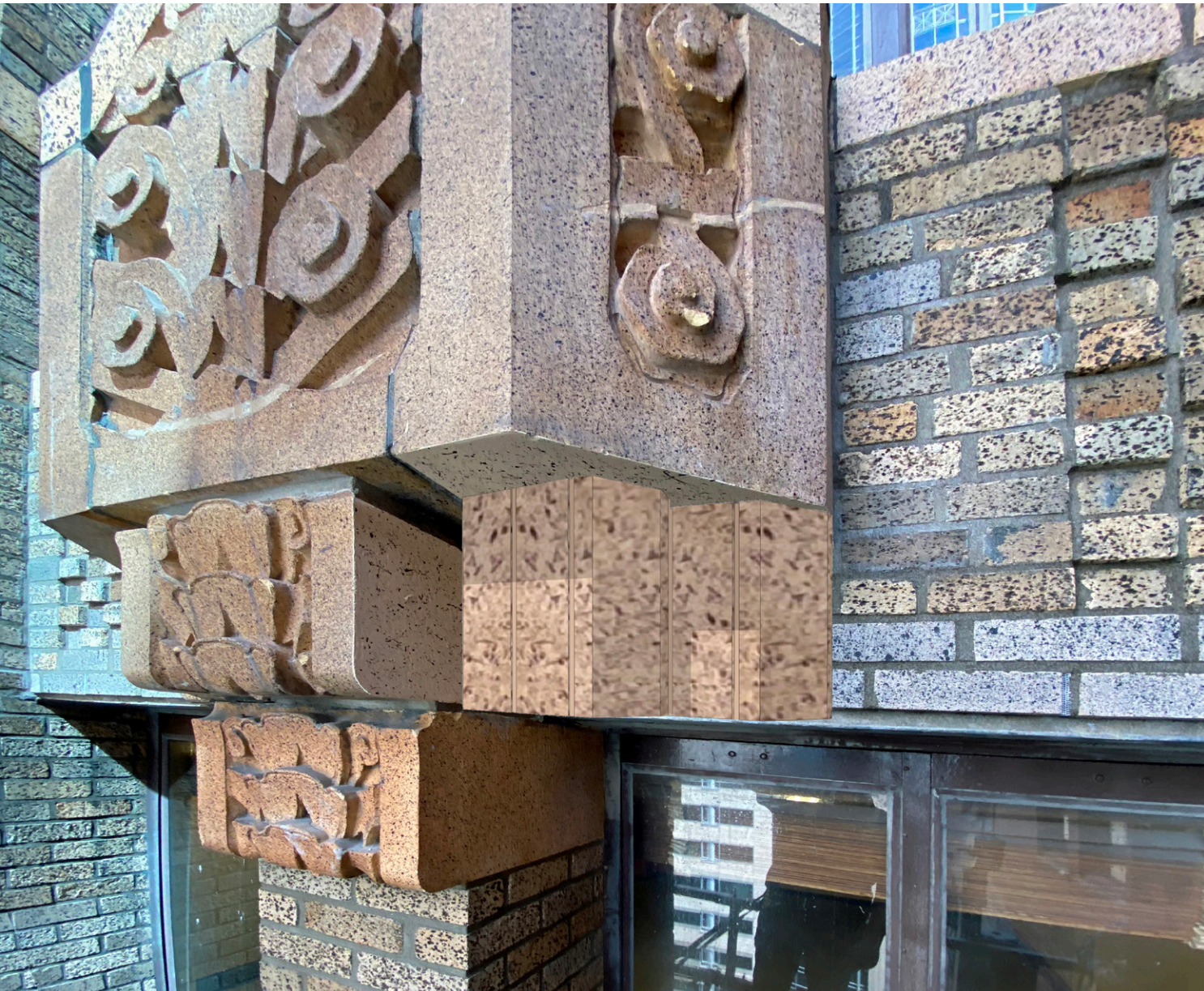
DETAIL OF LINTEL WITH TERRACOTTA ACCENT PIECE REMOVED AND REPLACED WITH COLOR MATCHED BRICK TO MIMIC EXISTING SUPPORT SHAPE. THE GROUT WOULD BE COLOR MATCHED TO BRICK TO MAKE THE ACCENT BRICK APPEAR AS MONOLITHIC AS POSSIBLE. THE LEFT SIDE SHOWS ORIGINAL ACCENT PIECE FOR COMPARISON.
