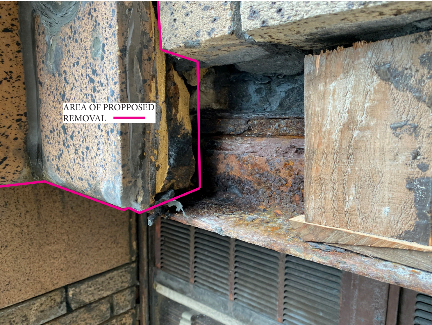
DETAIL OF DAMAGE AT LINTEL, BRICK, AND TERRACOTTA MEDALLION INTERFACE, TYPICAL OF ALL LOCATIONS TO VARYING DEGREES.
