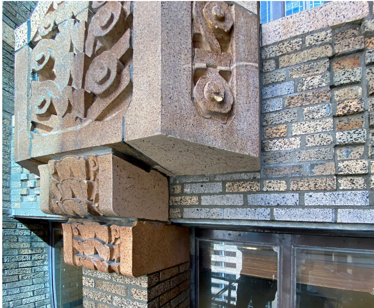
DETAIL OF LINTEL WITH TERRACOTTA ACCENT PIECE REMOVED AND PATCHED WITH BRICK TO MATCH EXISTING SURROUNDING FIELD BRICK.
