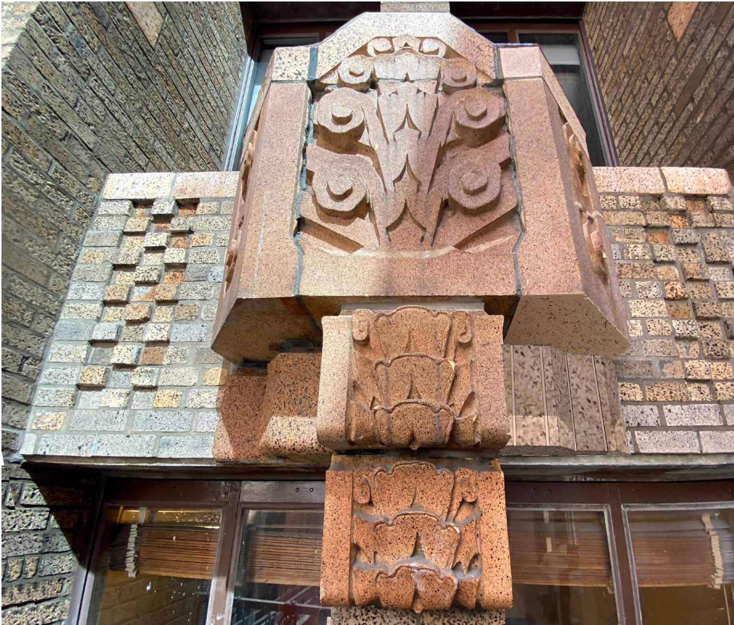
DETAIL OF LINTEL WITH TERRACOTTA ACCENT PIECE REMOVED AND REPLACED WITH COLOR MATCHED BRICK TO MIMIC EXISTING SUPPORT SHAPE. THE GROUT WOULD BE COLOR MATCHED TO BRICK TO MAKE THE ACCENT BRICK APPEAR AS MONOLITHIC AS POSSIBLE. THE LEFT SIDE SHOWS ORIGINAL ACCENT PIECE FOR COMPARISON.
