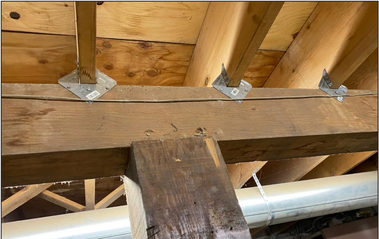
Figure 25 • 3414-3416 Fremont Avenue N, interior southern side sub-basement showing new floor framing
