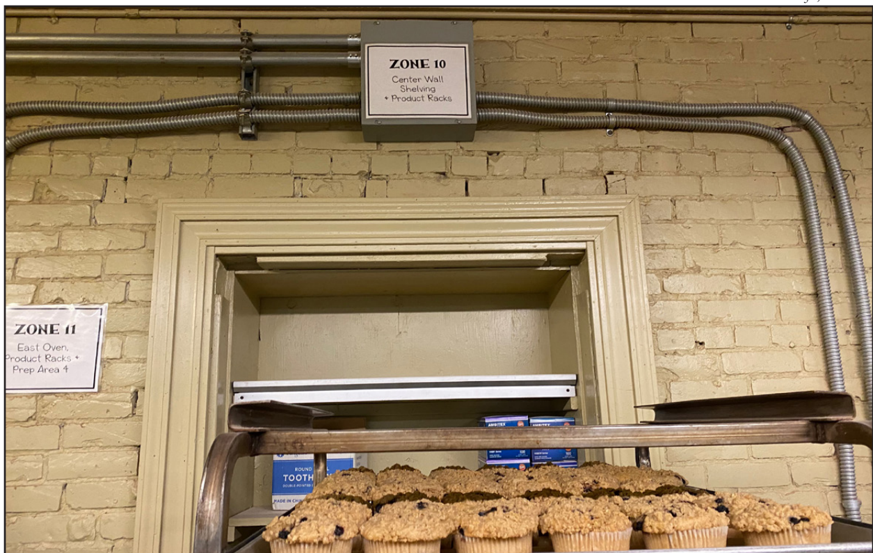
Figure 31 • 3414-3416 Fremont Avenue N, interior basement, northern side showing URM wall with former door to southern side basement.
