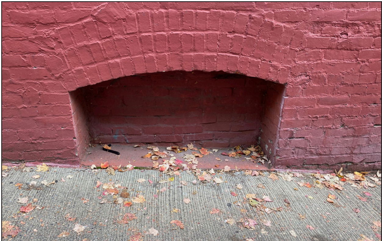
Figure 18 • 3414-3416 Fremont Avenue N, detail of infilled window on southern façade
