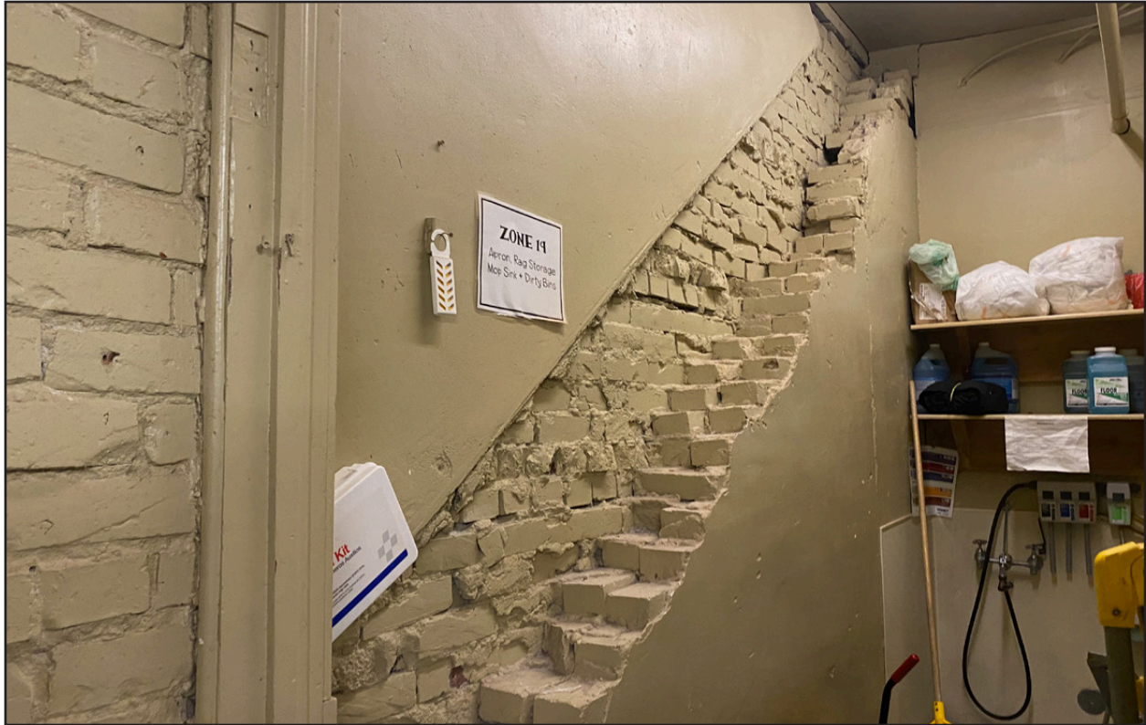
Figure 32 • 3414-3416 Fremont Avenue N, interior basement, northern side showing URM wall evidence of alteration.
