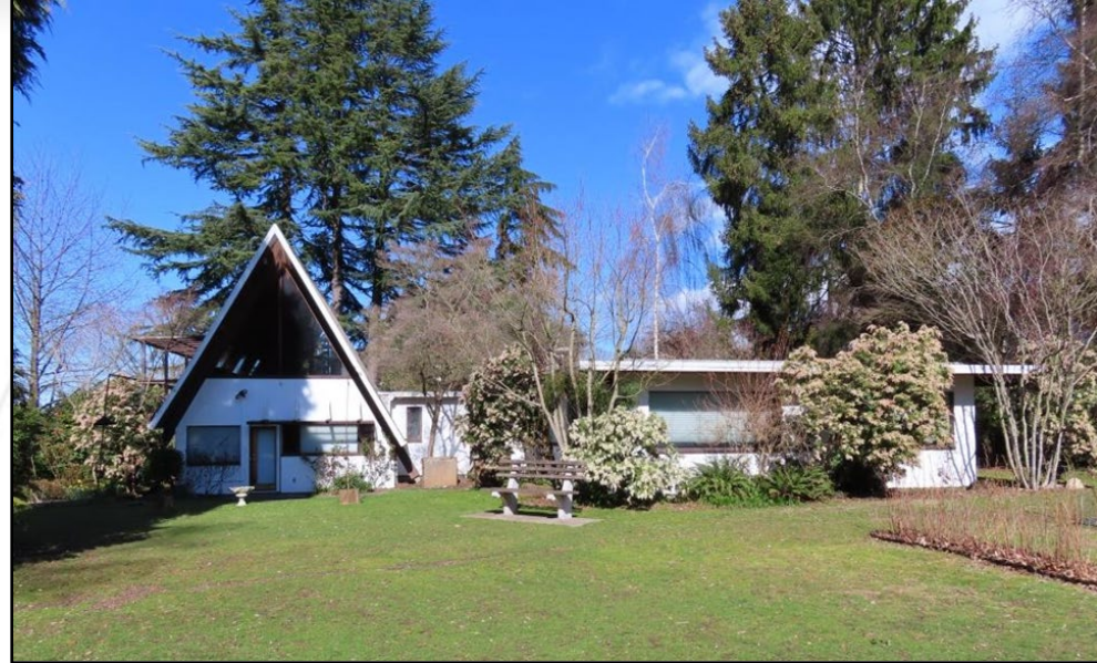
Bullitt House, south elevation, 2022.
