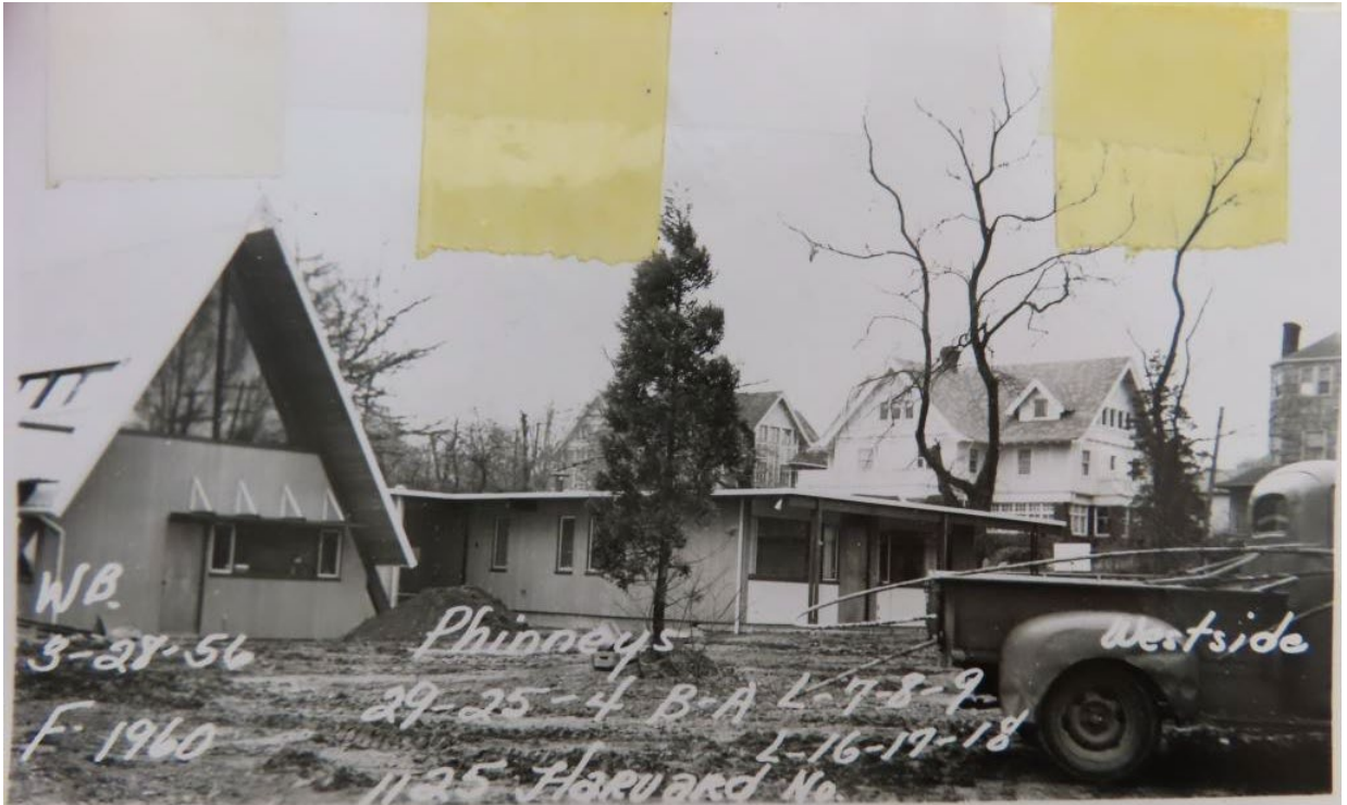
Figure 10. King County Assessor's photo of the Bullitt House, 1125 Harvard Avenue E, 1956, view northeast.
