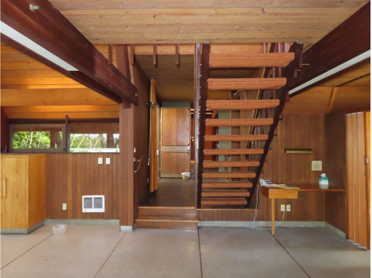
Photograph 22. Terrazzo floors, stair to loft, and front entry with slate floors, Bullitt House, 1125 Harvard Avenue E, view east.
