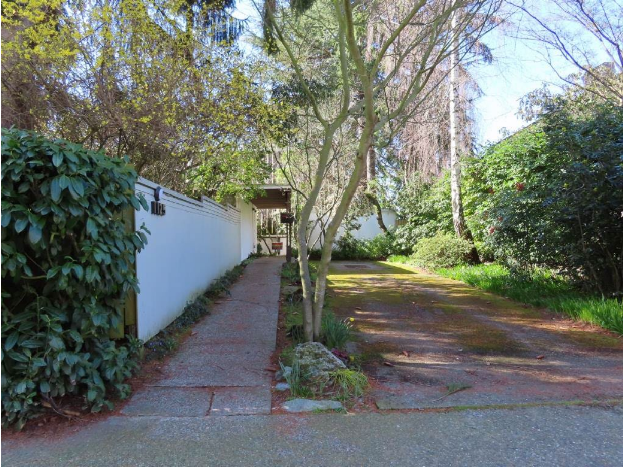
Photograph 1. The Bullitt House, 1125 Harvard Avenue E, as viewed from Harvard Avenue E, view west.
