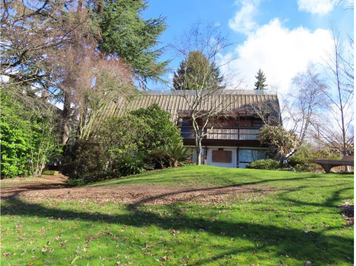
Photograph 9. The west elevation of the Bullitt House, 1125 Harvard Avenue E, view east.
