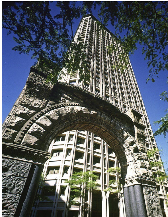
Figure 24. The Henry M. Jackson Federal Building, designed by Fred Bassetti, and John Graham, with Richard Haag, completed 1974. Photo courtesy of Clair Enlow, 2013. Daily Journal of Commerce.
