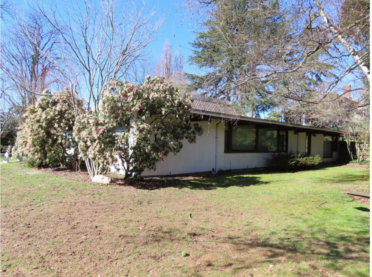
Photograph 11. The east elevation of the Bullitt House, 1125 Harvard Avenue E, view northwest.
