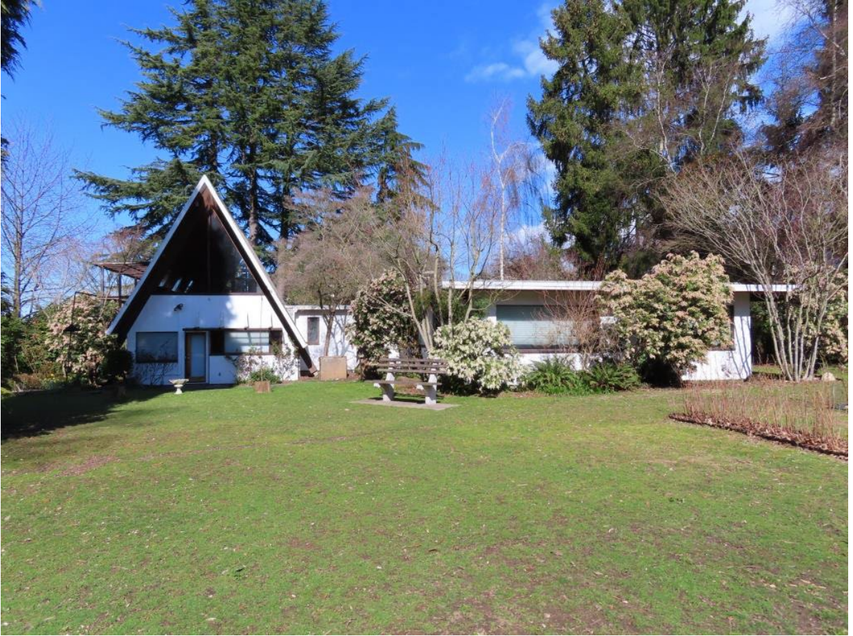
Photograph 10. The south elevation of the Bullitt House, 1125 Harvard Avenue E, view north.
