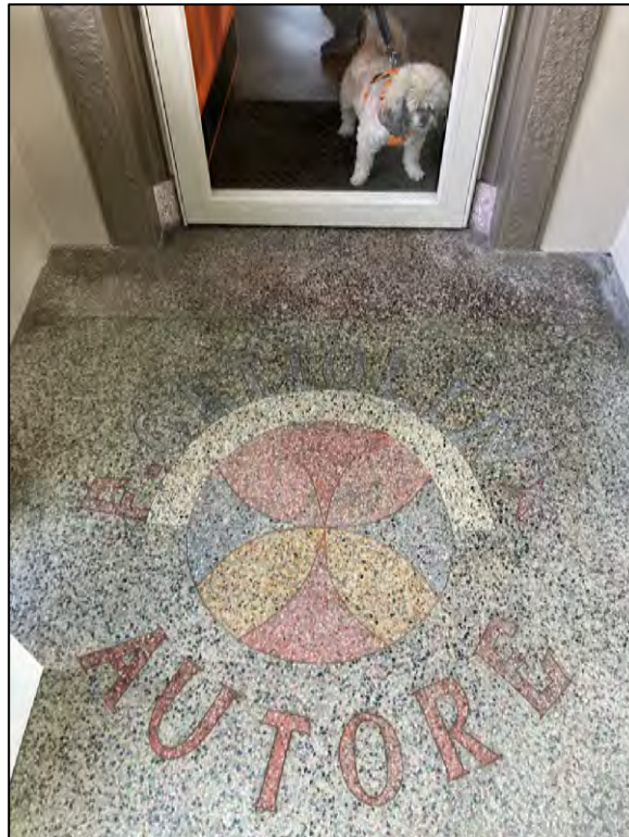
Fig. 11 – Front porch, detail of terrazzo paving, inscribed with center figure and “F. Cettolin, Autore” (meaning author or creator) in colored aggregate and binder.
