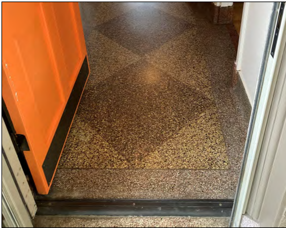
Fig. 28 – Interior, first floor corridor, detail of terrazzo.
