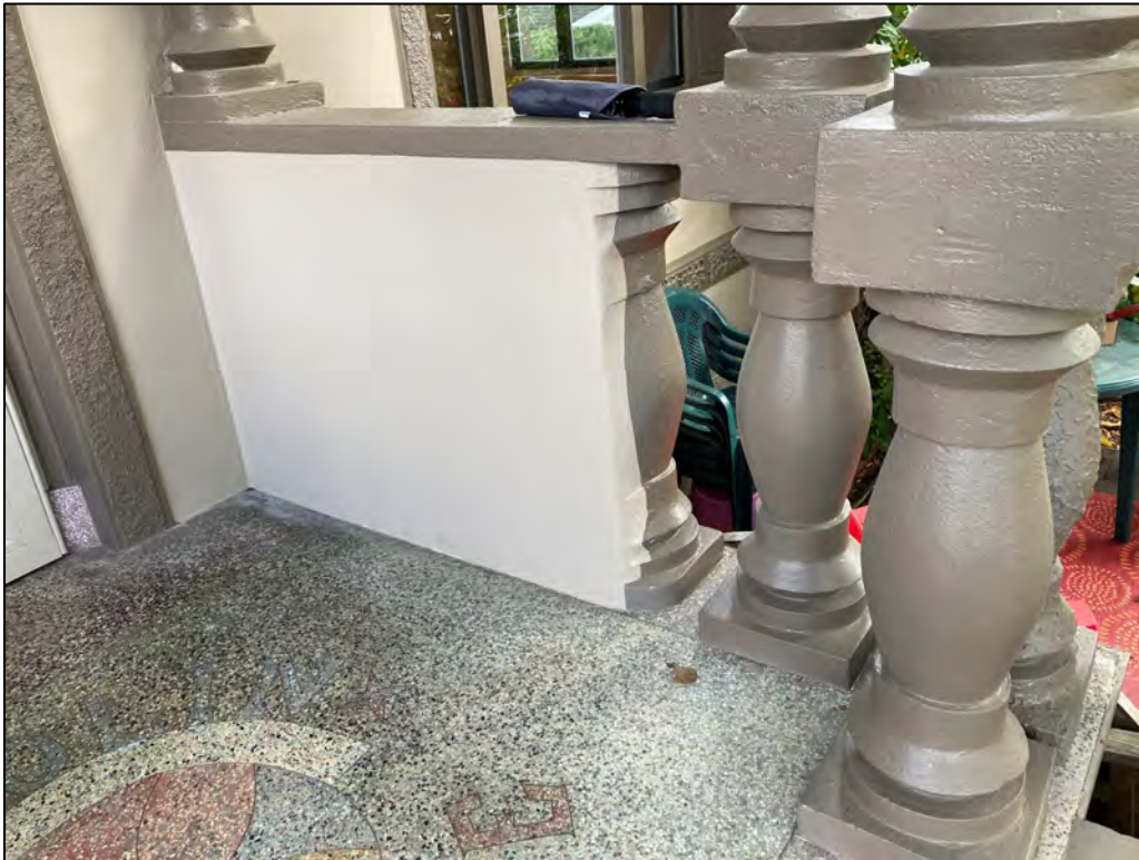
Fig. 9 – West facade, detail of front porch balustrade, interior side.
