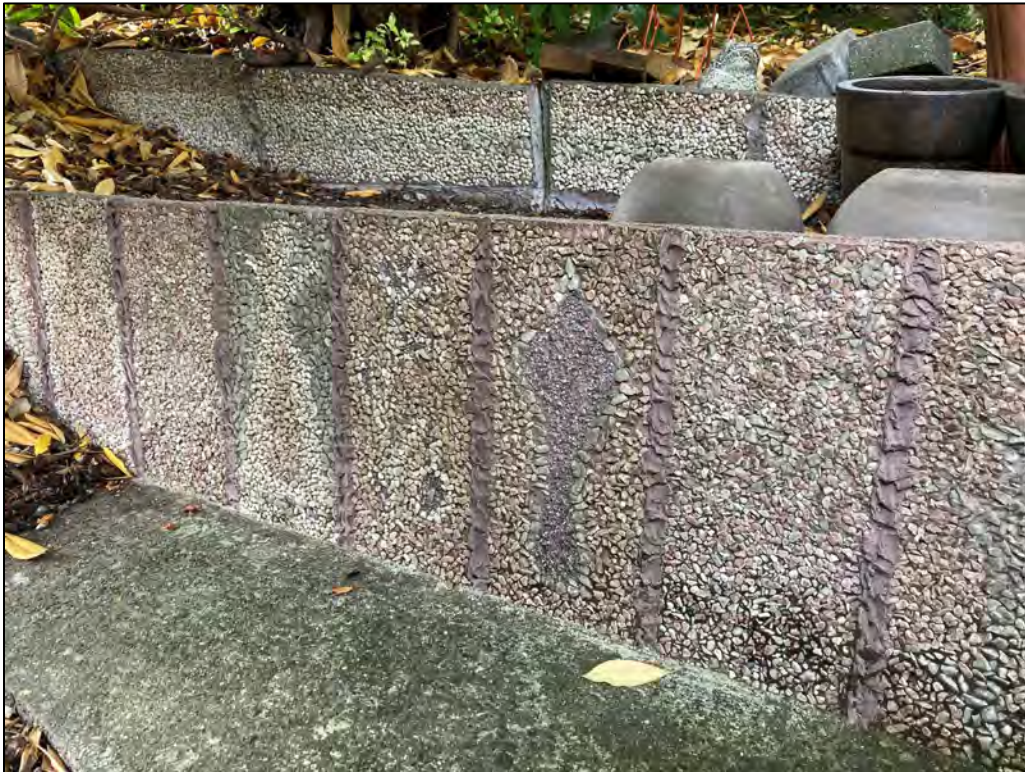
Fig. 25 – Pebble mosaic concrete tiles forming garden bed terraces, at front yard.
