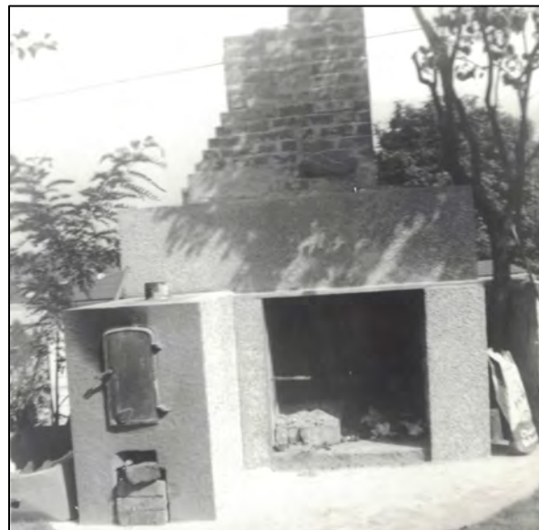
Fig. 98 - (Two photos) 1960s photos of the barbecue, located at the southeast corner of the original yard. Built by Fausto of brick and stucco. (No longer intact). (VC)
