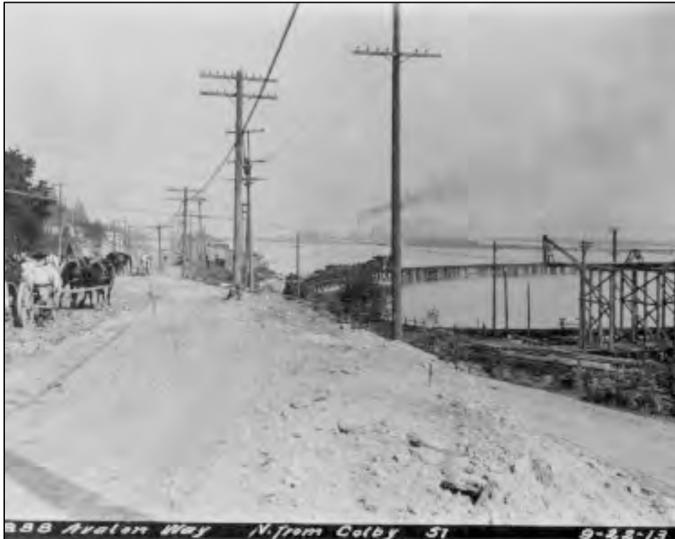
Fig. 53 - 1913 photo of the regrading of Avalon Way, showing view north. The Young's Cove tideflats, visible at right, are traversed by railroad trestles and have yet to be filled in. The steel mill is not visible, but is located just out of frame to the right. (SMA 6439)
