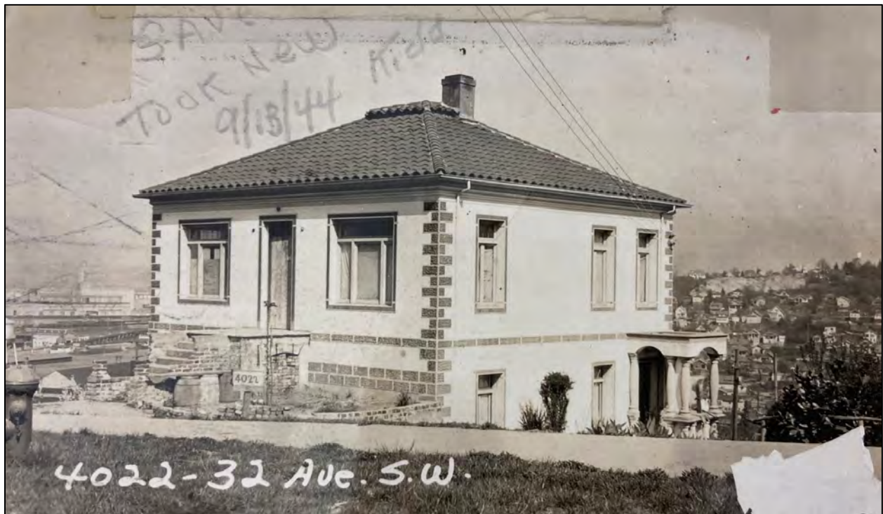
Fig. 73 – 1937 photo of the house, showing the completed decorative stucco work. Note the unfinished front porch. The side porch was the main entry for the family and Fausto, who worked down the hill at the steel mill, reached via the alley behind the house. (KCTA)
