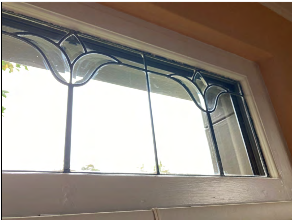
Fig. 32 – Interior, first floor, detail of typical tulip-motif leaded glass window transom used throughout the house.
