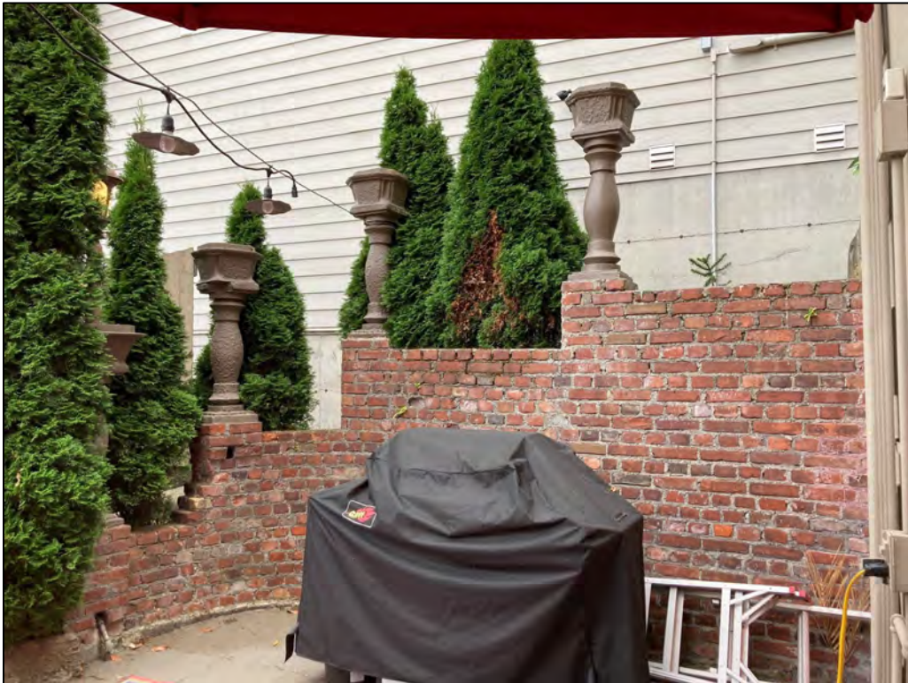
Fig. 19 – Rear yard, showing retaining wall at southwest building corner.
