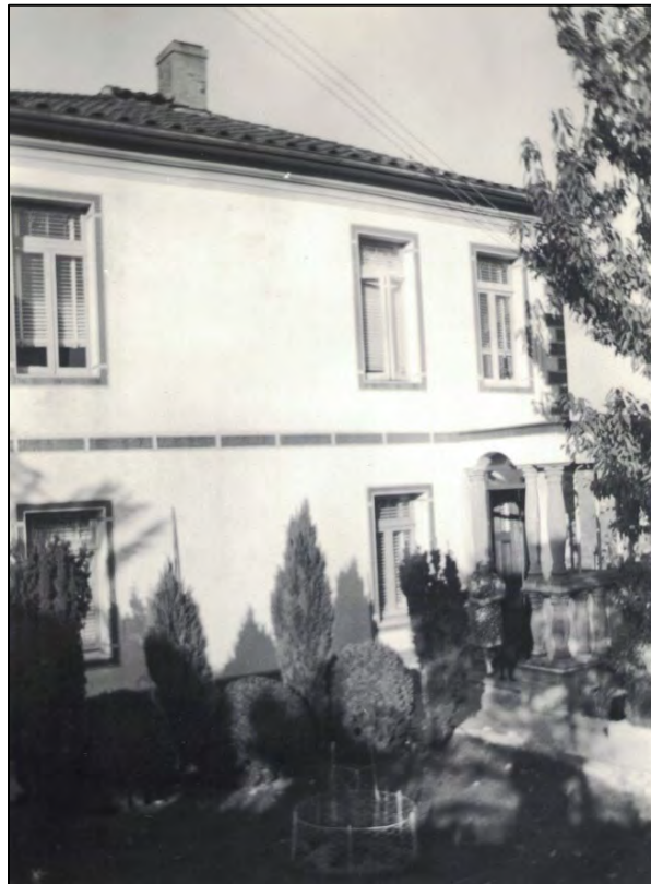
Fig. 78 - Ca. 1950s view of south facade. Erma Cettolin is visible at the side porch, and the small fenced area in the foreground was the location of the lily garden. (VC)
