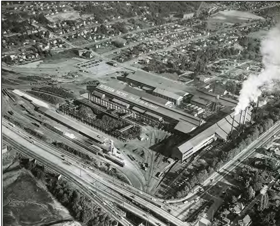
Fig. 57 – 1954 view southeast of the Bethlehem steel plant, now Nucor Steel, and Youngstown/Delridge. (MOHAI SHS11316)
