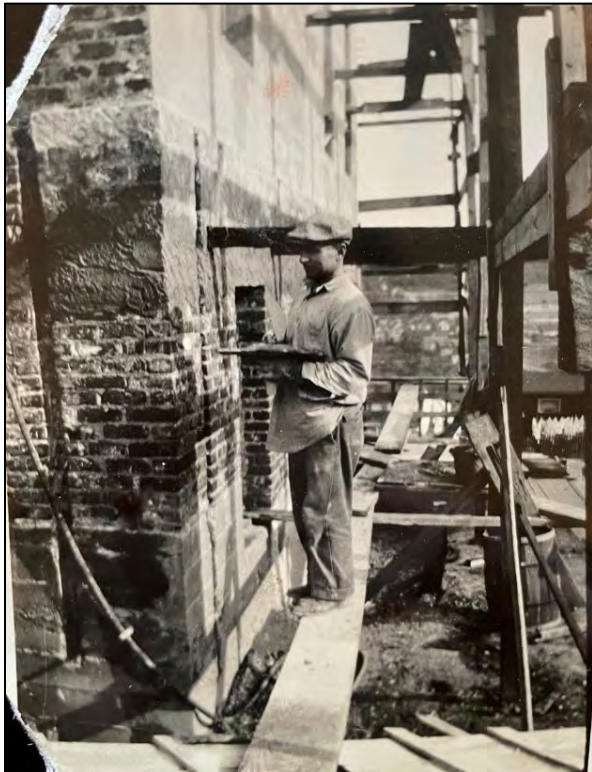
Fig. 71 - (Four photos) Ca. late 1920s-early 1930s masonry construction, showing Fausto on his home-made scaffolding with several of his children. Fausto received a building permit in 1928, but may have begun work at the site as early as 1926. We know the stuccoing was complete by 1937. Note the continuous concrete lintel serving as header for windows and doors. (VC)
