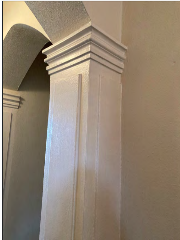
Fig. 30 – Interior, first floor corridor, detail of pilaster.
