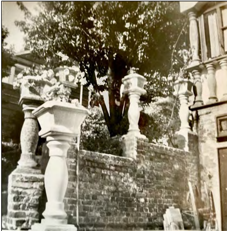
Fig. 96 - 1965 photo of the concrete column planters and brick retaining wall at the southeast corner of the house. (Intact) (VC)
