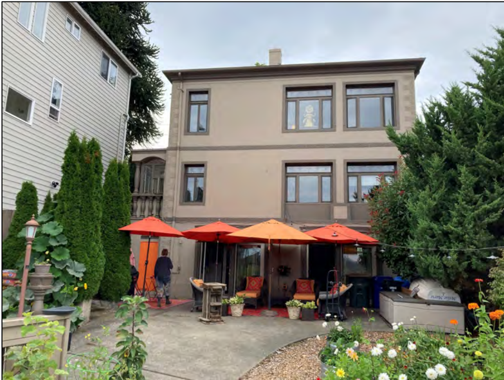
Fig. 23 – East or rear facade.
