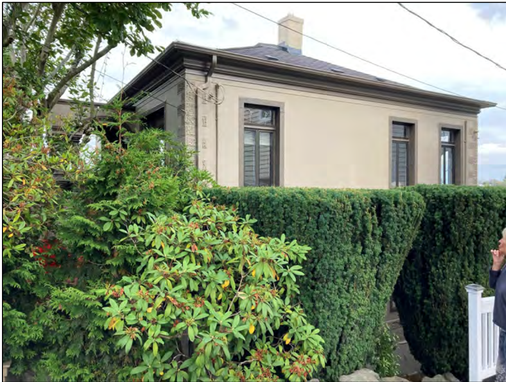
Fig. 14 – South facade (partial view)
