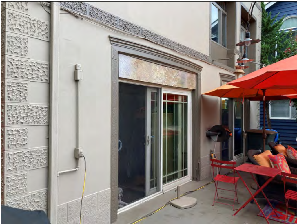
Fig. 24 – East facade, sub-basement level. The openings originally featured wooden garage doors.
