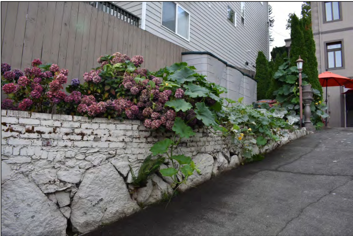
Fig. 20 – Rear yard, showing driveway retaining wall.
