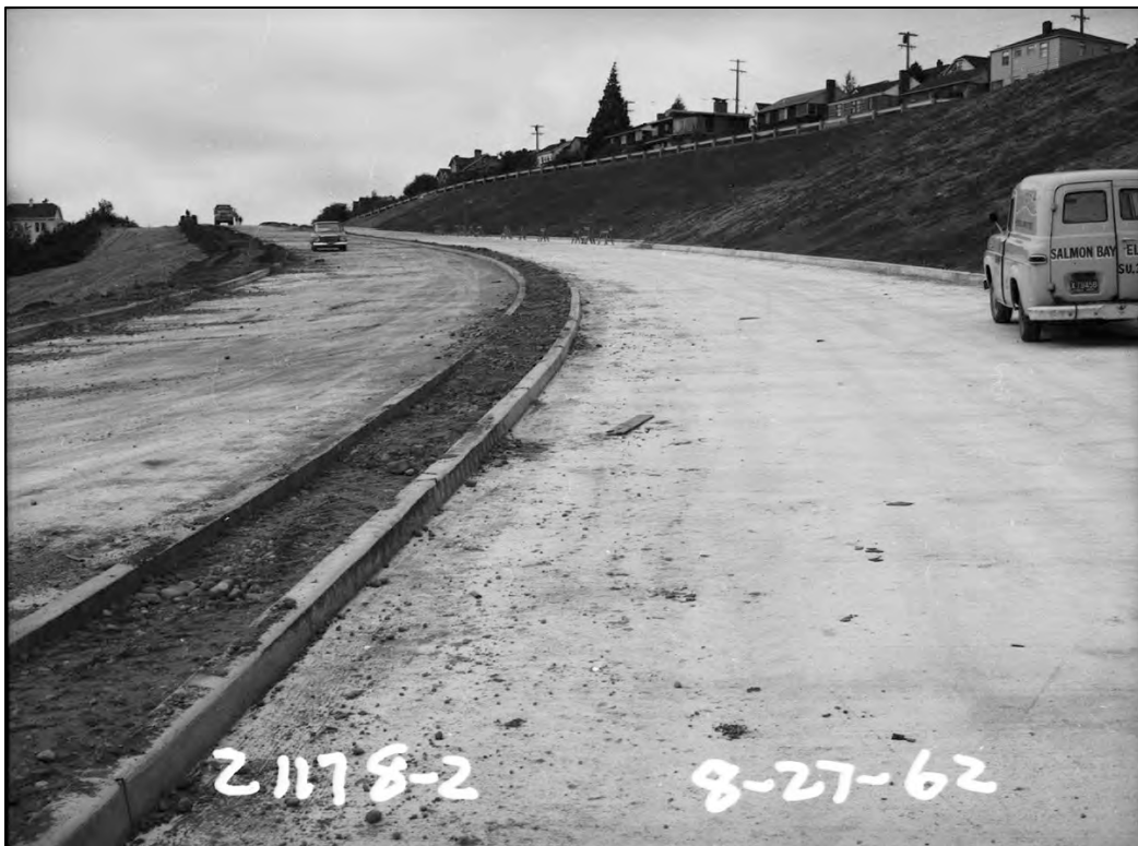
Fig. 60 – 1962 view of the newly widened and regraded Fauntleroy Avenue, one block uphill from the subject site. (SMA 72386)
