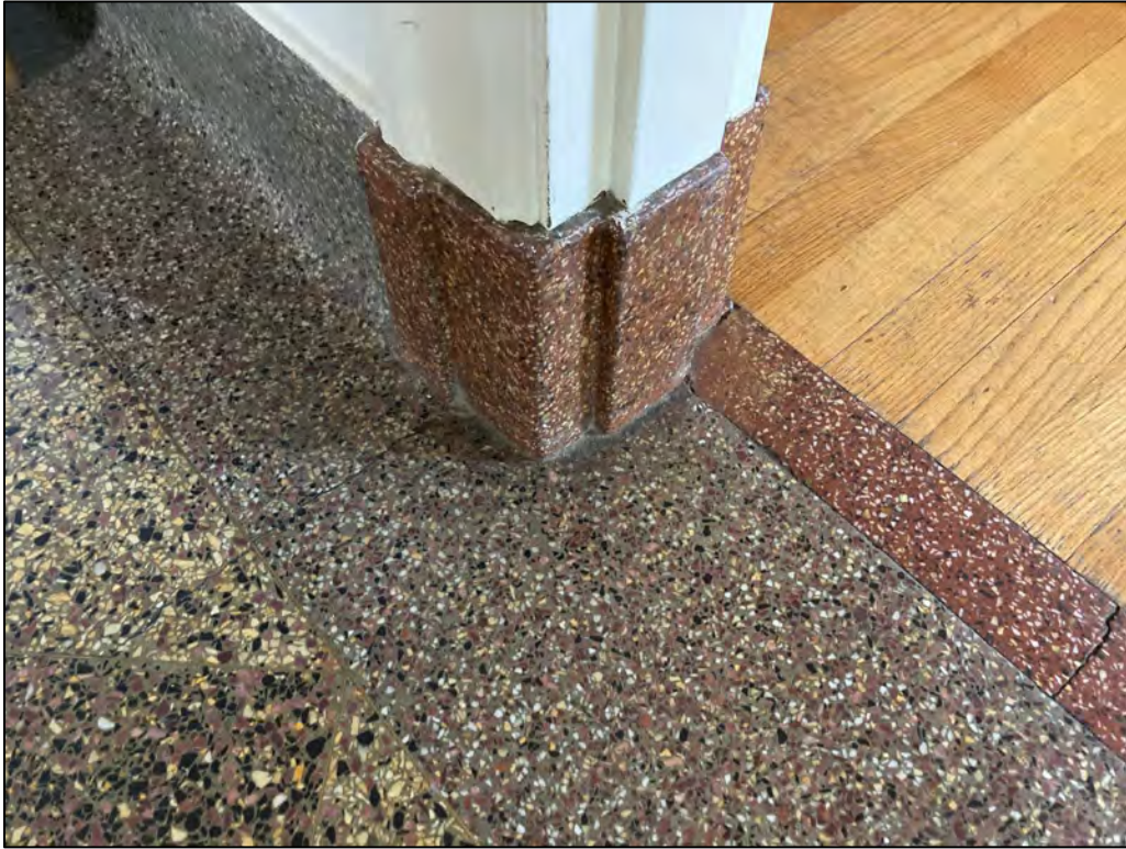
Fig. 29 – Interior, first floor corridor, detail of terrazzo and wood flooring.
