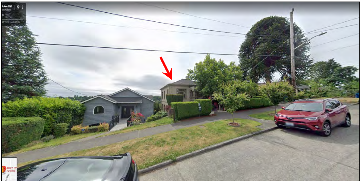
Fig. 4 – Context: View east to site across 32 nd Avenue SW. Subject house indicated by red arrow. The original property included the lots on either side of the house, which were part of the yard, and included terraced gardens. The two lots were sold in the 1990s and houses built upon them. Note large monkey puzzle tree at right, planted by Fausto Cettolin, now on adjacent property. (Google Streetview)
