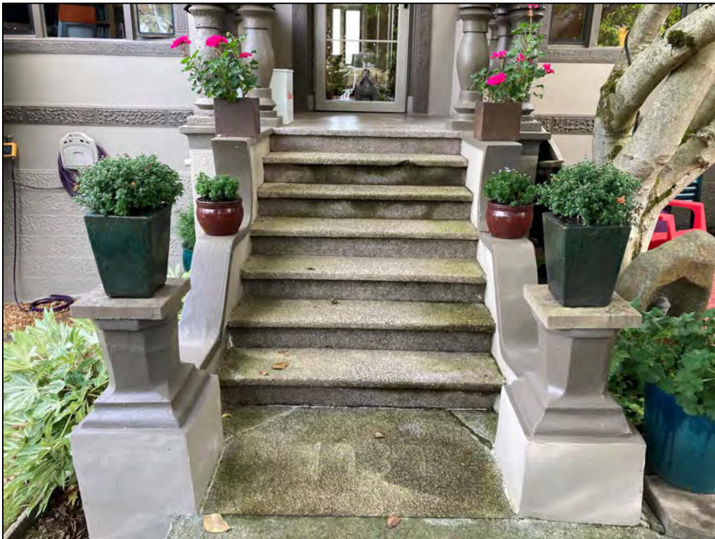
Fig. 8 – West facade, detail of front porch steps. Note “1939” at front of steps in pavement (the year the house exterior was completed), formed using metal strips and light colored aggregate.
