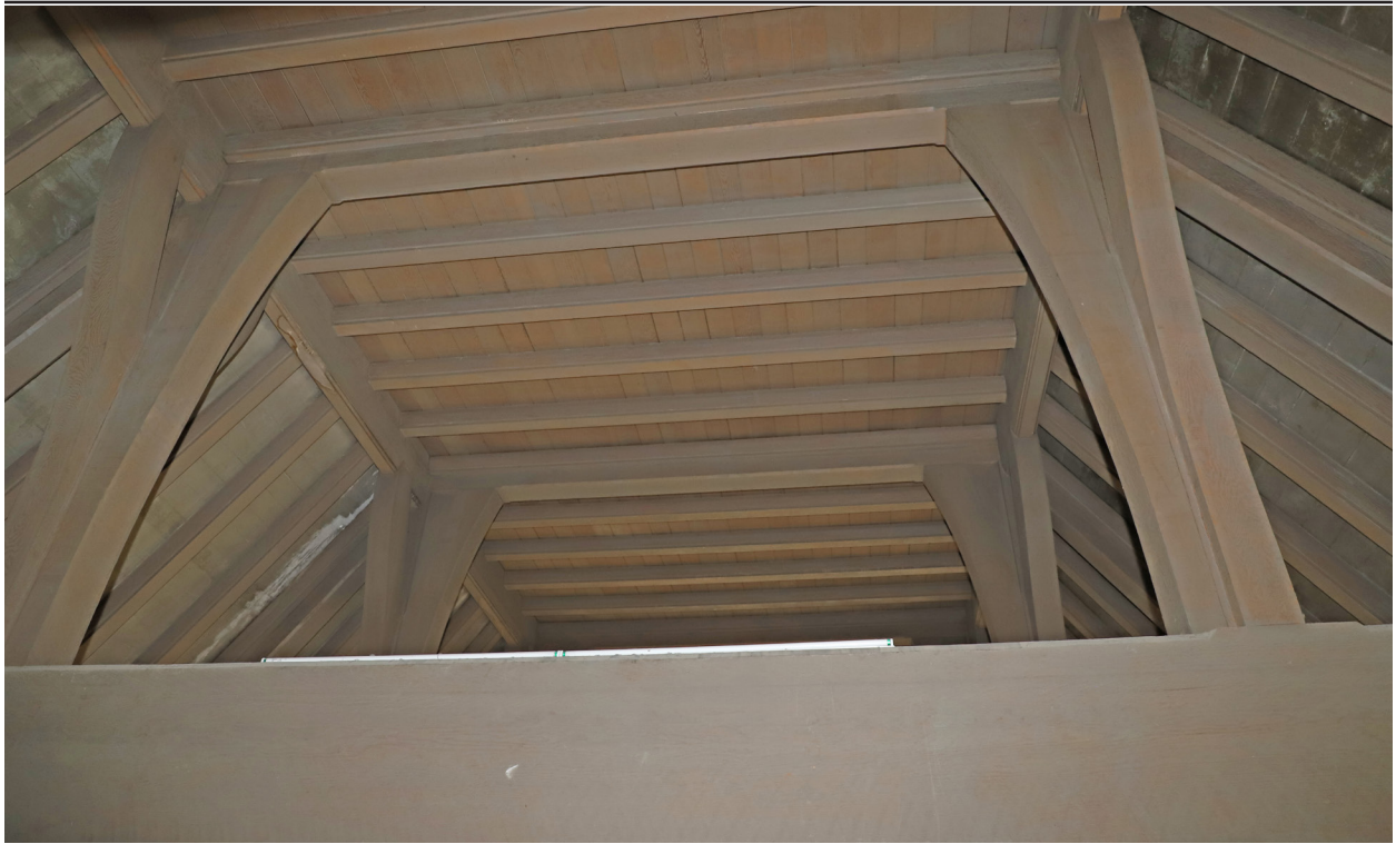
Figure 61. Reading room, roof framing.
