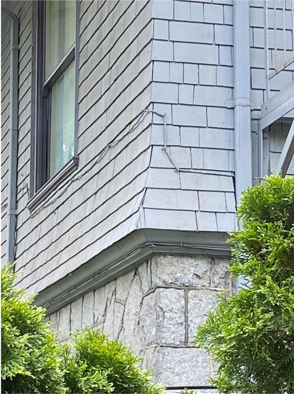
Figure 10. Stone first floor and flared shingles at second floor. (Author photo)
