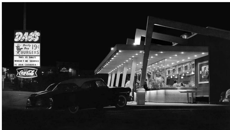
Figure 72. Left, Dag's drive-in opened at 800 Aurora Avenue N in 1955, in a highly glazed Modern style building with signage and lighting to draw customers in cars. (Both photos, Dorpat, 2018)
