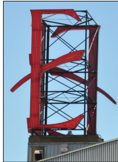
Figure 46. Above left, the original 1952 Wonder Bread sign was an example of a rooftop scaffold type. This photo shows the sign after it was salvaged, rebuilt, and installed above a new building (Kewshaw, March 28, 2006).
