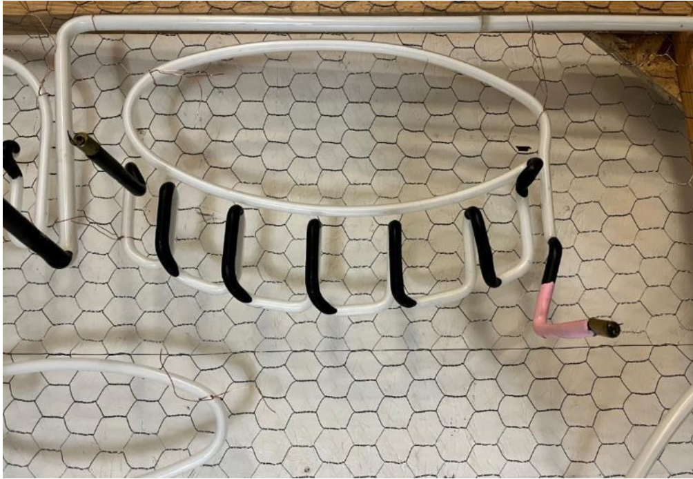
Figure 9. Above, detail view of the neon tube for elephant's pillbox hat on a temporary support.
