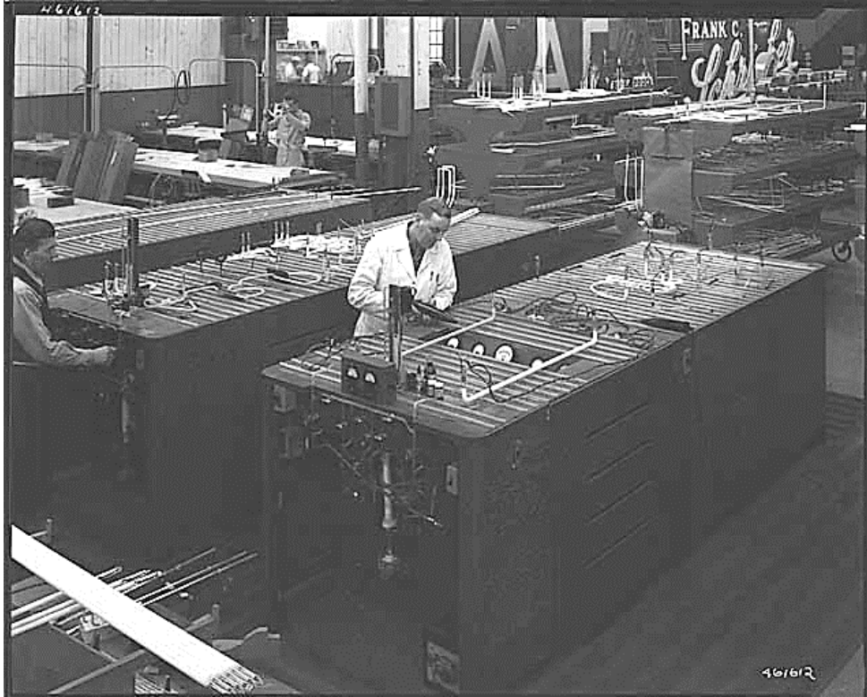
Figures 30 & 31. Below, two views of an unnamed neon sign workshop in 1947 (Webster & Stevens photos, MOHAI 1983.10.166191 & 1983.166191.5
