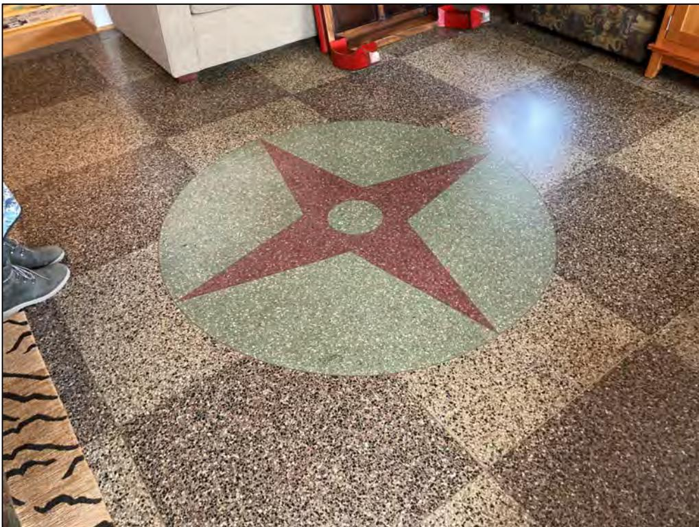
Fig. 48 – Interior, basement level, showing present living room at northeast building corner, and original terrazzo floors. The Cettolins used this room as the dining room.
