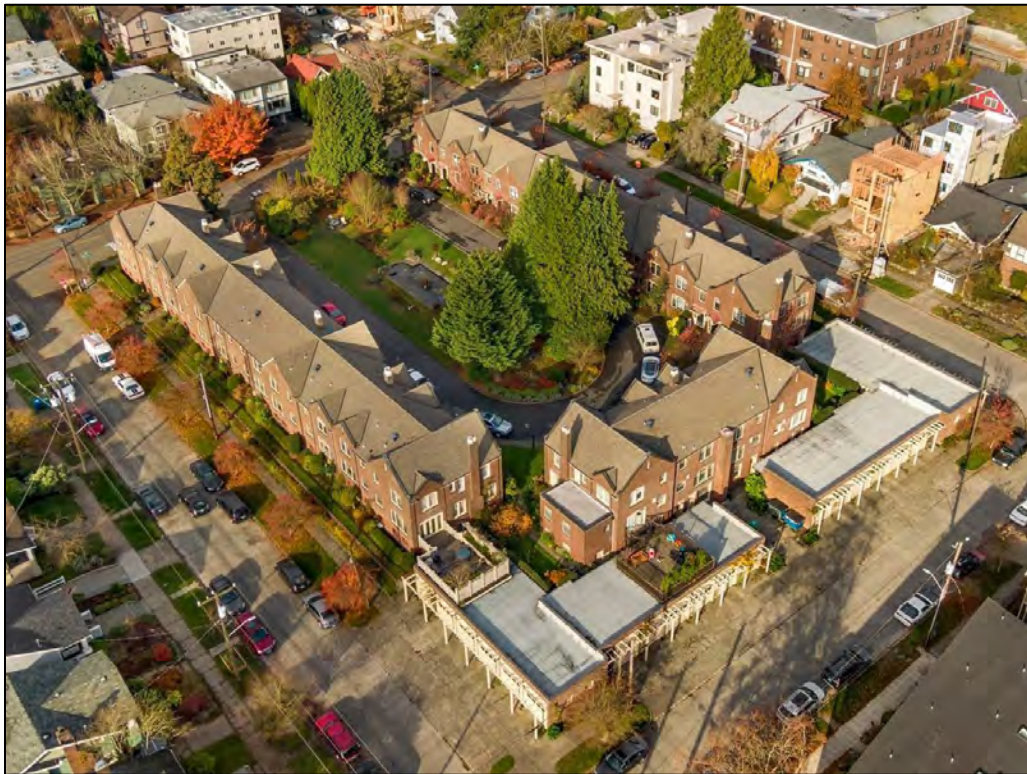
Fig. 74 – Lawton & Moldenhour: Hawthorn Square (1923). (NW Multiple Listing Service)
