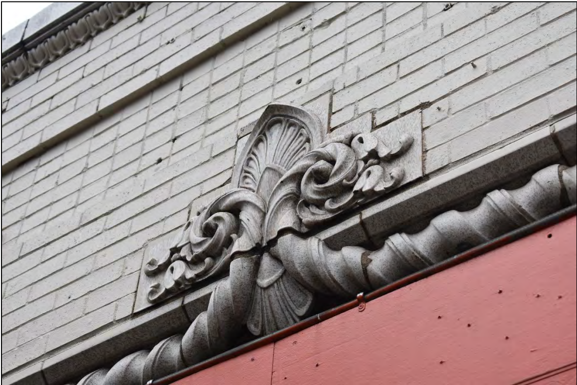
Fig. 43 - East facade, detail of glazed terra cotta ornament above storefront.
