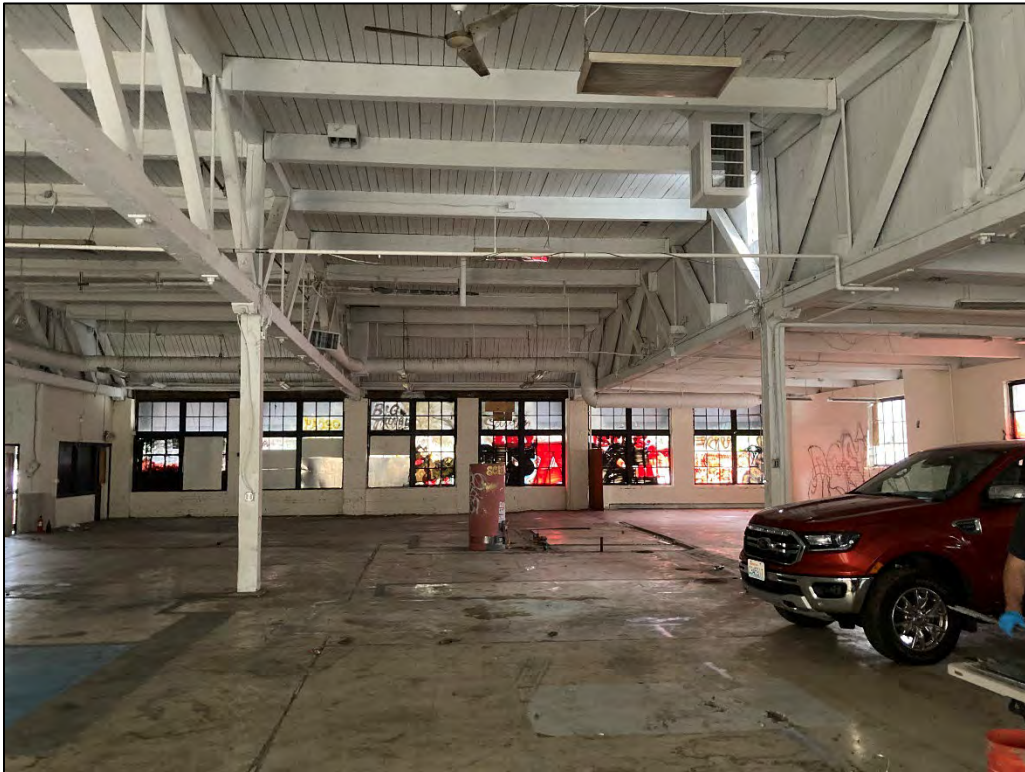
Fig. 55 – Garage interior, view west.
