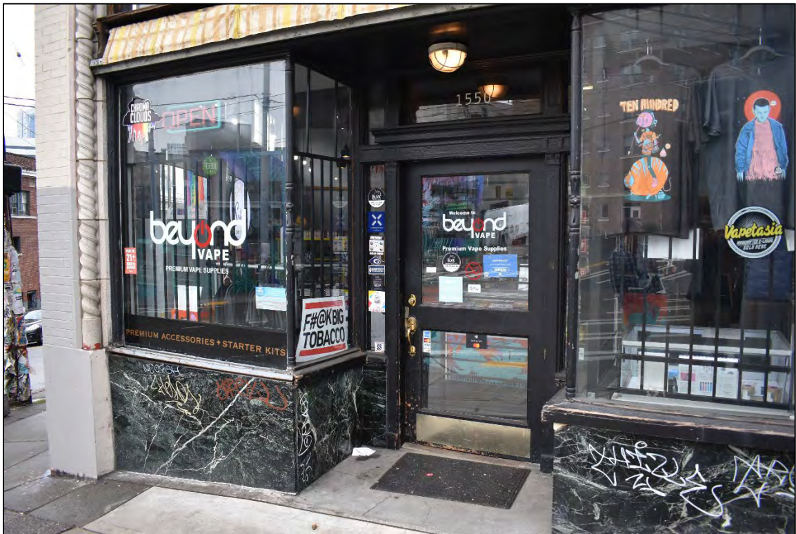
Fig. 21 – East facade, first bay, detail of lower part.
