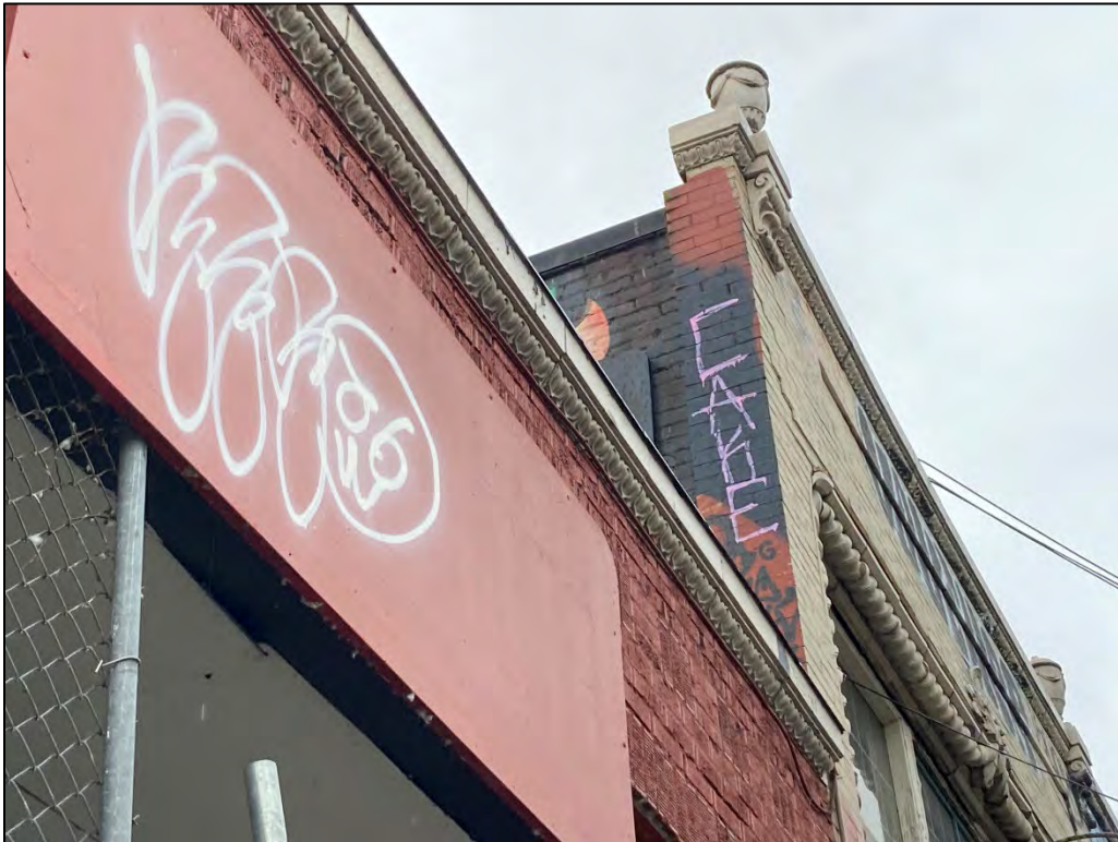
Fig. 13 – South facade, detail of parapet trim at garage and retail components.
