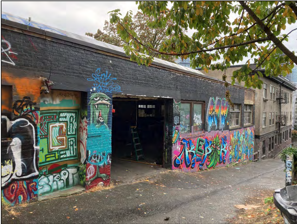
Fig. 50 – North facade, west part.
