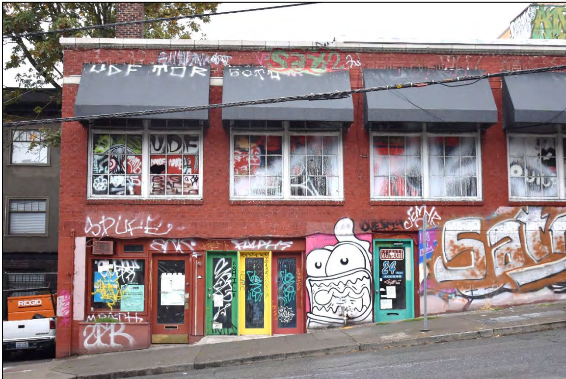
Fig. 8 - South facade, west part.
