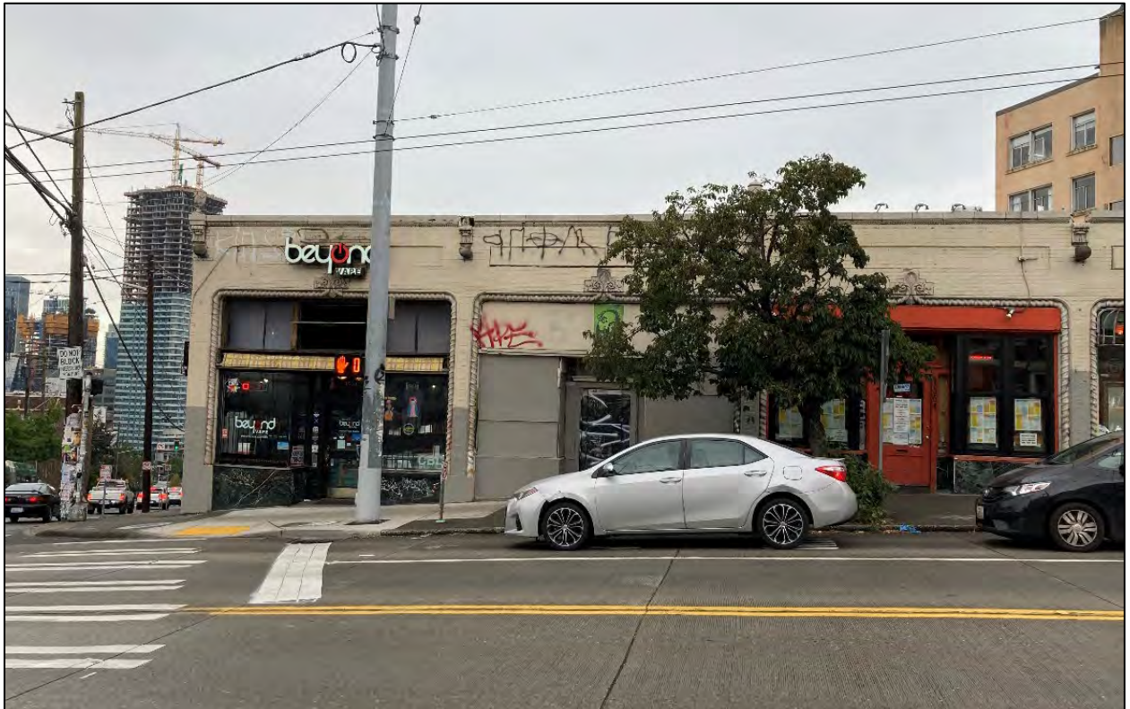
Fig. 16 - East facade, south part.
