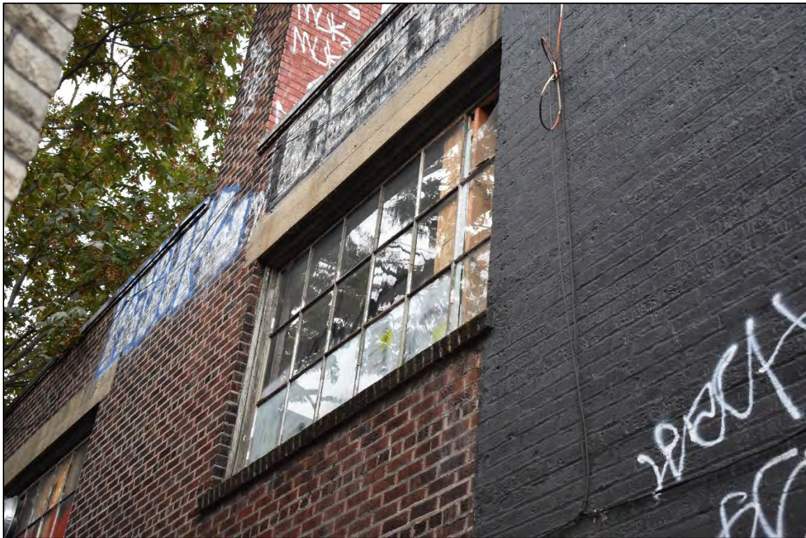
Fig. 52 – West facade, detail of window and masonry.
