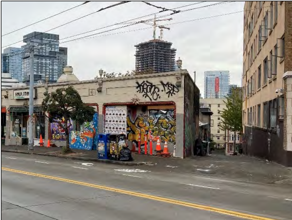
Fig. 19 – Northeast building corner, showing alley.
