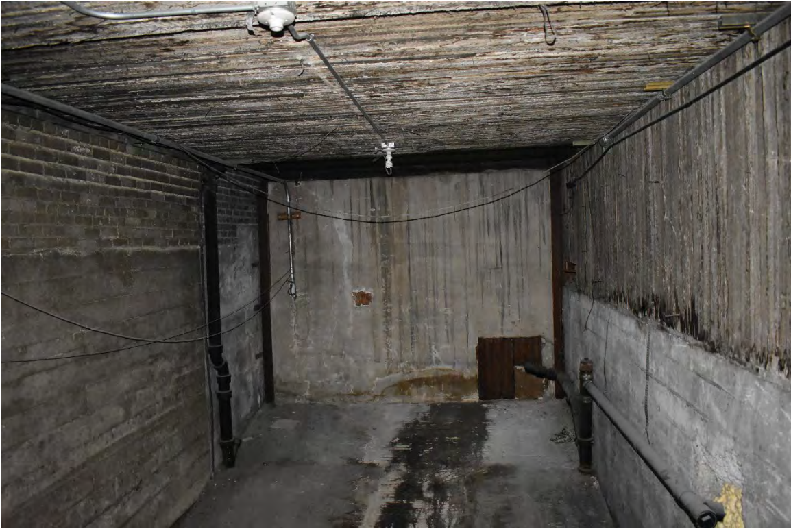
Fig. 41 - East facade, sixth bay, interior (a former garage entry).
