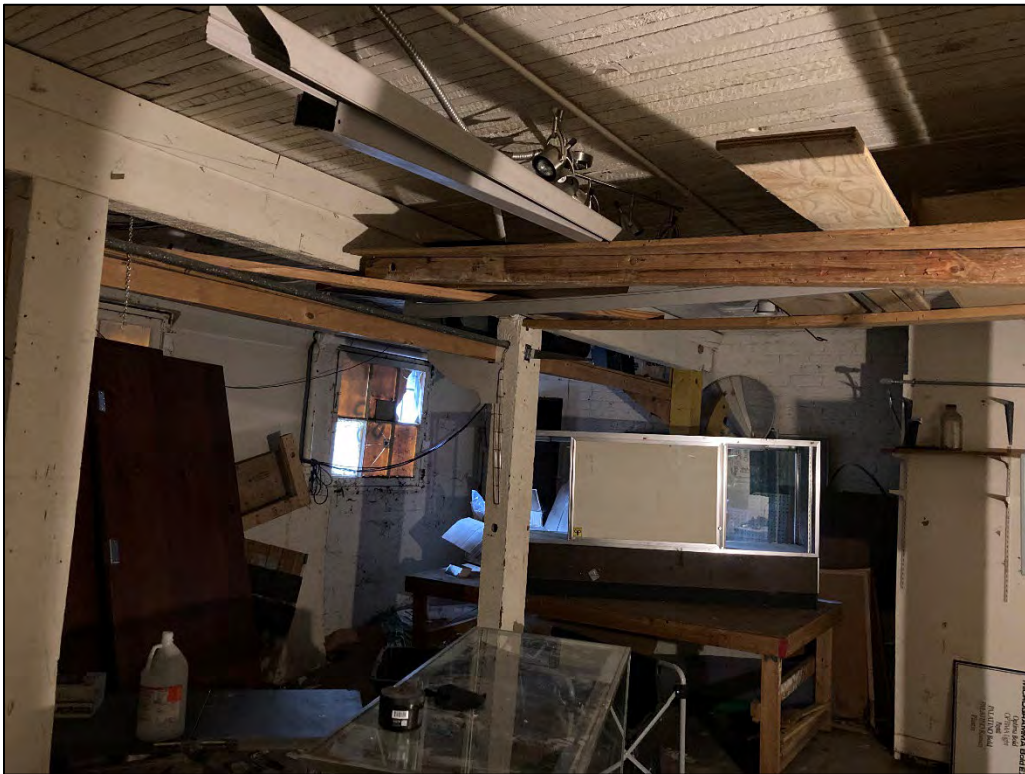
Fig. 58 - Garage basement, interior, showing westernmost retail space accessed from E Denny Way.
