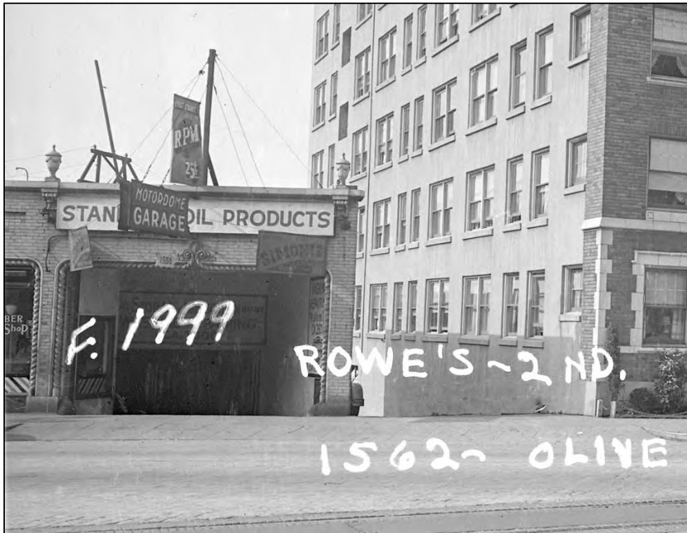
Fig. 62 - 1937 tax assessor photo detail of adjacent property, showing sixth bay of east facade of the subject building, when it was a garage entry from E Olive Way. (KCTA)
