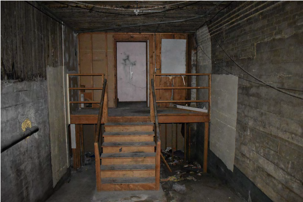
Fig. 42 - East facade, sixth bay, interior (a former garage entry). Wood frame wall visible is the back of the store that was built in the former ramp space.
