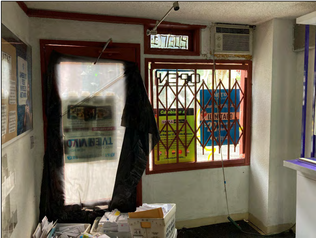
Fig. 57 - Garage basement, interior, showing westernmost retail space accessed from E Denny Way.
