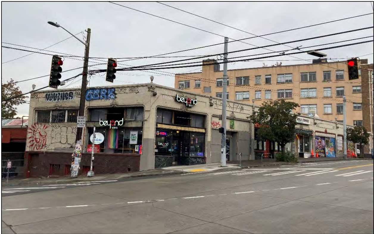
Fig. 14 – Southeast building corner, showing retail component.
