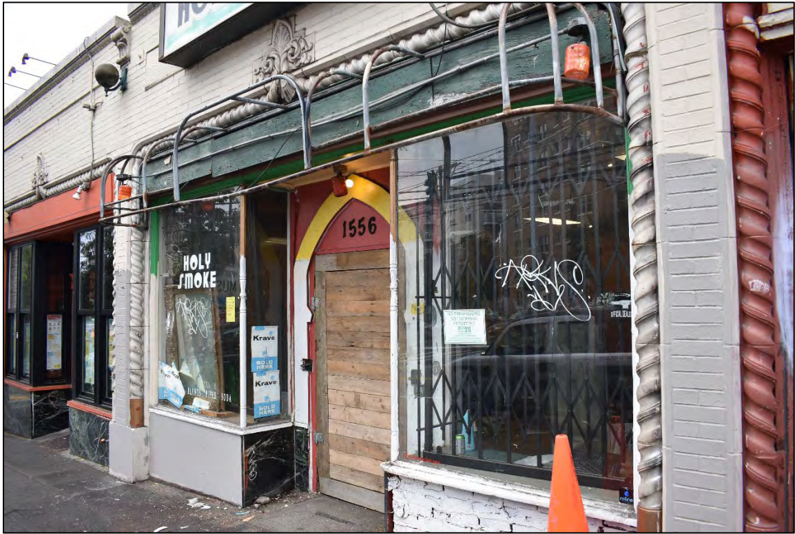
Fig. 33 – East facade, fourth bay.
