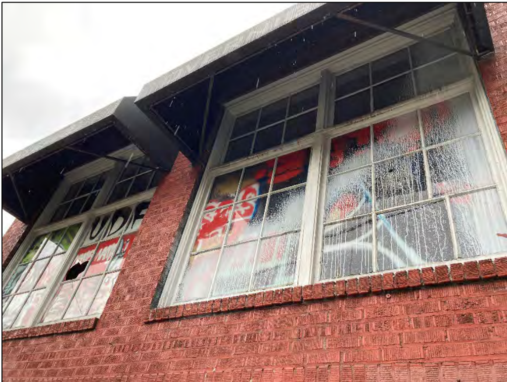
Fig. 10 – South facade, detail of windows.
