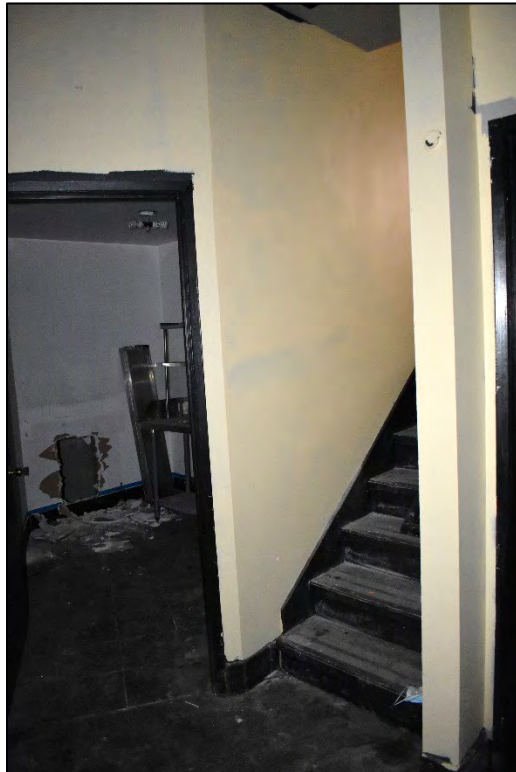
Fig. 37 – East facade, fifth bay, interior, showing stairs to mezzanine.
