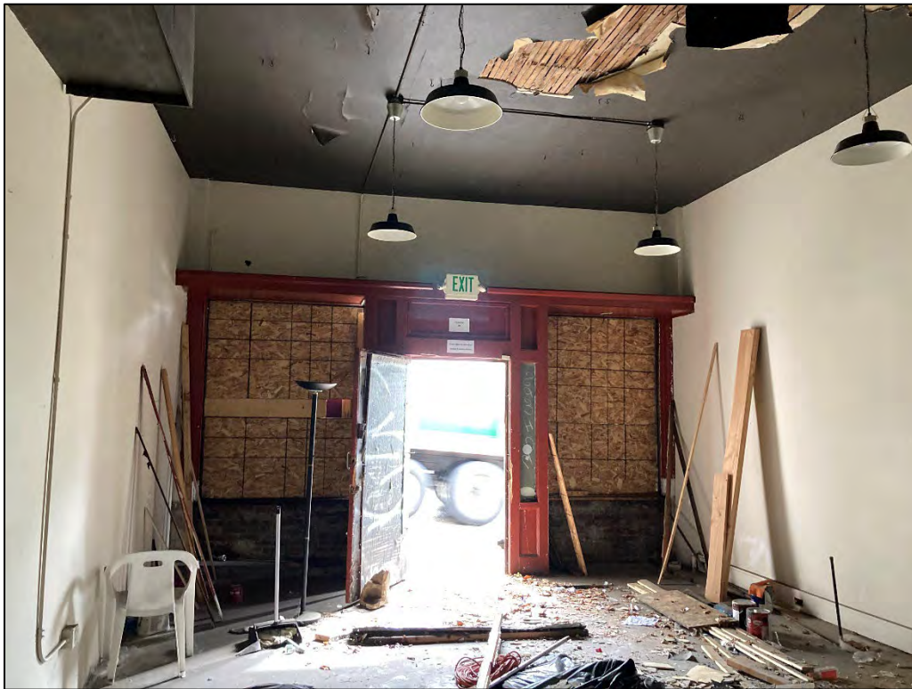
Fig. 28 – East facade, second bay, interior.
