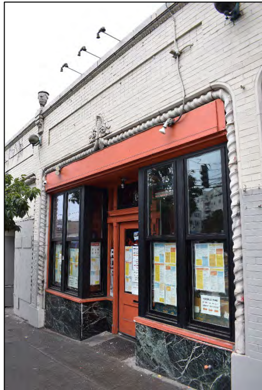
Fig. 30 – East facade, third bay.
