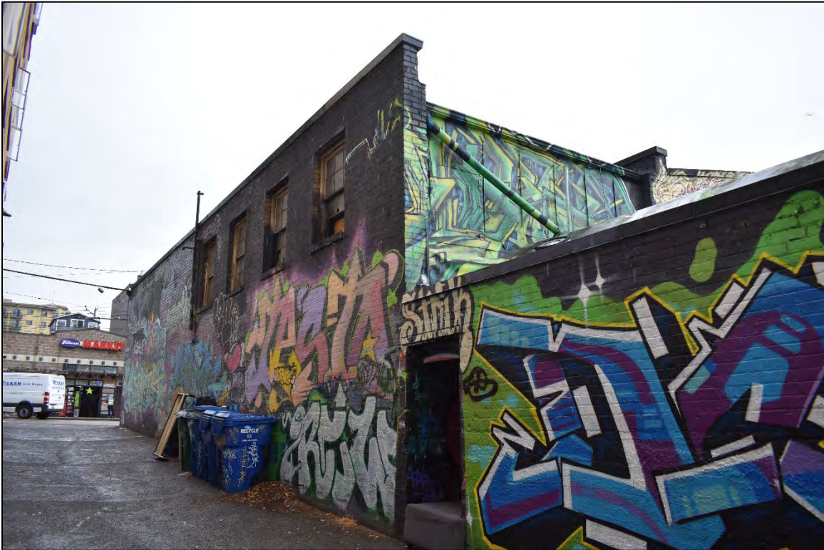
Fig. 48 – North facade, east part. Windows visible at left light the mezzanine of the fifth storefront.
