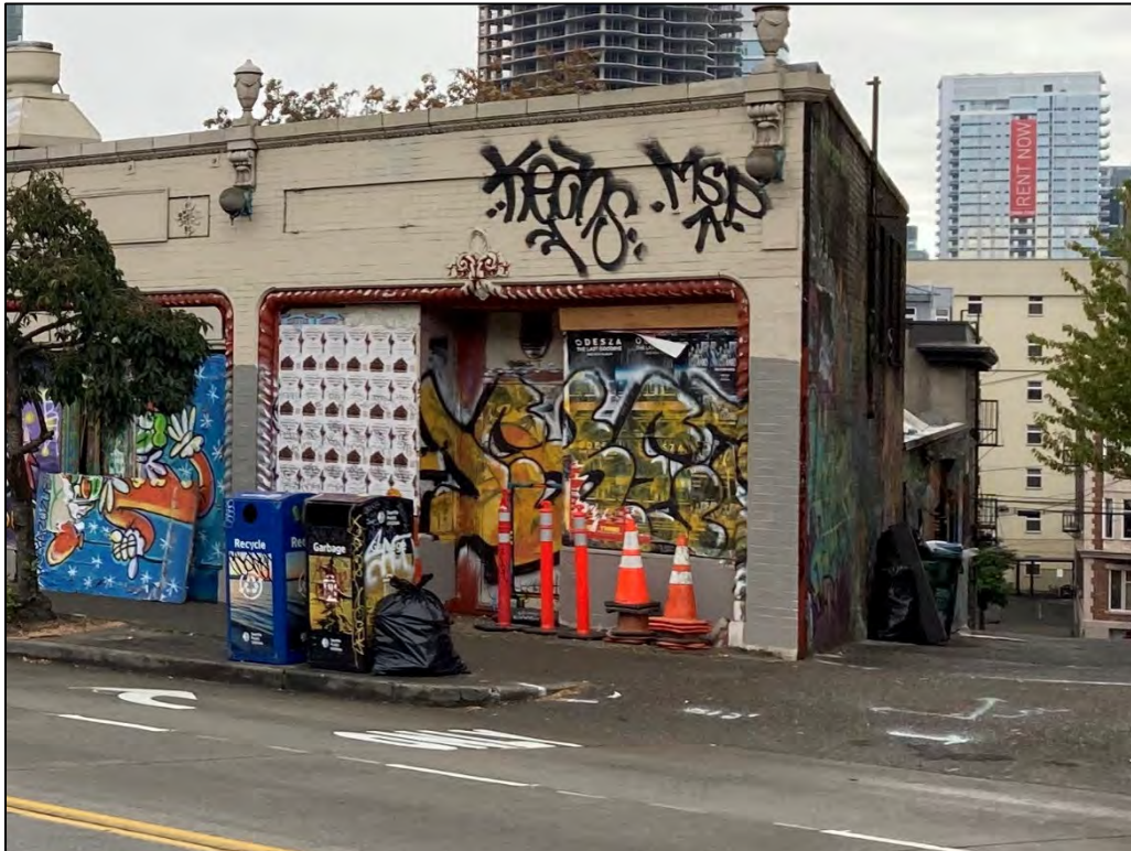
Fig. 39 – East facade, sixth bay.
