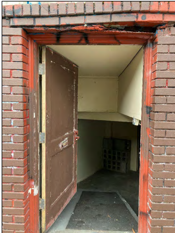
Fig. 59 – Garage basement, interior, showing easternmost retail space accessed from E Denny Way.
