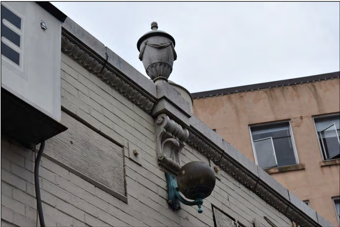
Fig. 44 - East facade, detail of glazed terra cotta bracket, painted brick wall, parapet urn, and light fixture.
