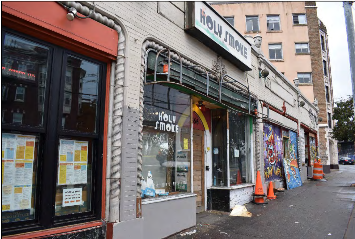
Fig. 18 – East facade, view north along sidewalk.
