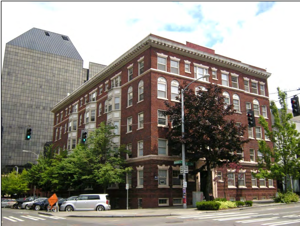
Fig. 71 – Lawton & Moldenhour: Castle Apartments (1918). The building is a designated Seattle landmark. (Joe Mabel)
