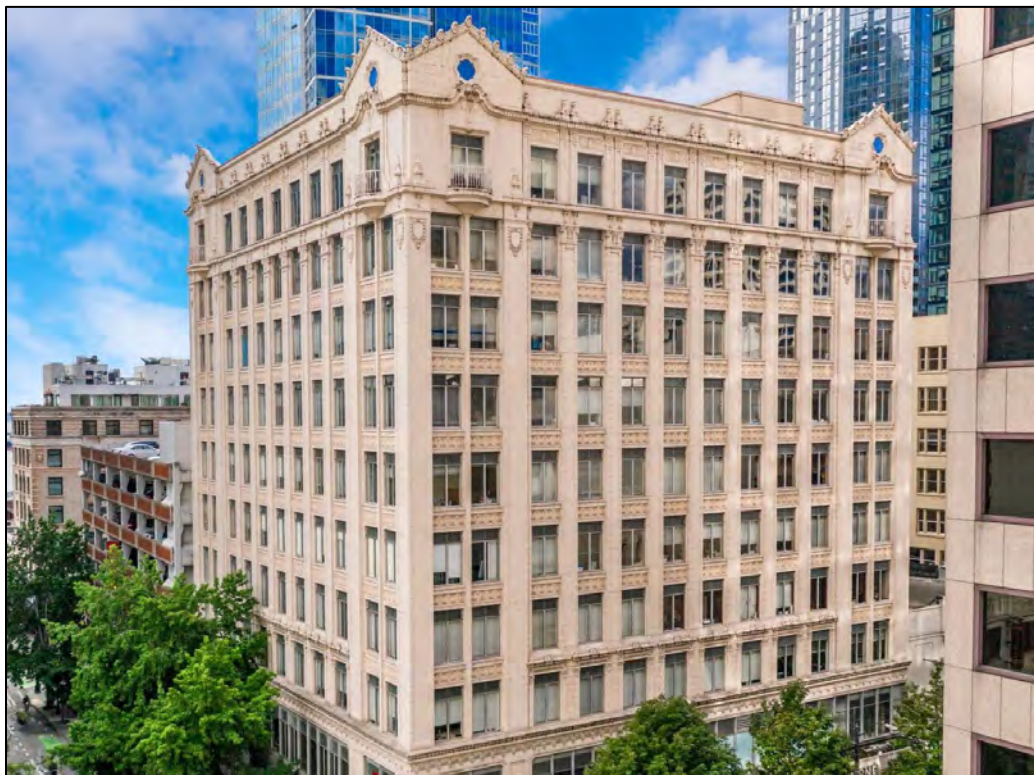
Fig. 80 – Lawton & Moldenhour: Republic Building (1927, now the Melbourne Tower). (MelbourneTower.com)
