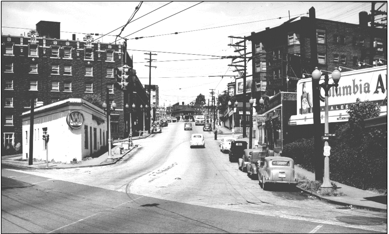
Fig. 63 – 1945 view north on E Olive Way at Bellevue Avenue, after the former was cut through in 1923. Subject building hidden but located in distance, at left. (SMA 54404)
