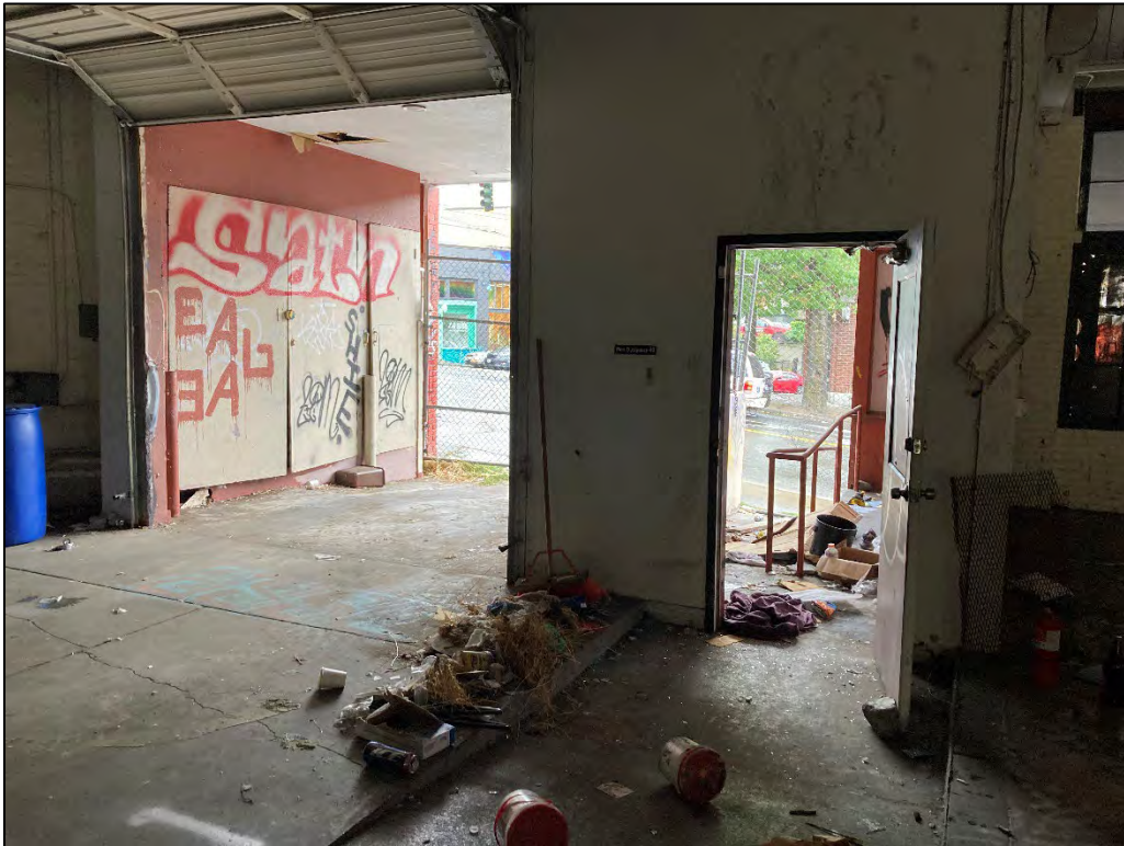
Fig. 53 – Garage interior, view south showing access to E Denny Way.
