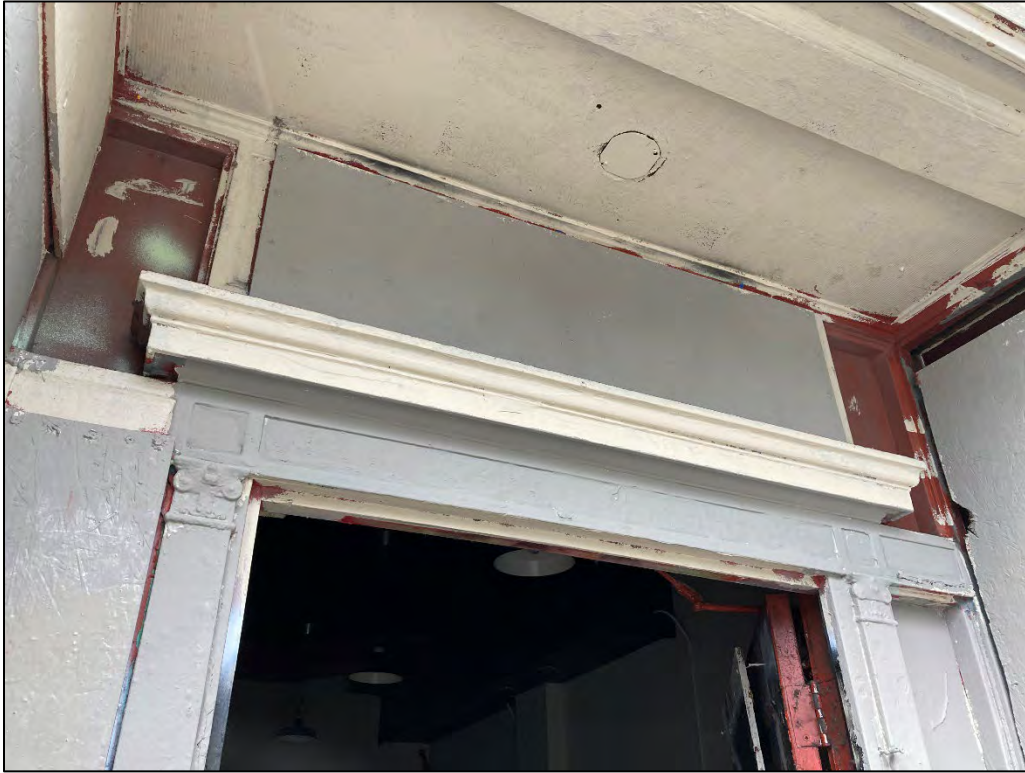
Fig. 45 - East facade, detail of storefront entry trim.
