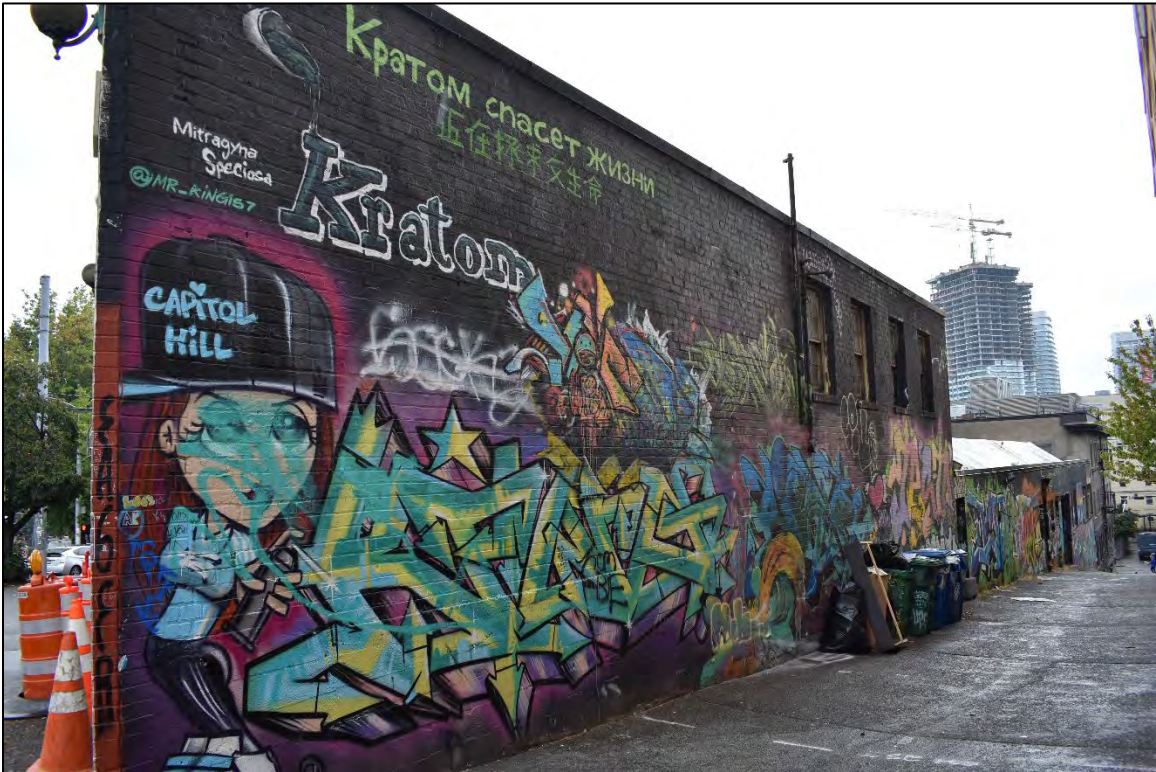
Fig. 47 – North facade, view west along alley.
