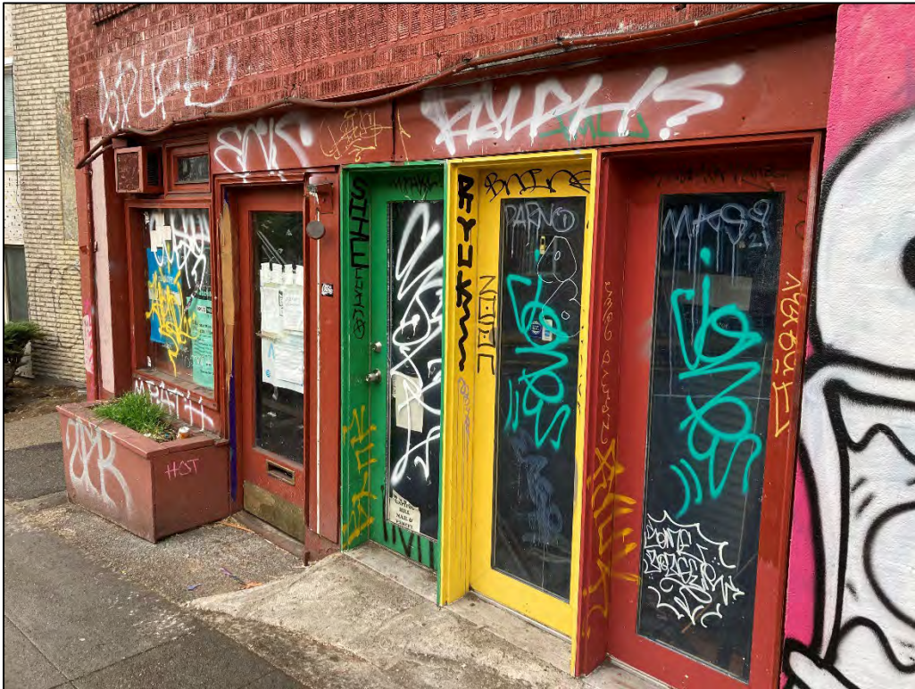
Fig. 11 – South facade, detail of basement level storefront.
