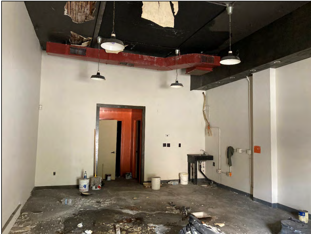
Fig. 29 – East facade, second bay, interior.
