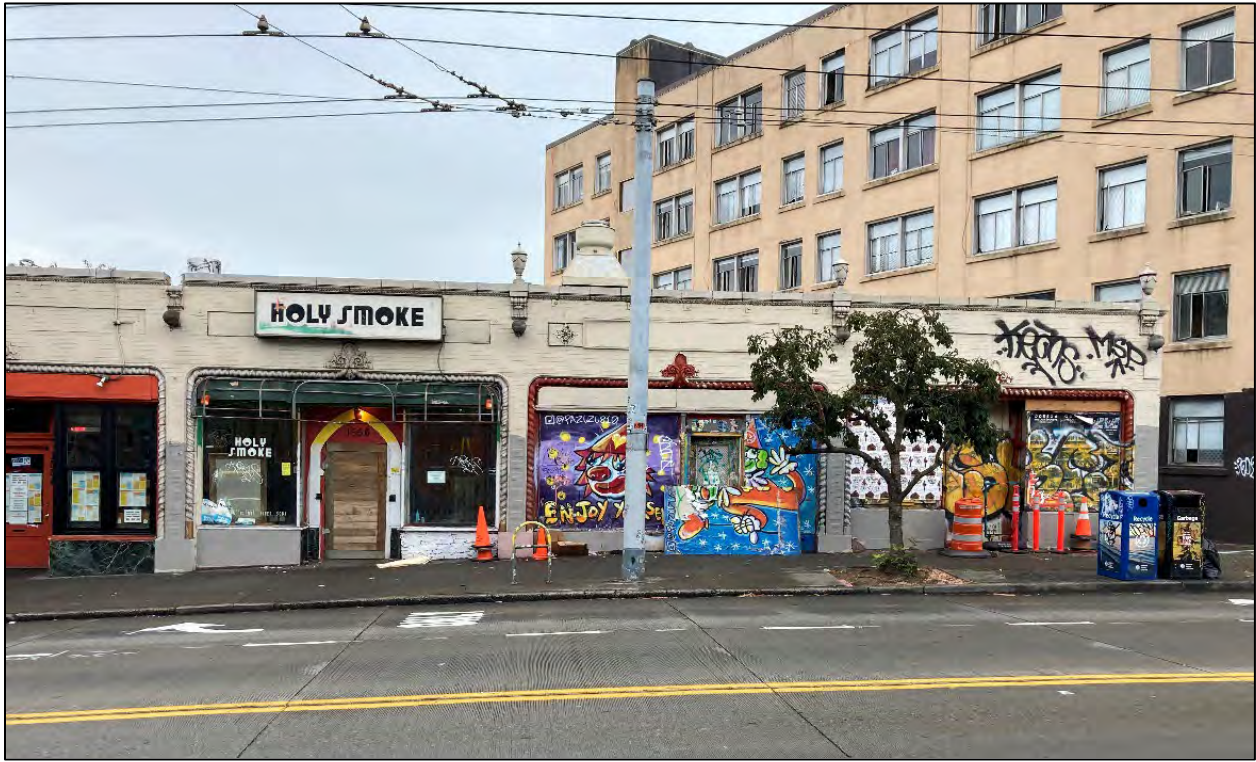
Fig. 17 – East facade, north part.
