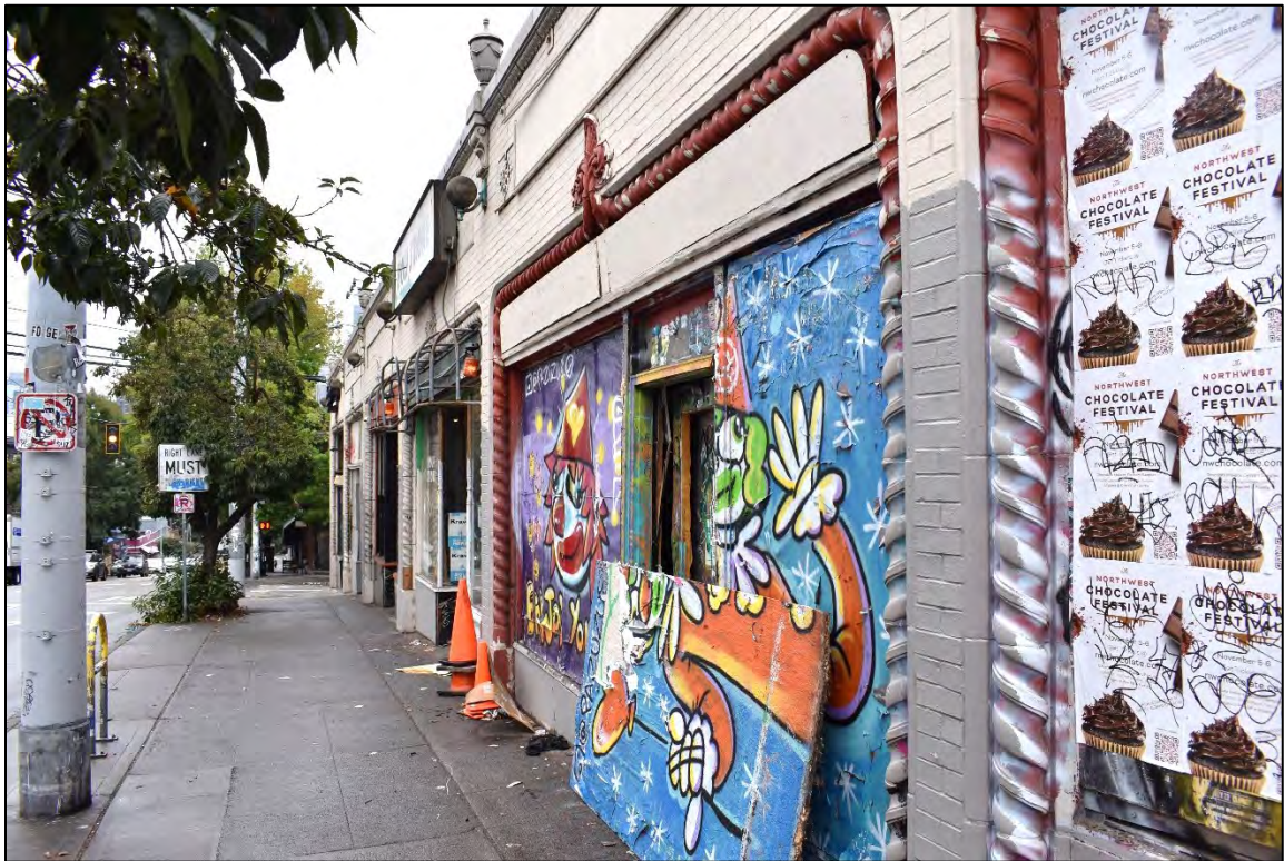
Fig. 34 – East facade, fifth bay.
