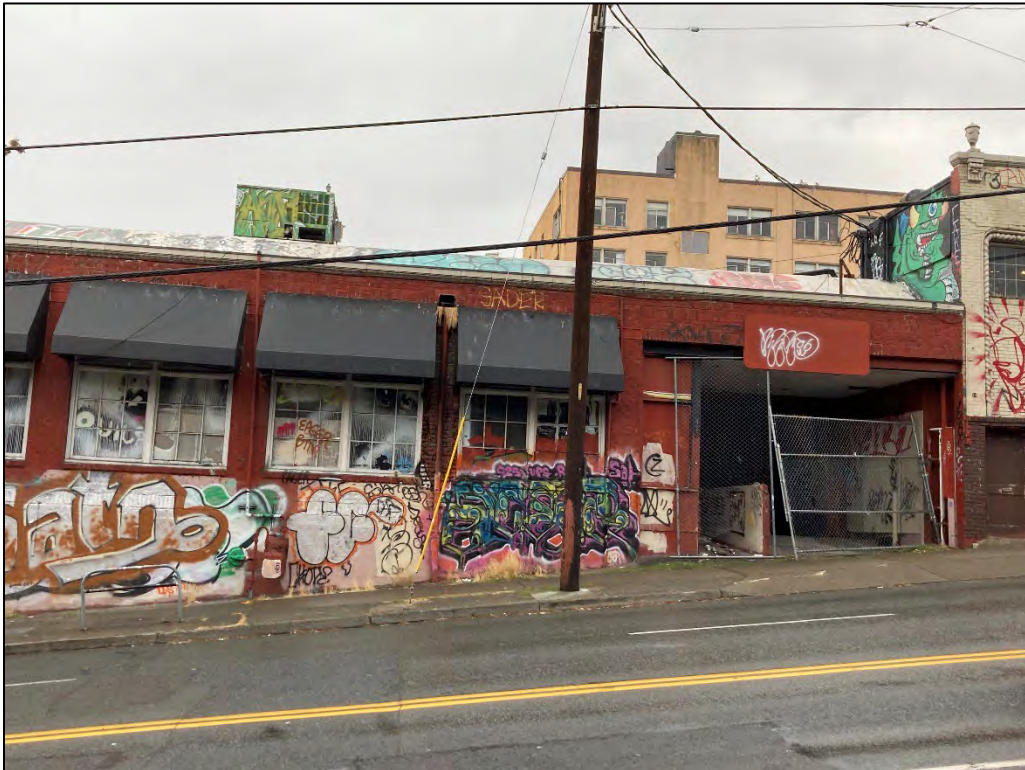
Fig. 9 – South facade, center part.
