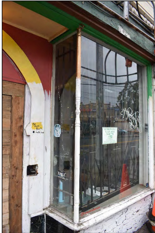
Fig. 46 - East facade, detail of storefront window with turned wood corner post.
