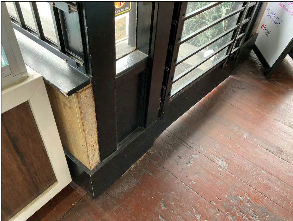
Fig. 26 – East facade, first bay, interior.
