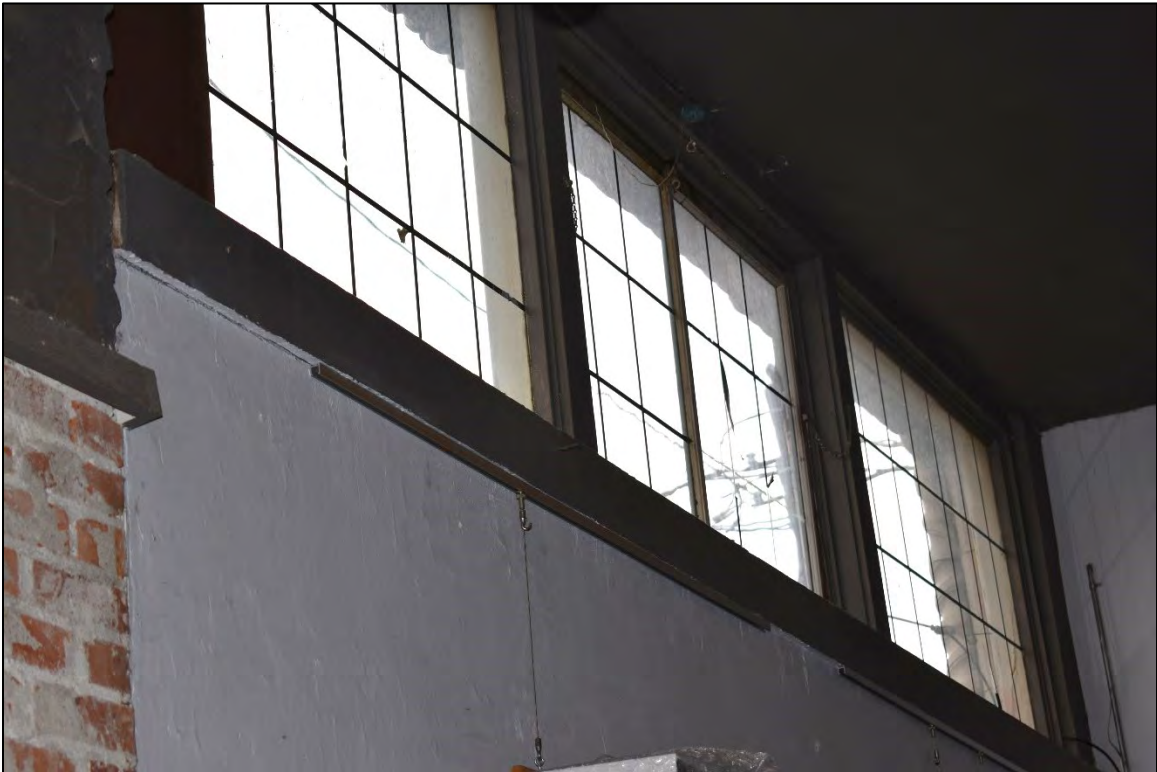
Fig. 25 – East facade, first bay, interior.
