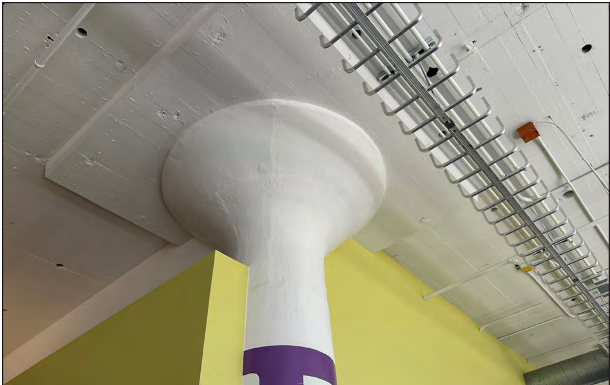
Figure 30 • Interior of former American Can Co., detail of 1925 column capital, 2nd floor
