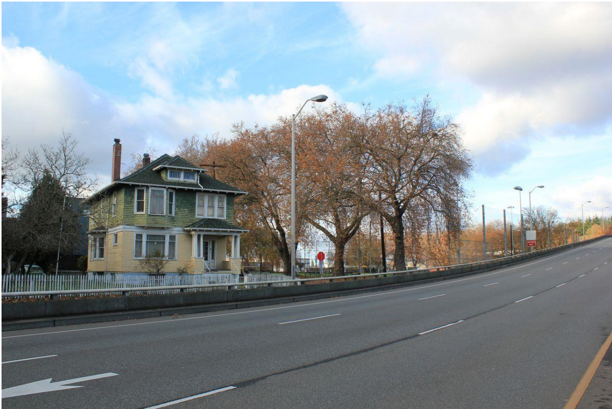
B2. Woodin House, view N from Corson Ave S exit ramp
