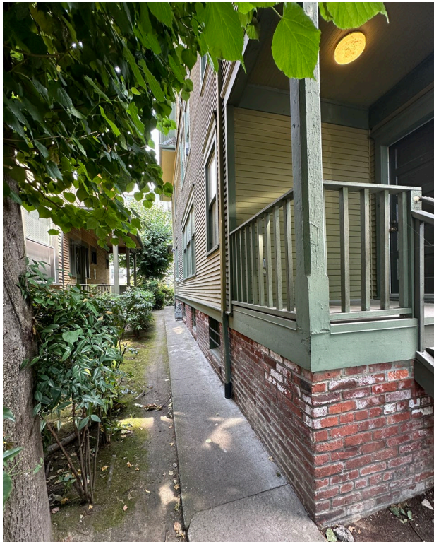
Fig.15: (left) Walkway along north side of building (looking east) showing masonry brick foundation and Fig. 16: (right) typical Palladian window on upper gable.
