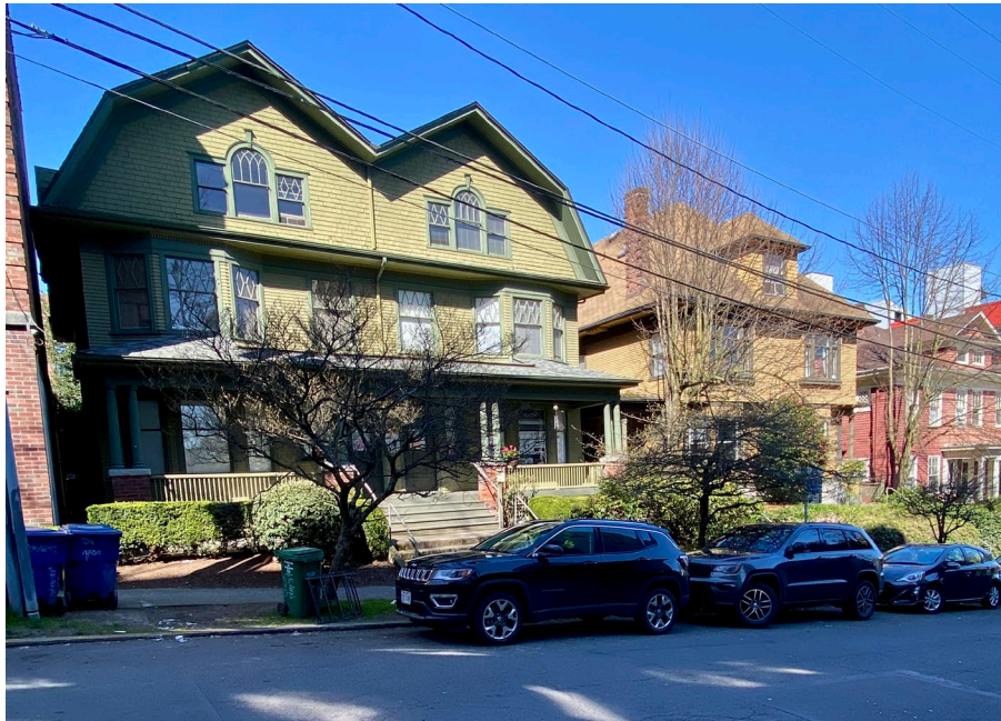
Fig. 6: Street view of Boylston Ave (Apr 2021), view west. 1411 Boylston Ave on left, with neighboring “double houses” to the right.
