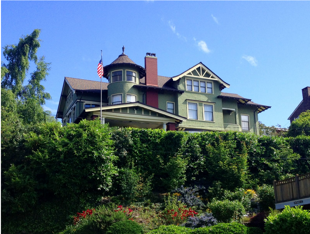
Fig 37a: Poulson House, 103 Highland Drive, Queen Anne neighborhood. by Josenhans & Allen, 1904-1906. Source: Historic Seattle
