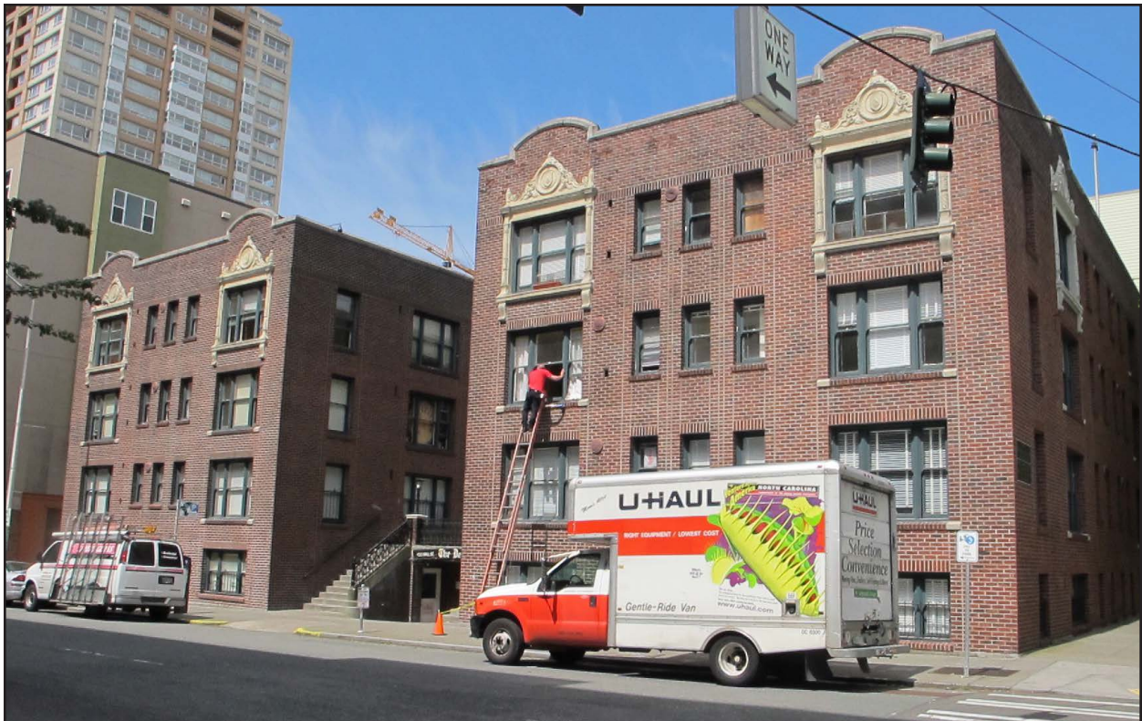
Figure 46 • Devonshire Apartments (420 Wall Street, 1925)
