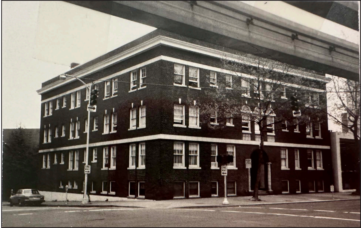
Figure 31 • King County Tax Assessor photograph, 2132 Fifth Avenue, 1986
