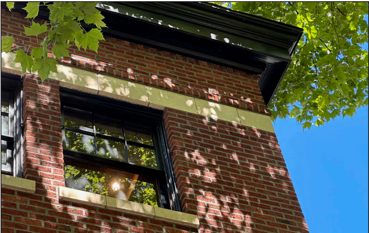
Figure 9 • 2132 Fifth Avenue, western façade, roof detail
