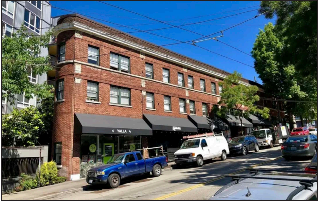
Figure 35 • Olive Crest Apartments (Lawton & Moldenhour, 1924)
