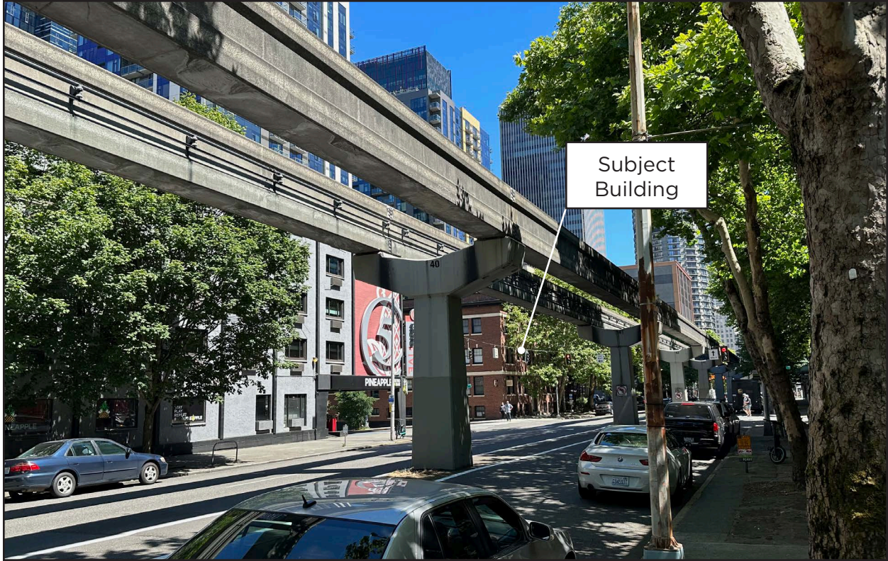
Figure 5 • View C: Viewing southeast along Fifth Avenue
