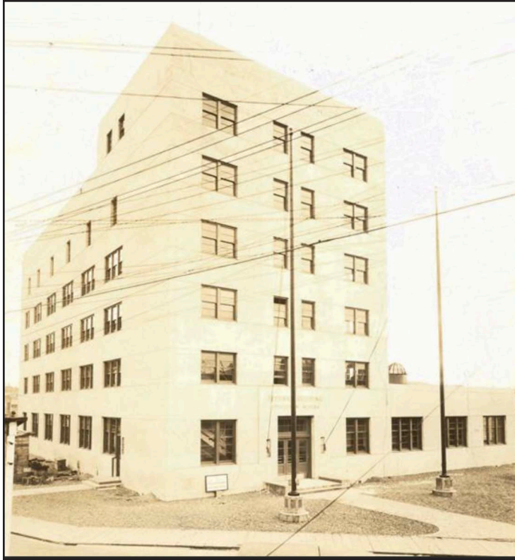
Figure 37 • Ketchikan Federal Building, Alaska 1938
