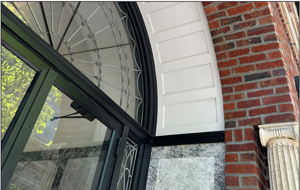
Figure 11 • 2132 Fifth Avenue, western façade, main entrance detail
