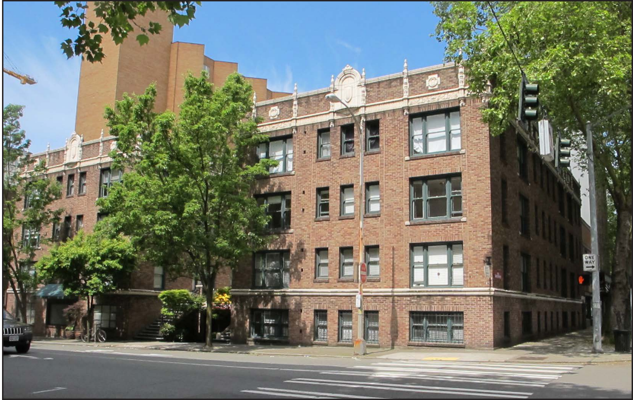
Figure 45 • Davenport Apartments (420 Vine Street, 1925)
