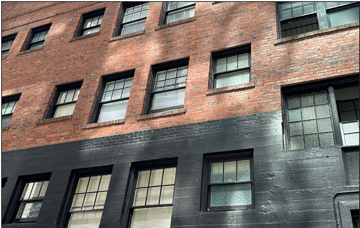
Figure 17 • 2132 Fifth Avenue, eastern façade, brick and window detail
