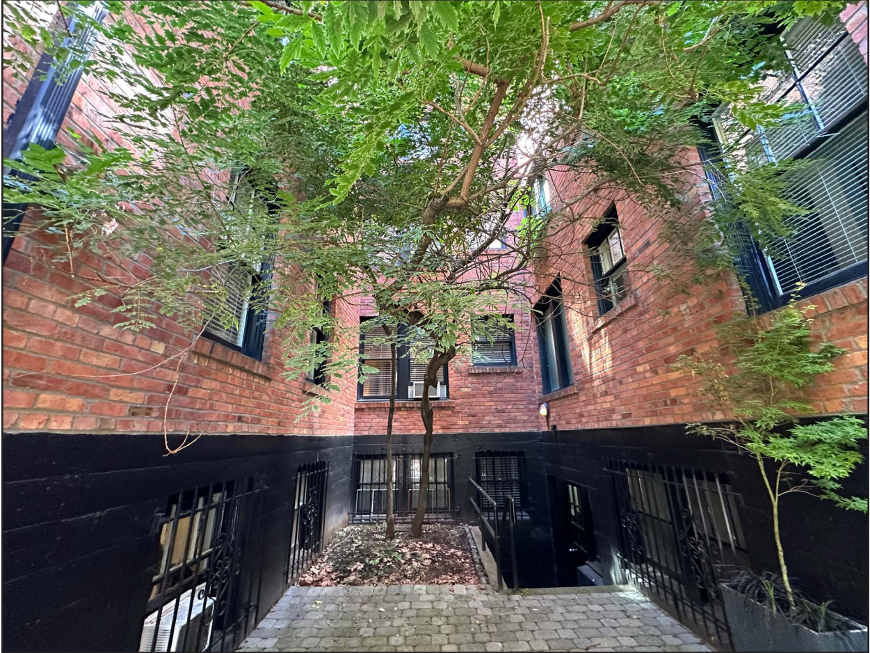
Figure 15 • 2132 Fifth Avenue, courtyard facing north
