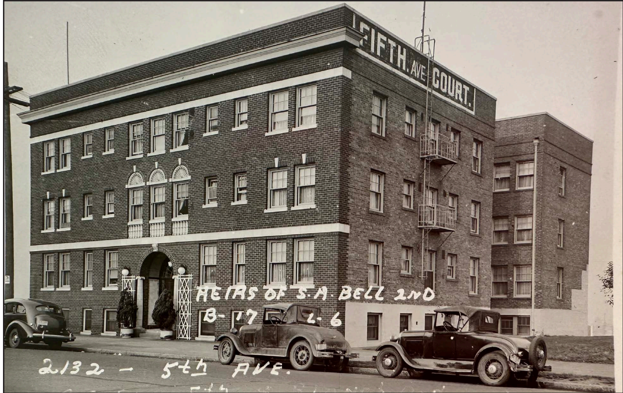
Figure 29 • King County Tax Assessor photograph, 2132 Fifth Avenue, 1937
