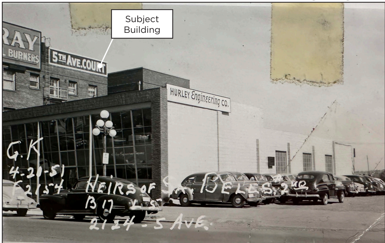
Figure 30 • King County Tax Assessor photograph, 2124 Fifth Avenue, 1951
