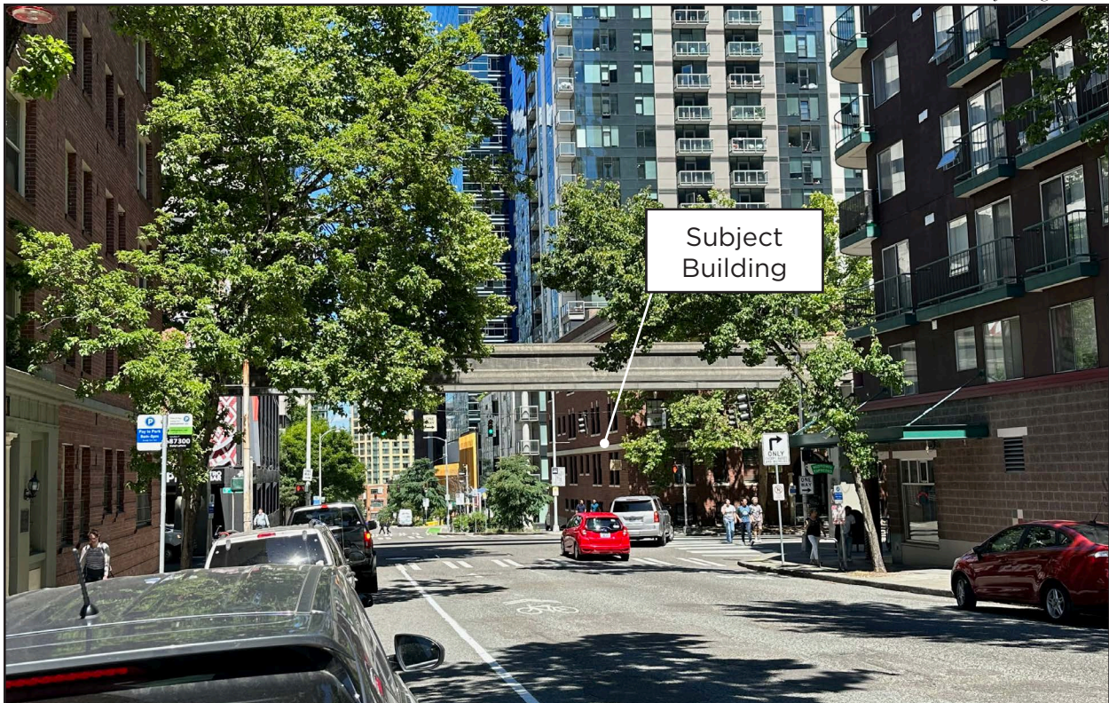
Figure 4 • View B: Viewing northeast along Blanchard Street
