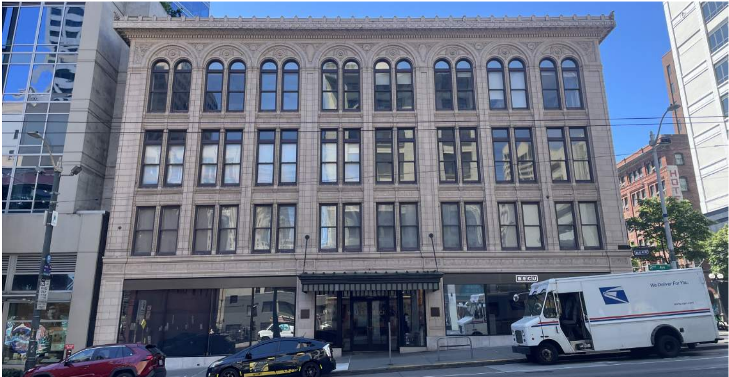
EAST (2ND AVENUE) FACADE
