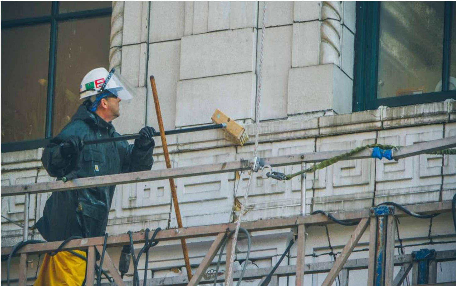
EXAMPLE OF WORKER CLEANING TERRA COTTA FACADE
