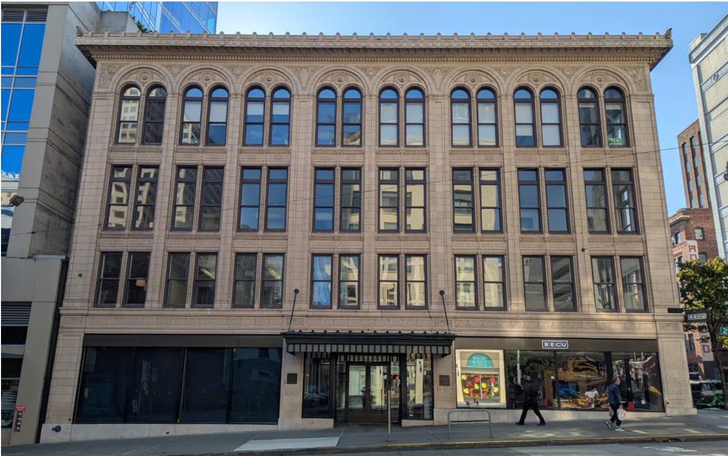
EAST (2ND AVENUE) FACADE
