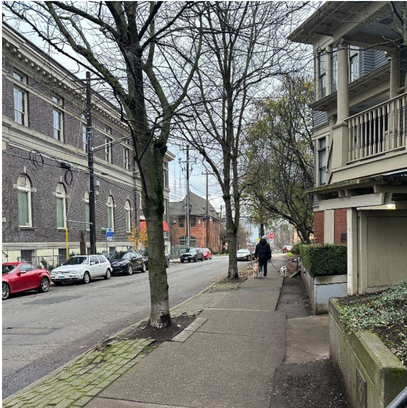
North elevation and neighborhood.
