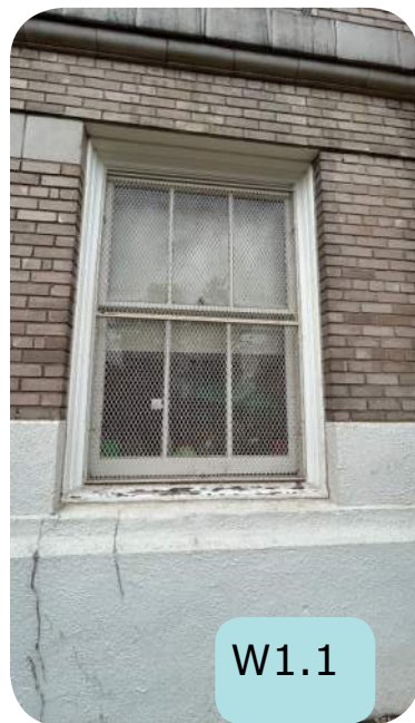
Level 1 Double hung windows with protective expanded steel mesh at 1913 Building
