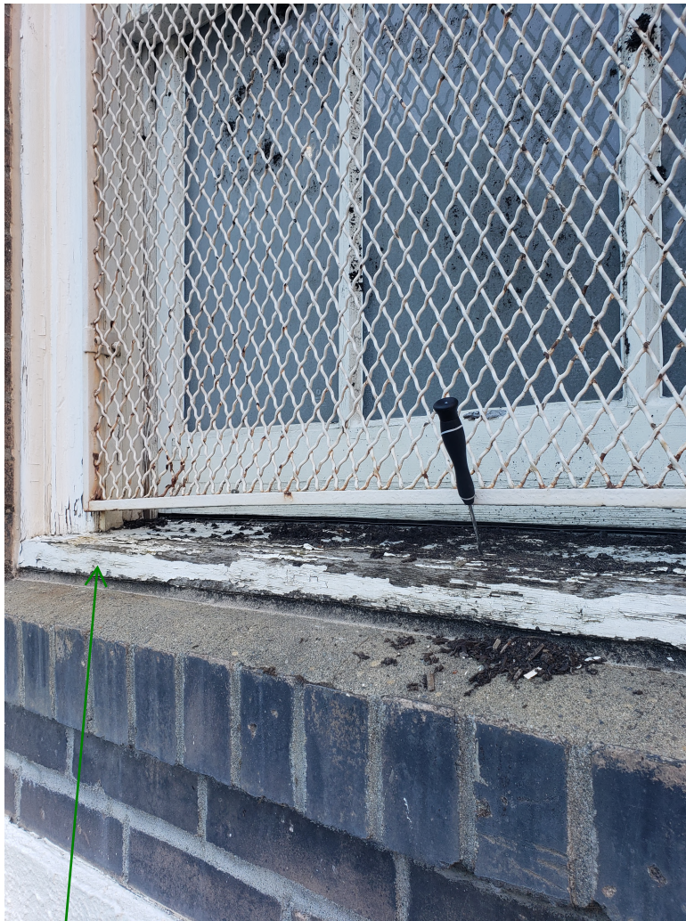
The restroom window sills at the 1913 projecting one story building at the rear are rotted due to the protective expanded, steel mesh and smaller window area causing leaves and debris to fill the window cavity.
