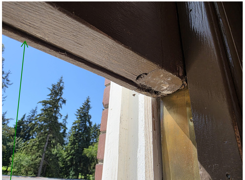
Existing groove in window sash to be used to install weatherstripping
