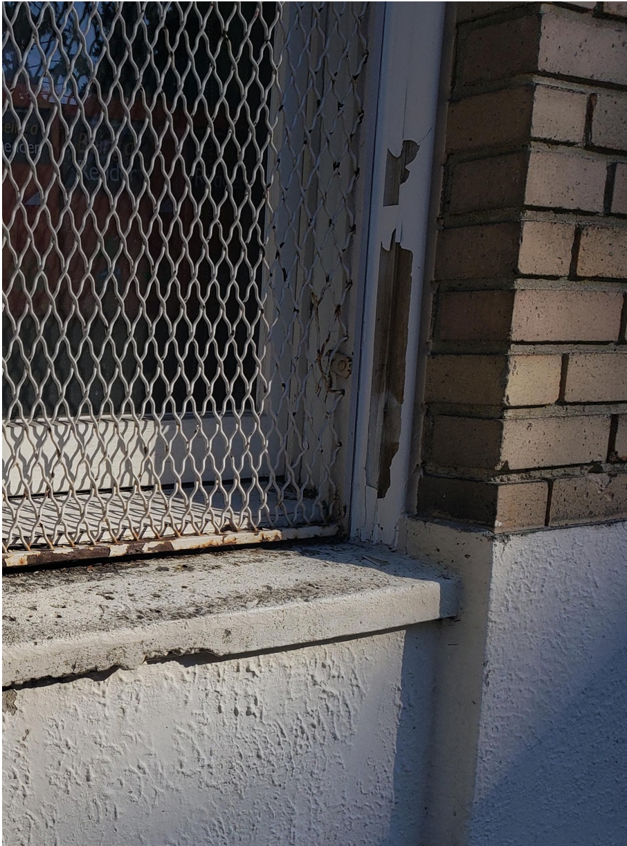
1940 Ground floor, classroom windows have protective expanded steel mesh on the exterior. There are some damage to the wood window frame where the expanded steel mesh is attached along with chips in the paint on the jambs. The exterior window sill has moderate damage due to its skyward facing nature.
