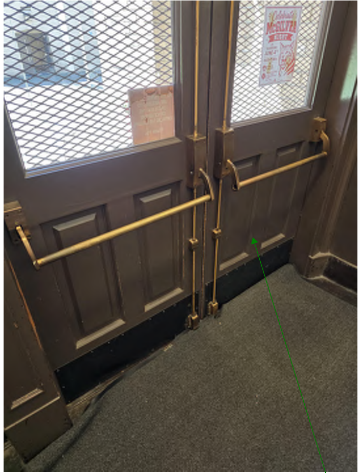
Brass door hardware. Unknown whether they are original or historic match. Back double door interior side is in good condition with some scratches to the paint
