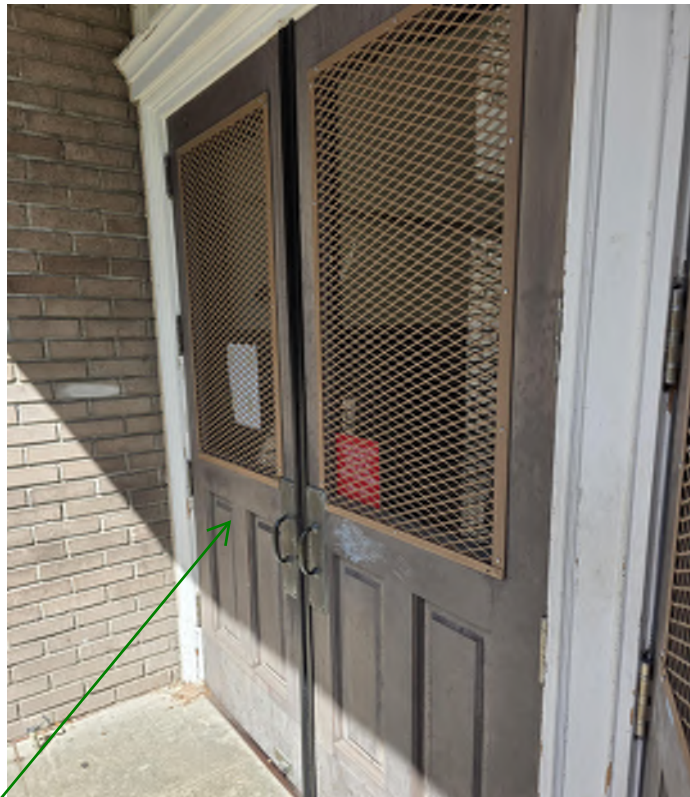
Exterior of Back double door and transom is in good condition, protected from the weather by doors setback with floor above providing protection from the elements. The paint appears faded due to its consistent use over the years.
