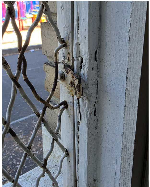
1940 Ground floor, classroom windows have protective expanded steel mesh on the exterior. There are some damage to the wood window frame where the expanded steel mesh is attached along with chips in the paint on the jambs. The exterior window sill has moderate damage due to its skyward facing nature.
