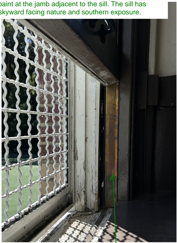
The metal jamb frame is in good condition
