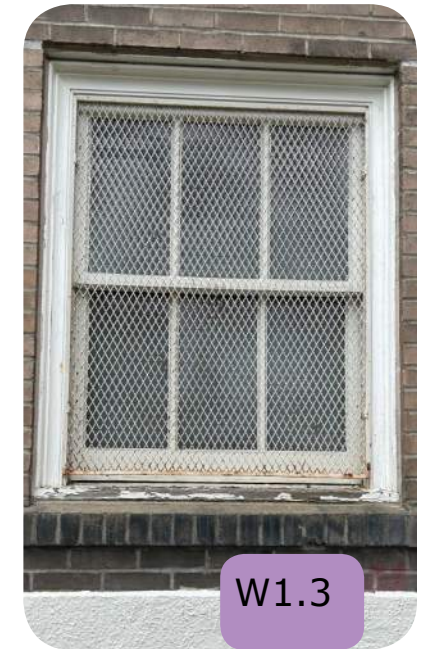
Level 1 Boiler Room and Restroom Double Hung windows with wire grilles
