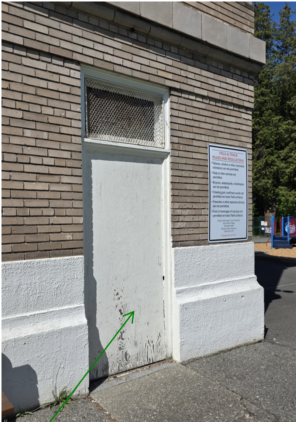
South East, ground floor corner door at music room was infill in 2002 when cafeteria was relocated
