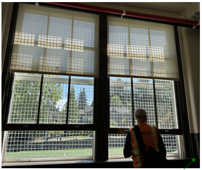
The metal jamb frame is in good condition
