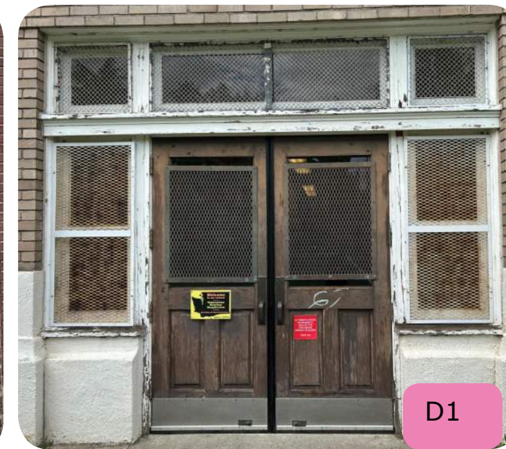
Level 1 Double Wood Door with half lite, relites and transoms.
