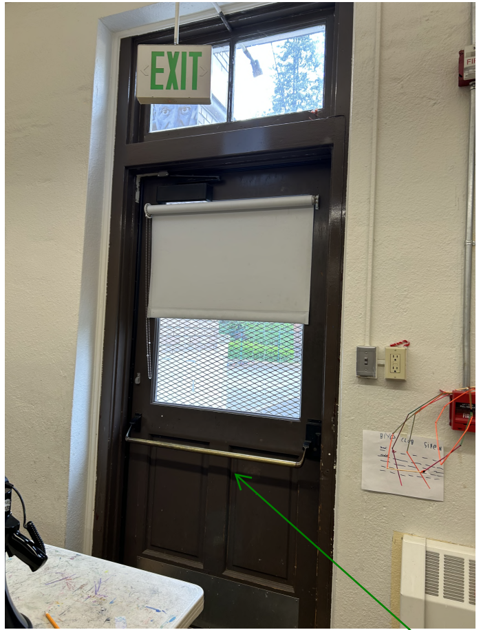
Interior paint, frame, trim and door panel is in good condition.
