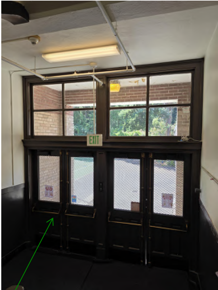
Brass door hardware. Unknown whether they are original or historic match. Back double door interior side is in good condition with some scratches to the paint
