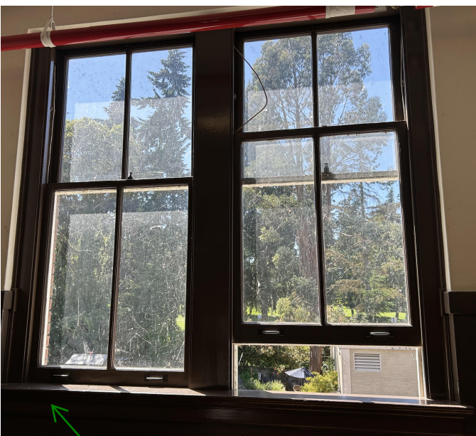
The Interior case work shows some signs of wear, with chips and scratches in the paint but overall is in good condition
