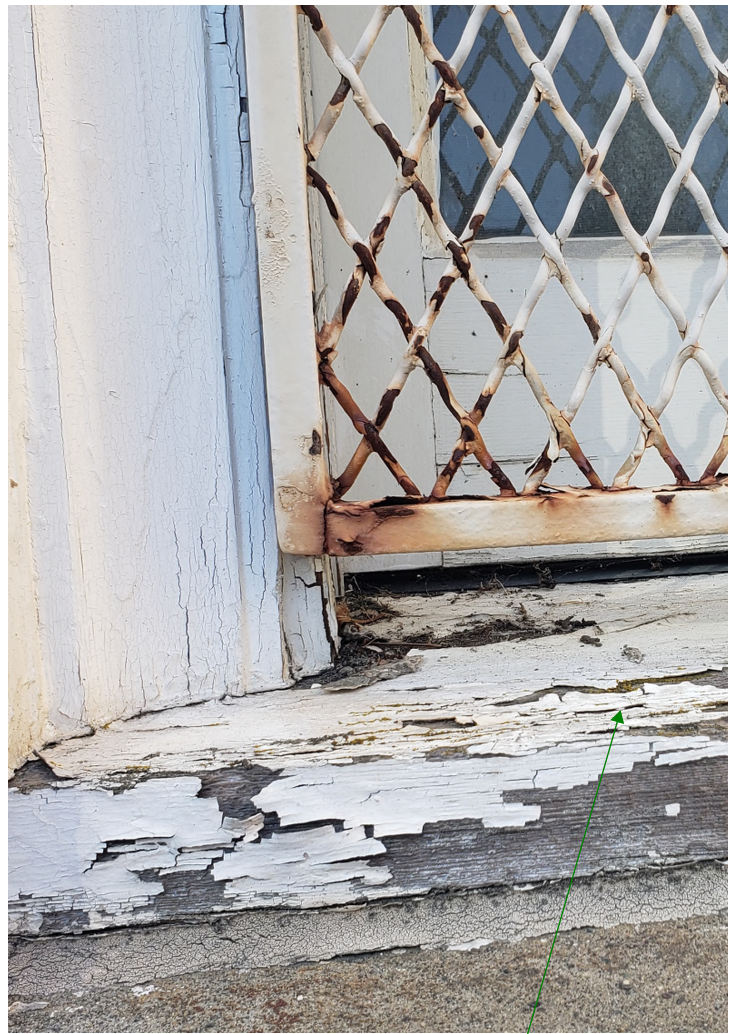
The restroom window sills at the 1913 projecting one story building at the rear are rotted due to the protective expanded, steel mesh and smaller window area causing leaves and debris to fill the window cavity.
