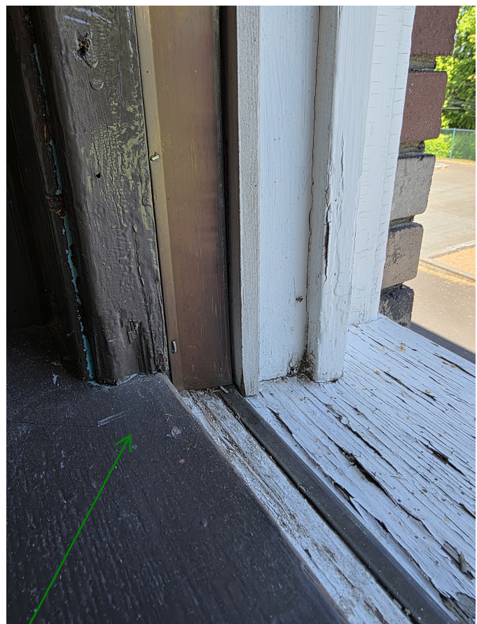
Interior case woks in good condition with some chips or scratches in the paint
