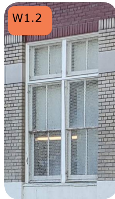
1940 Level 1 Two operable, two over two single-hung with two, fixed two-light sash with wire grilles
