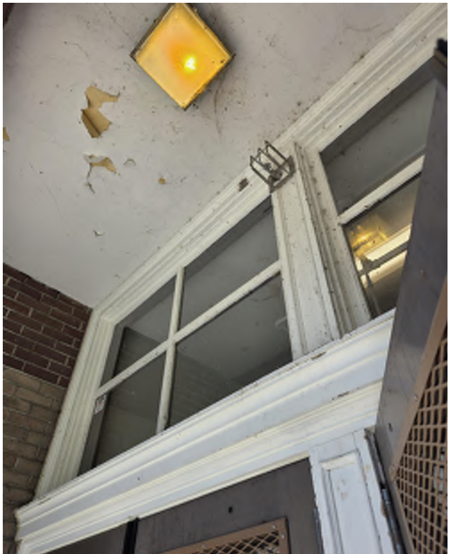
Exterior of Back double door and transom is in good condition, protected from the weather by doors setback with floor above providing protection from the elements. The paint appears faded due to its consistent use over the years.
