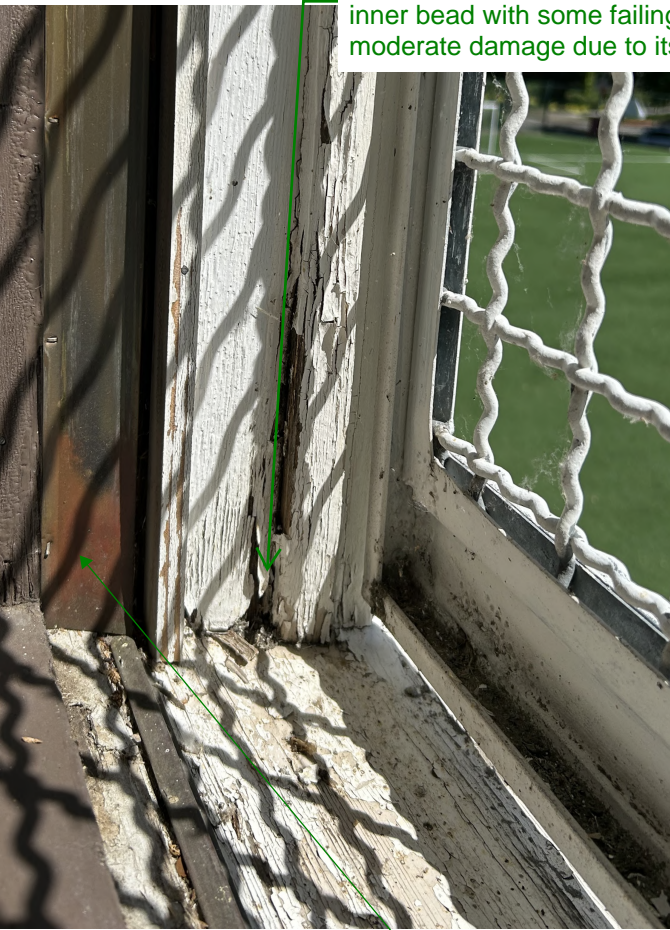
The metal jamb frame is in good condition
