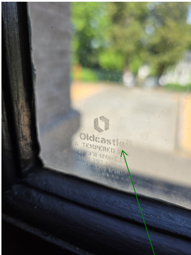
Previously replaced window glazing
