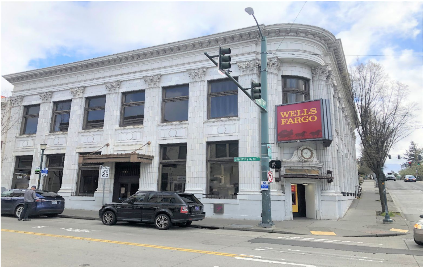
Before construction - Exterior at purchase as a closed down Wells Fargo Bank. Exterior has failing paint, faded canopies, tucking on stone, cracked glazing, lack of lighting, etc.
