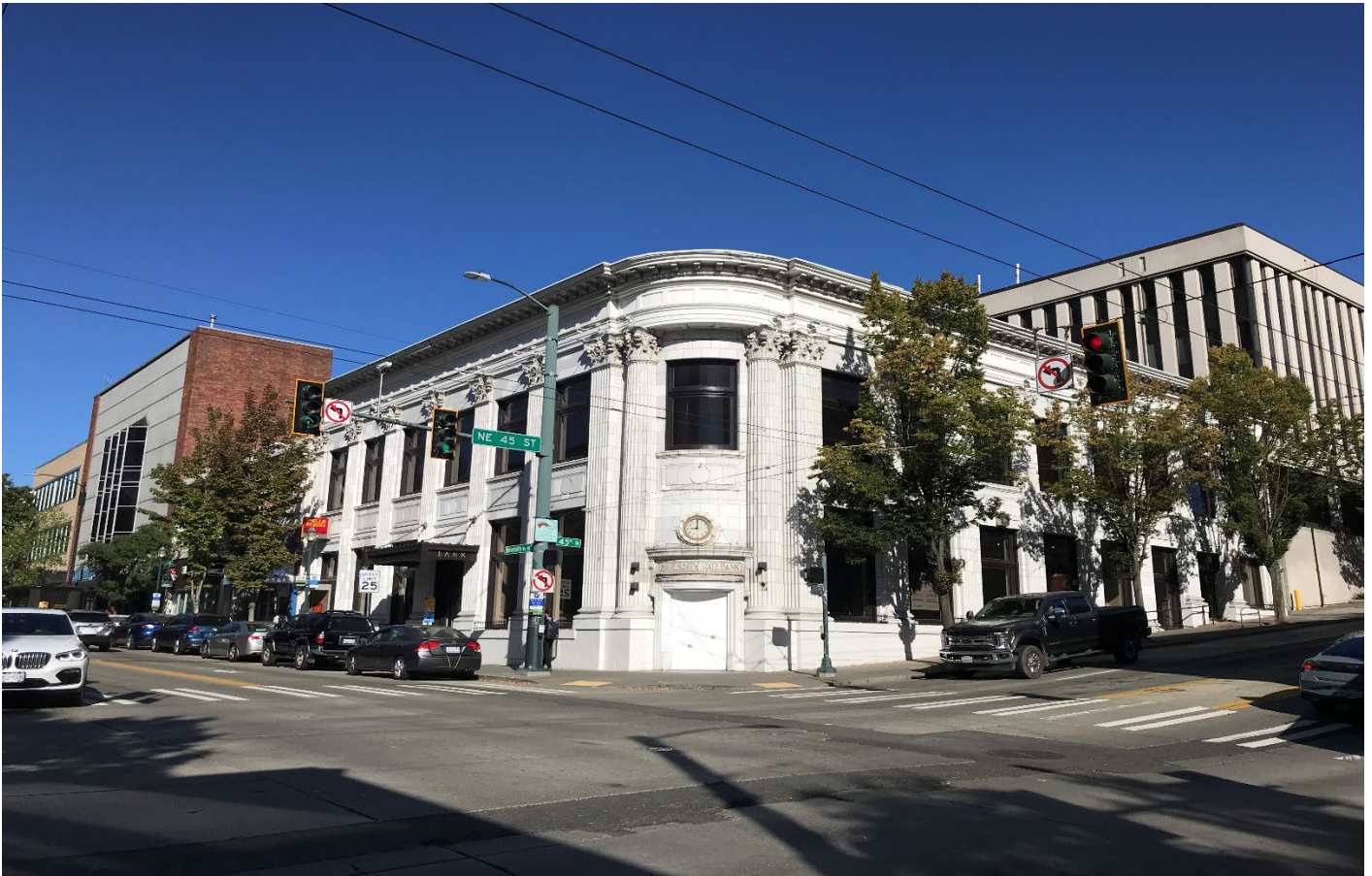
Before construction - Exterior at purchase as a closed down Wells Fargo Bank. Exterior has failing paint, faded canopies, tucking on stone, cracked glazing, lack of lighting, etc.
