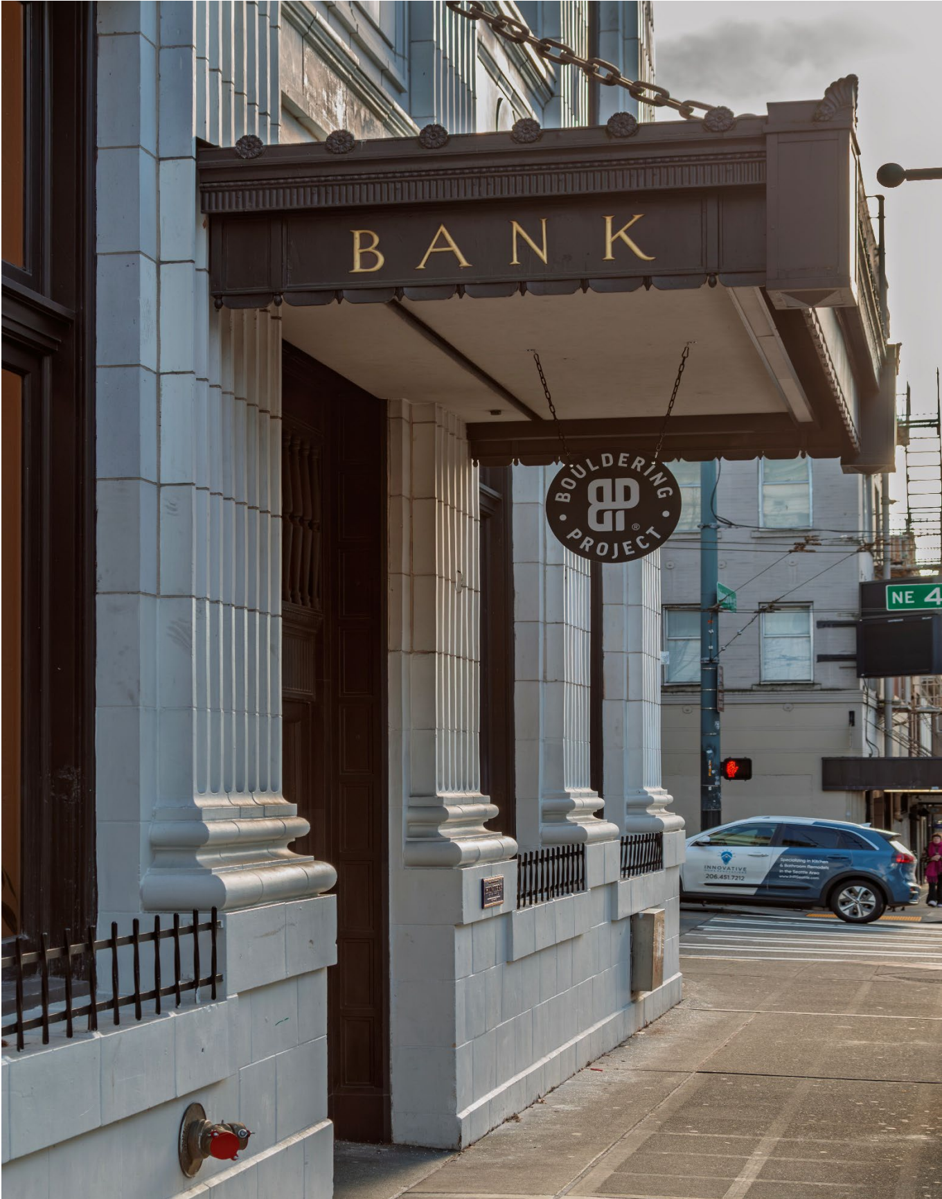
After construction - New Bouldering sign at entry, looking S.
