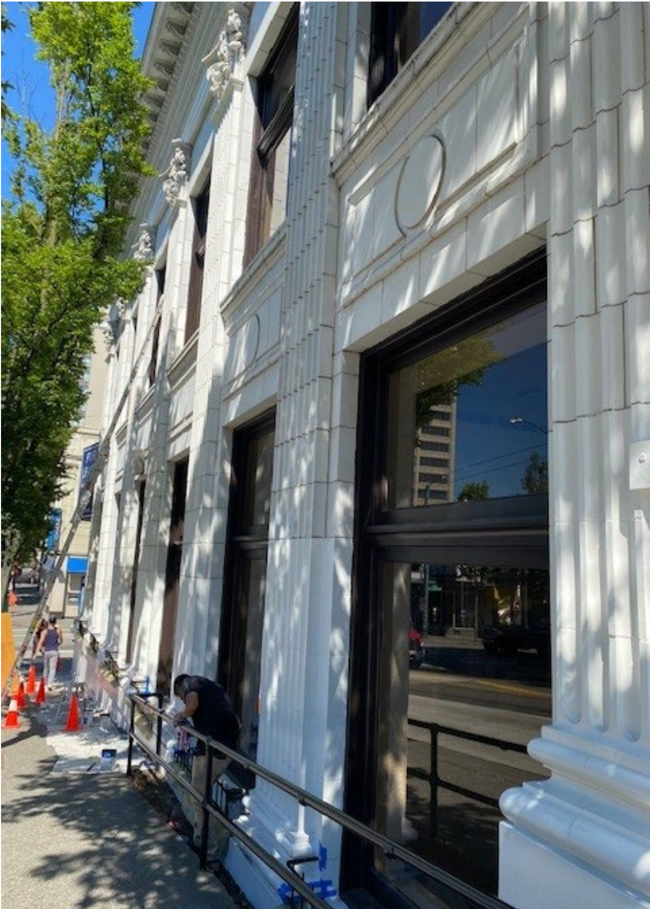
During final LL construction- 45th street facade during rehab
