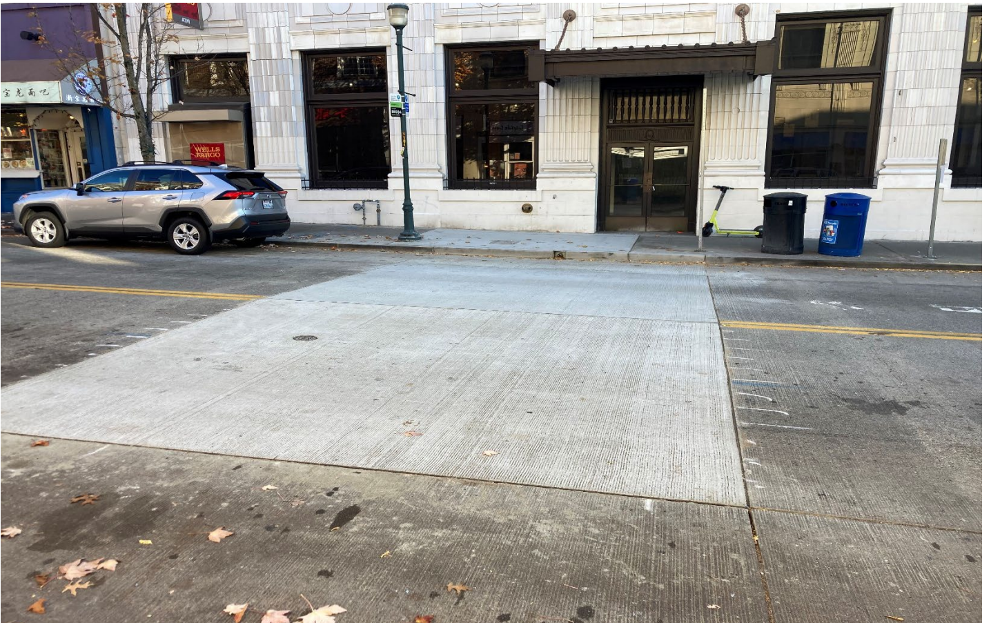
Post LL construction- New street panels after bringing sprinklers to site looking E.
