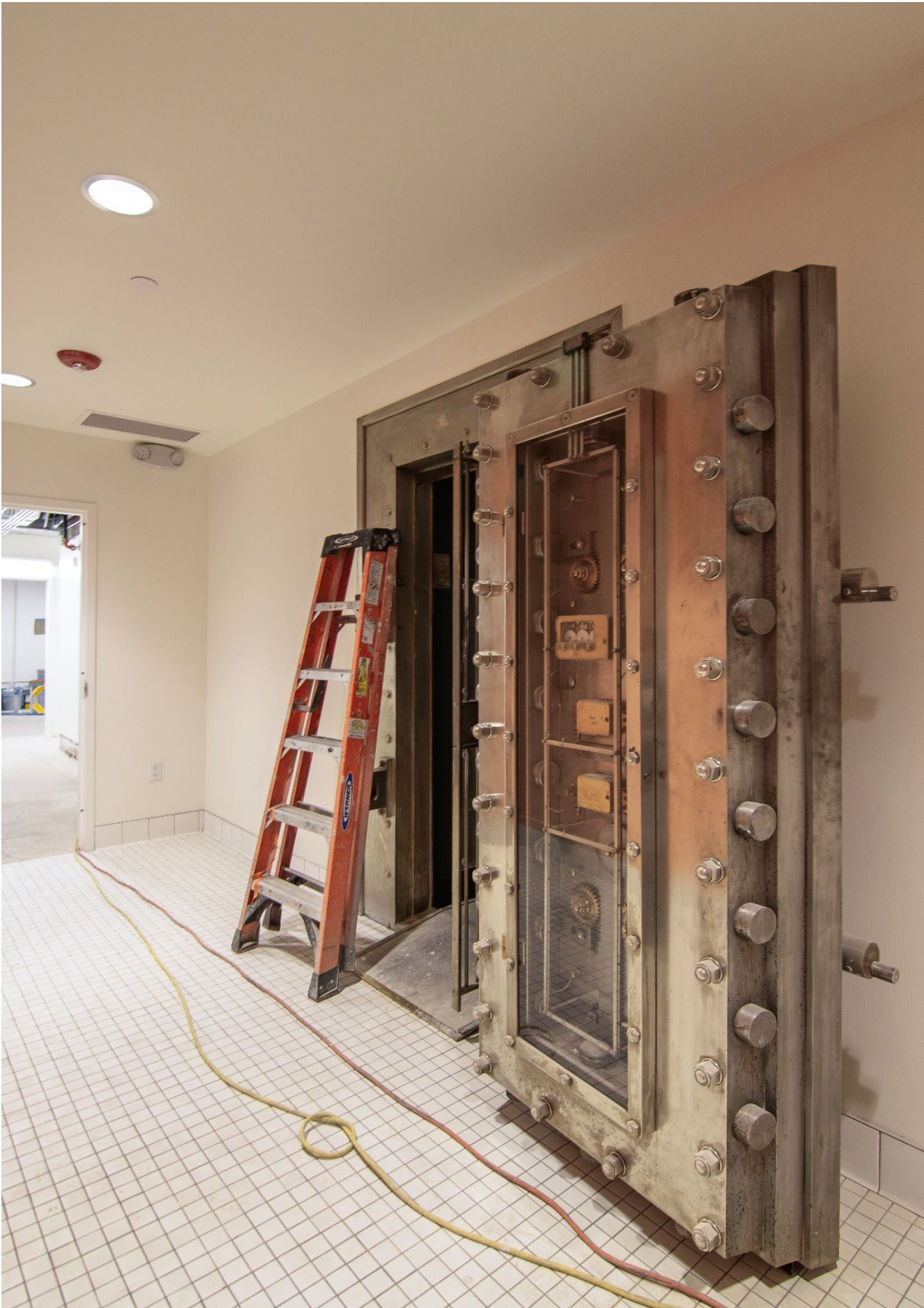
During construction - Vault 2 work, new flooring during TI, basement looking S.
