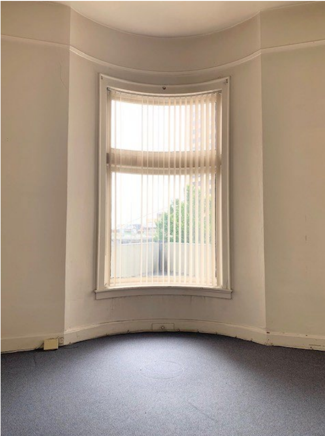
Before construction – Typical second floor office at purchase. Second floor looking SW.
