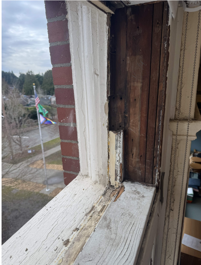
Upper frame with pivoting transom sash removed
