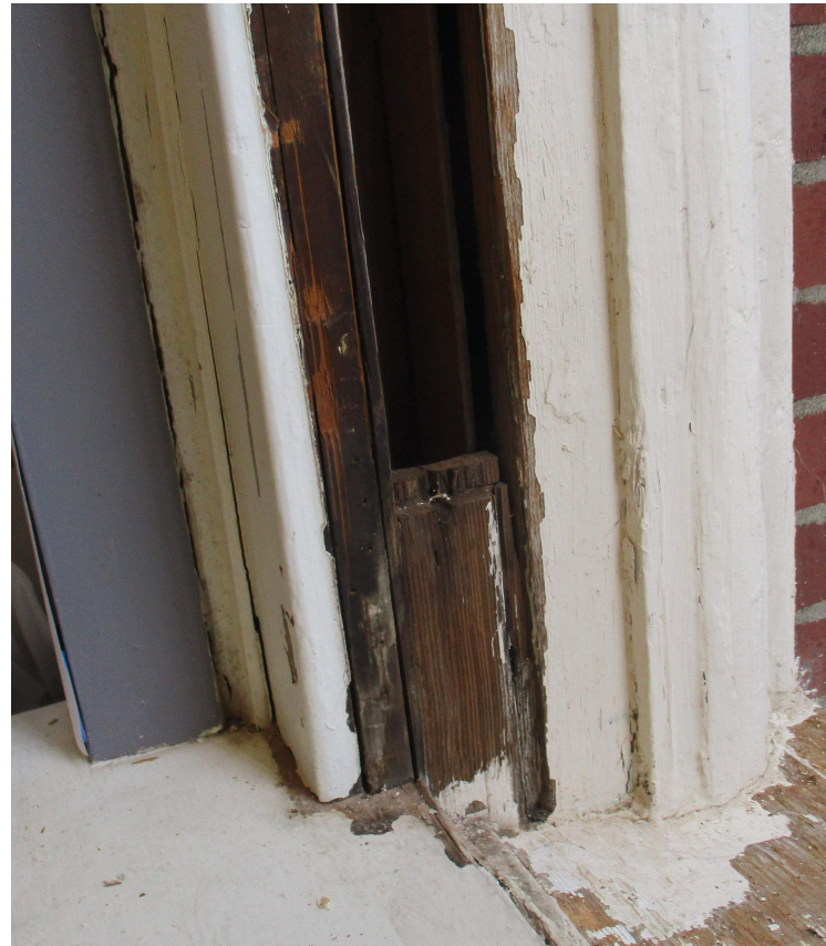
Lower frame with double hung sashes removed
