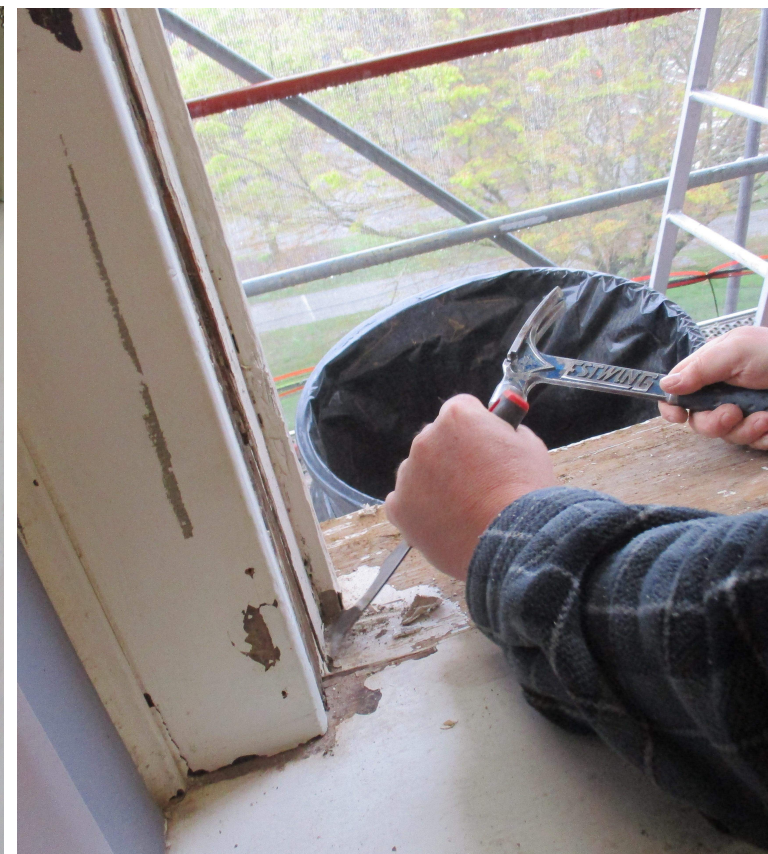
Careful removal of exterior sealants and minor wood rot
