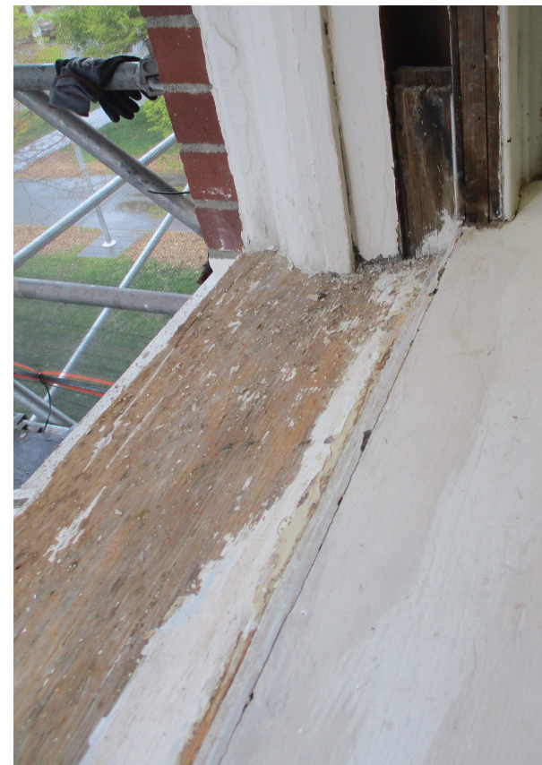
Subsill with loose paint removed and prior to epoxy repairs
