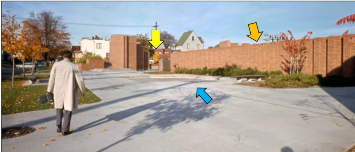
West side of substation, NE view showing tower separate from substation. SMA 19554 (1967-1970)
