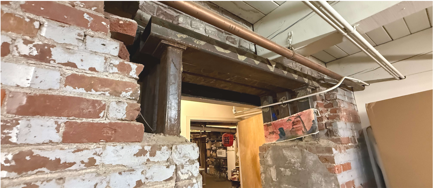
Disconnect between different portions of the building.
