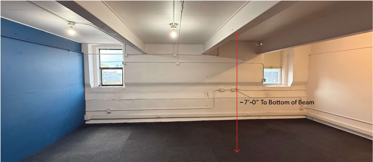
The original design for drying malts required spaces with proportions that are difficult to re-purpose into new uses, especially the original floor to floor heights
