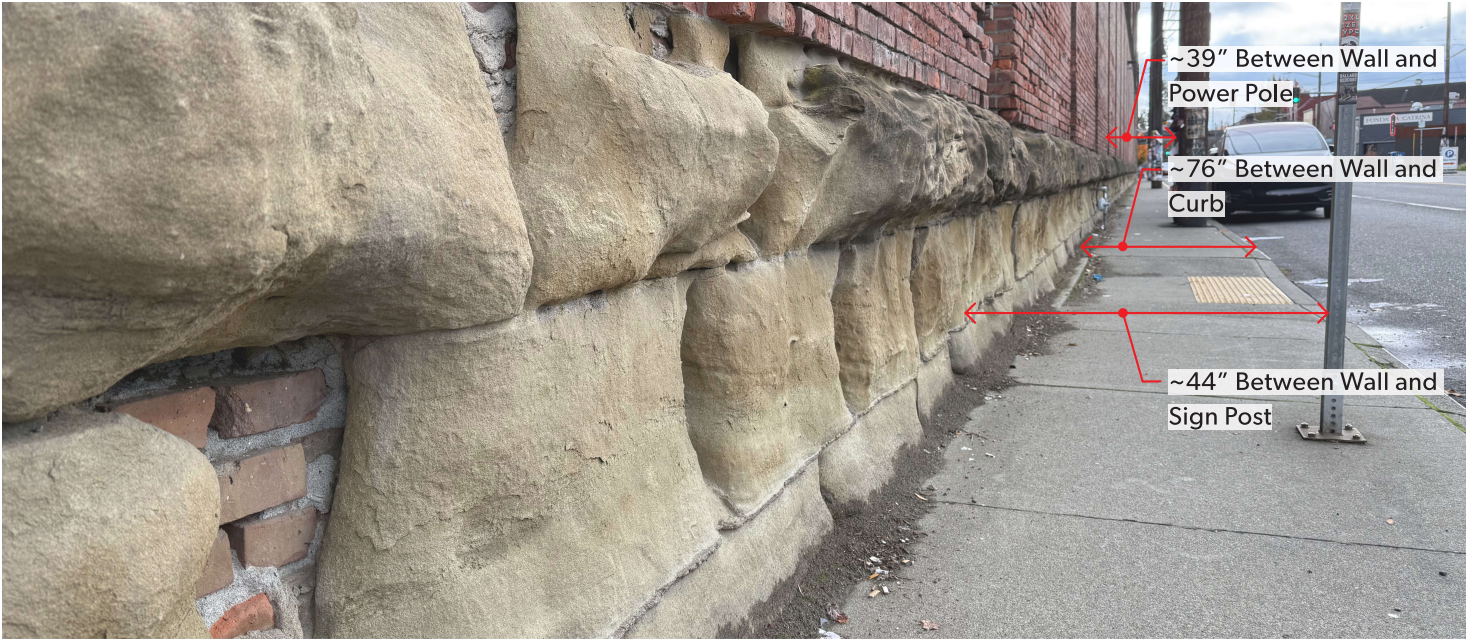
The condition of the masonry, both brick and stone, along Airport Way has significant deterioration which is assumed to be occurring due to it's proximity to heavy traffic. The usability of the sidewalk is hampered by the location of the west facade in relation to the curb providing sub-optimal. The sidewalk width is further reduced by street appurtenances.
