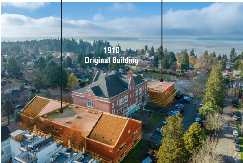
1990 additions to East and West side of school
