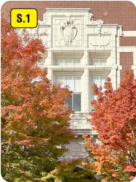
Level 2-3 Operable + fixed windows at ornamental Terra cotta facade areas.
