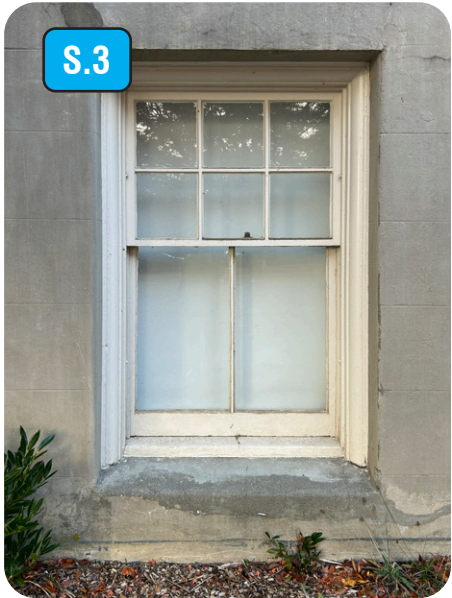
Level 1 Operable Windows at Kindergarden classrooms.
