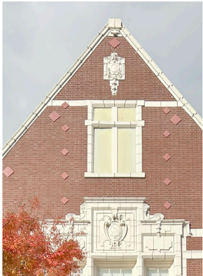
Ornamental Terra cotta facade elements typical of early 20th century revival styles derived from the English Jacobean Manor house
