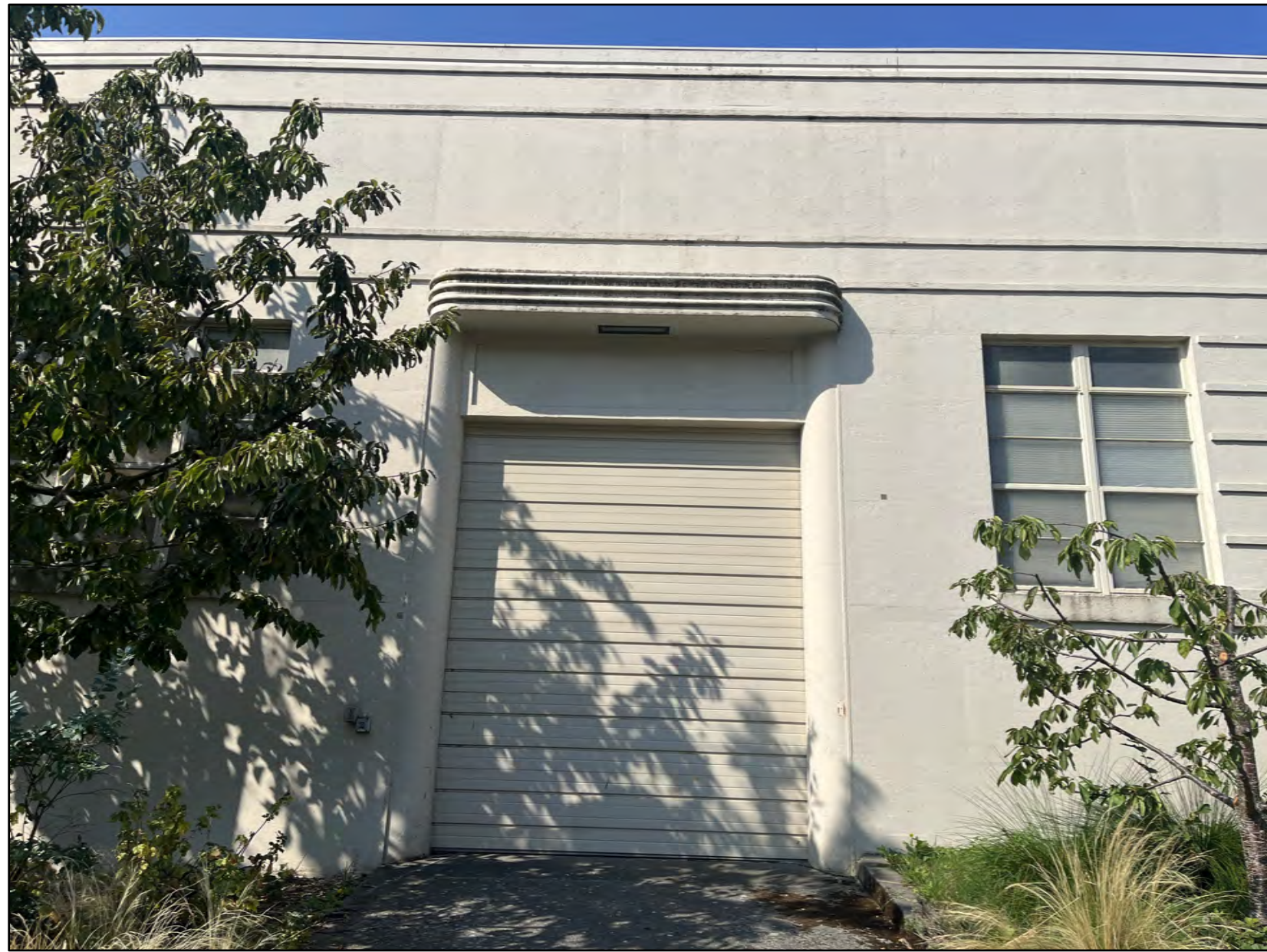
EXISTING GARAGE DOOR PHOTO
