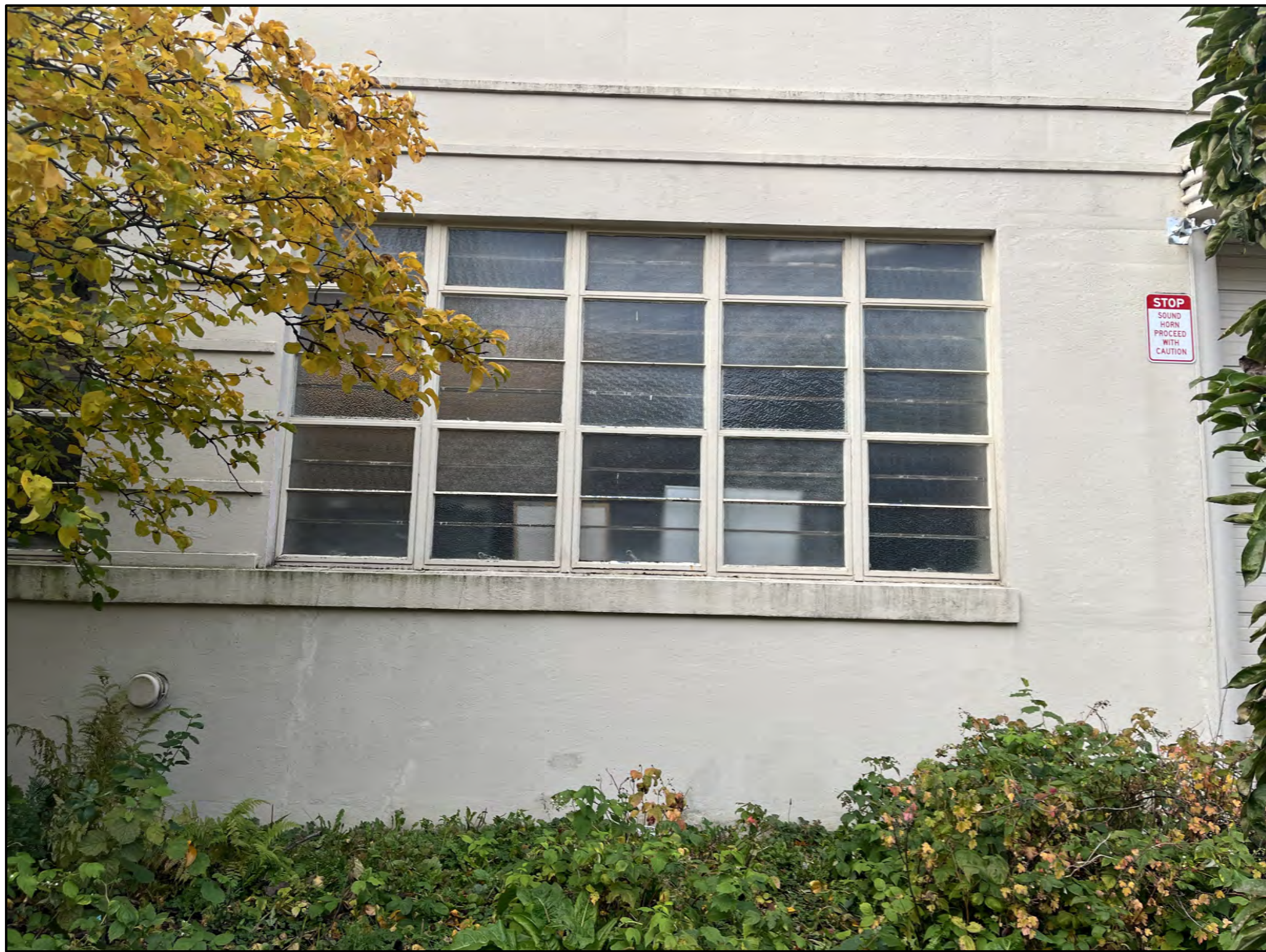
EXISTING WINDOW PHOTO NO SCALE
