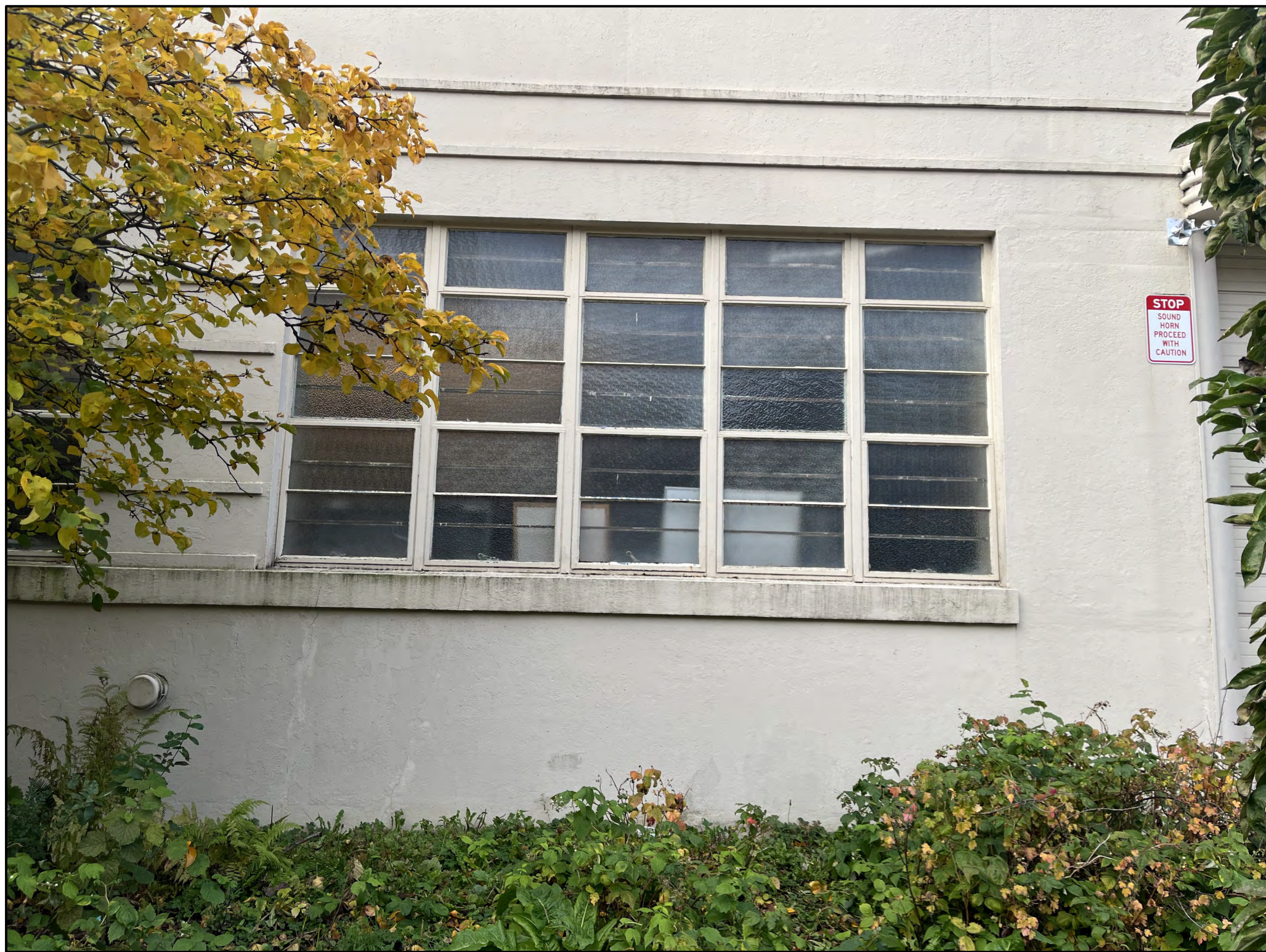
EXISTING WINDOW EXTERIOR 4 NO SCALE
