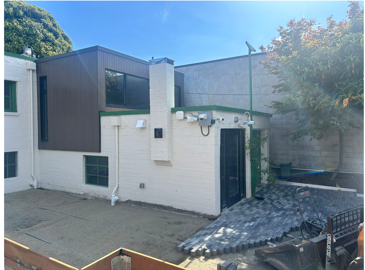
Back of house, landscaping in process, photo courtesy of Wing Luke Museum
