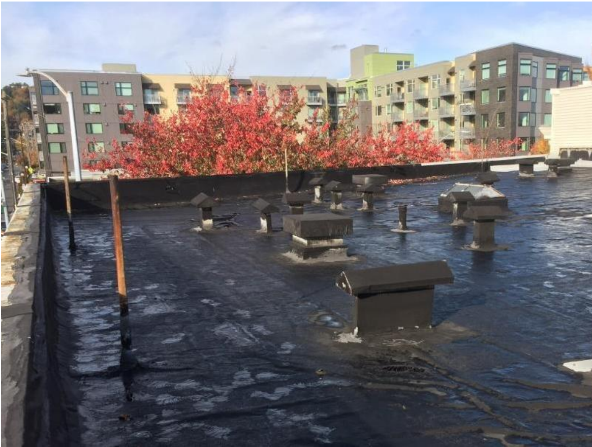
Old Roof prior to seismic upgrades and new roofing.
