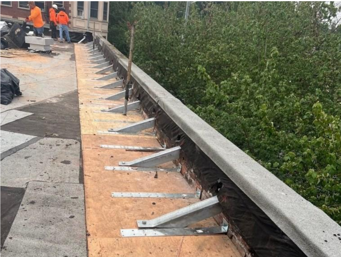
New parapet bracing west wall.
