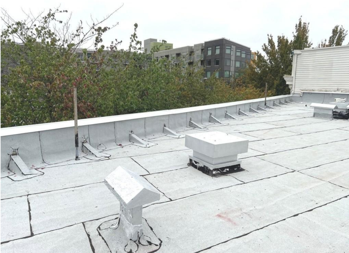
New Roof, new flashing and new cap metal, along with new seismic parapet bracing.
