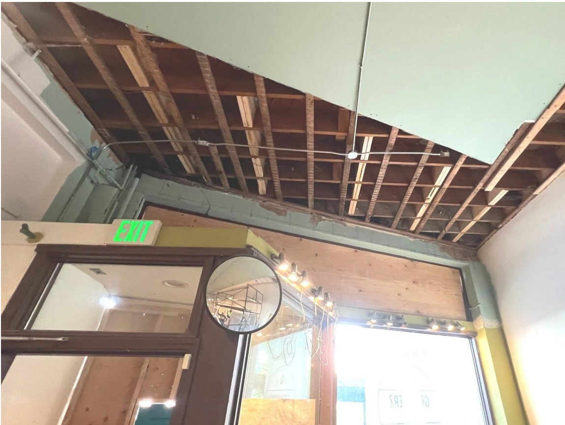
Wall ties and new blocking on West ceilings in 4820 Rainier Ave. S.
