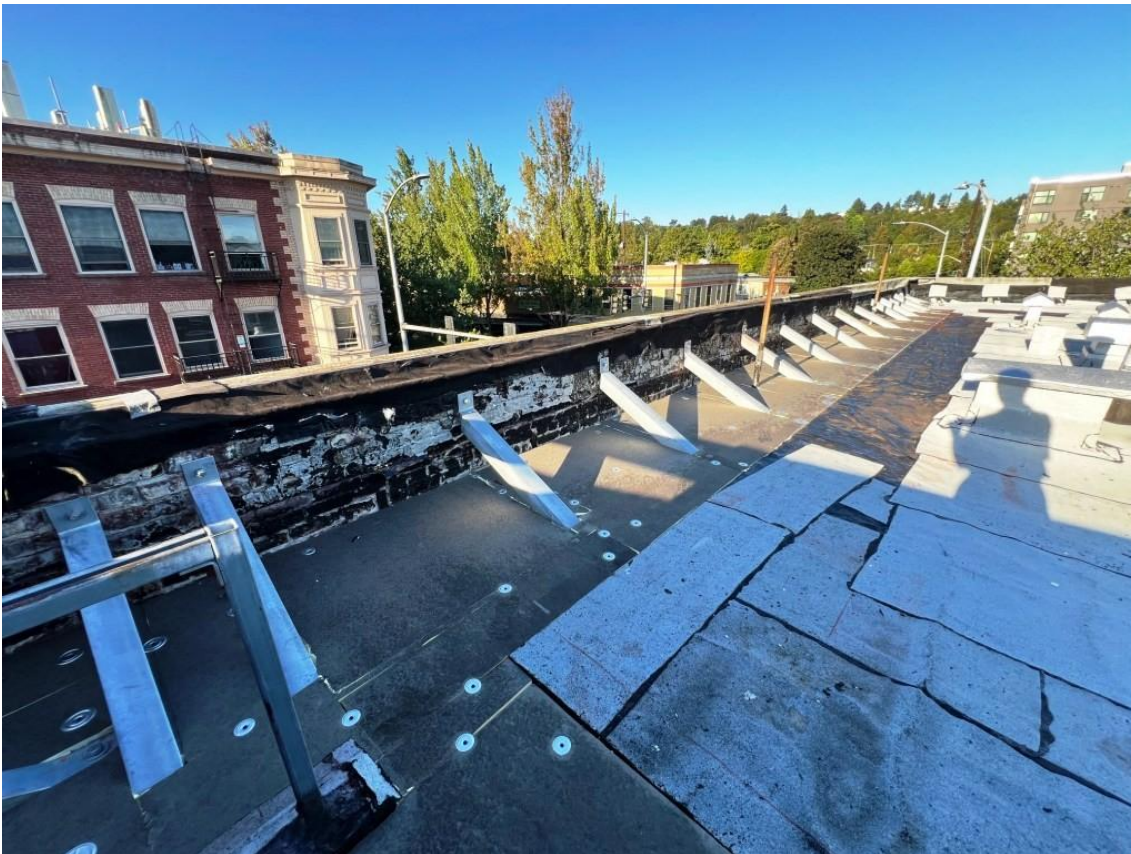
New parapet roof bracing on the south wall.
