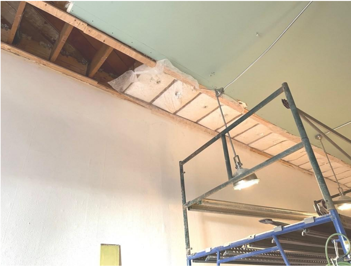
New blown-in ceiling insulation.
