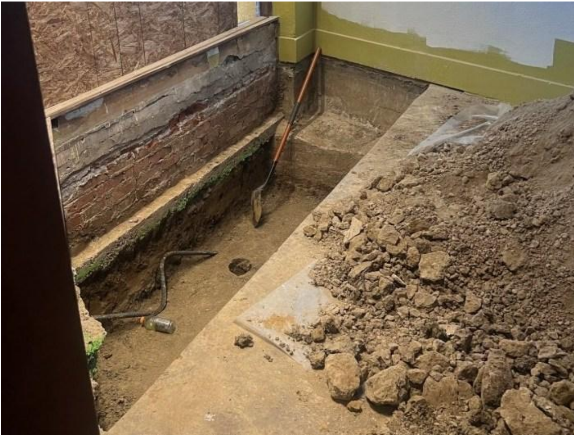
Excavation for new grade beam to support new brace frame.
