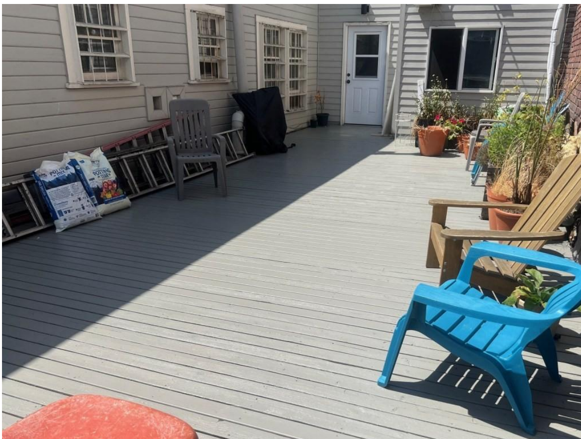
New deck rails as needed and new stain installed.
