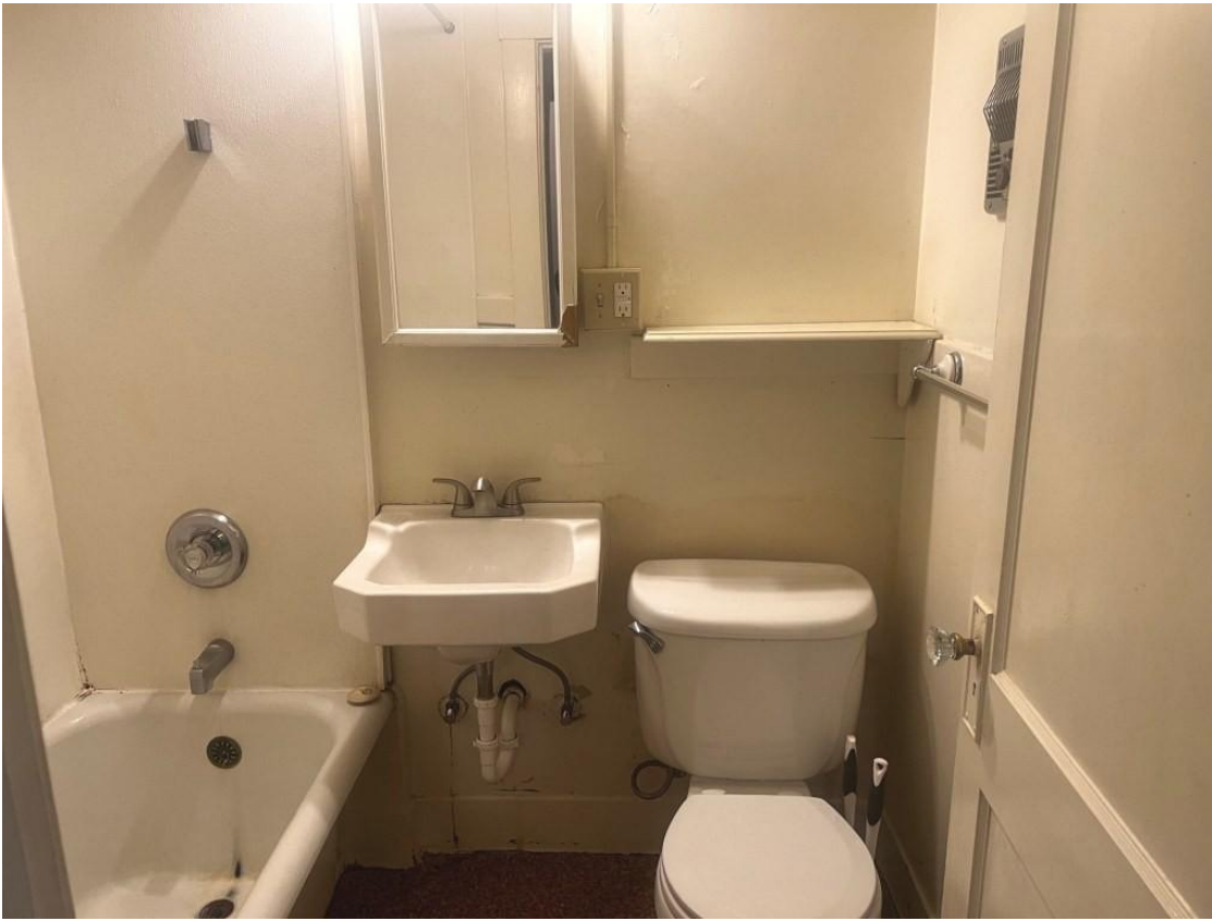
Old Bathroom with non-historic sink and cabinet
