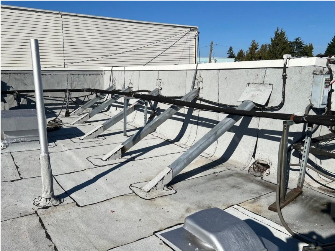
New Bracing and new roof.
