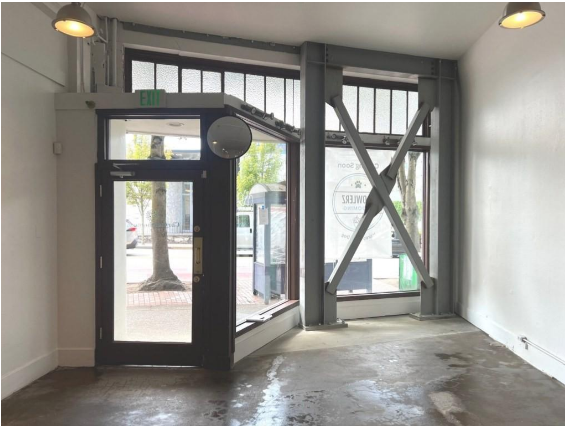
Storefront post seismic brace frame installation.
