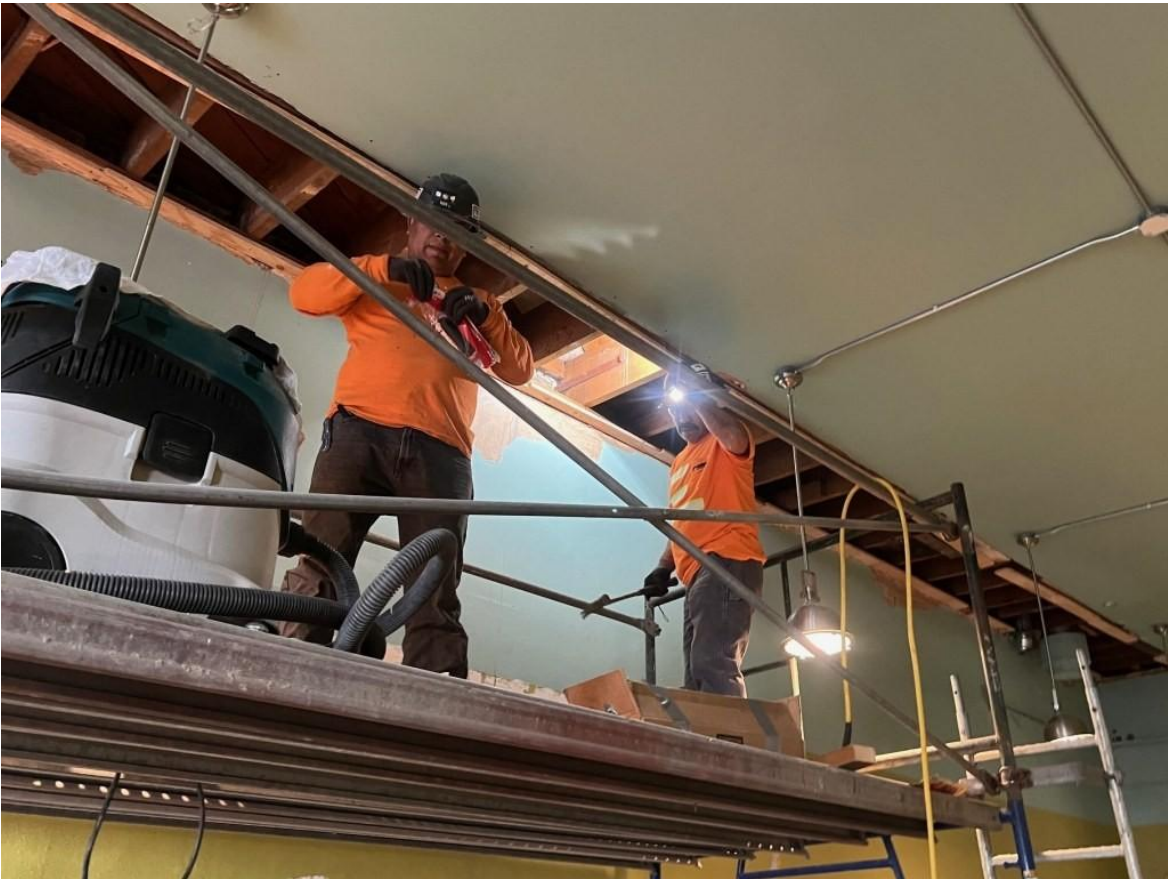
Installation of threaded rods & wall ties on West, North and East ceilings in 4820 Rainier Ave. S.
