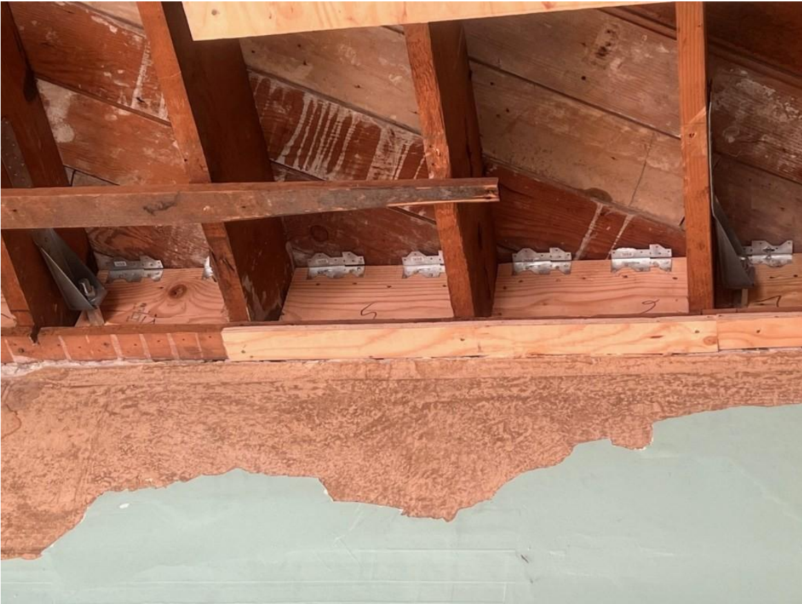
Installation of wood blocking and clips in joist pockets.
