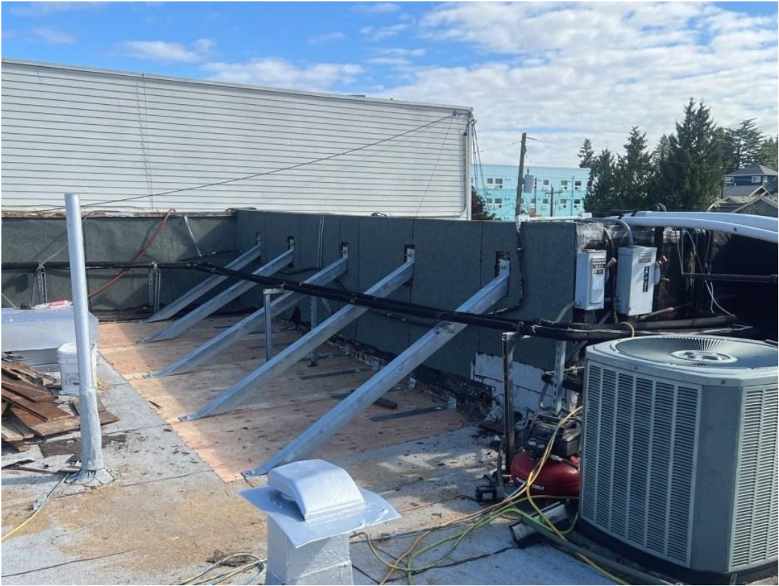
New Parapet bracing in NE corner of roof.
