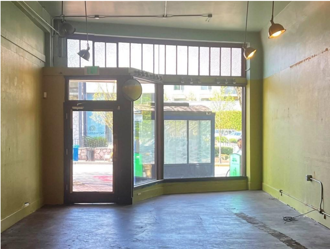
Storefront at 4820 Rainier Ave. S. prior to seismic brace frame installation.
