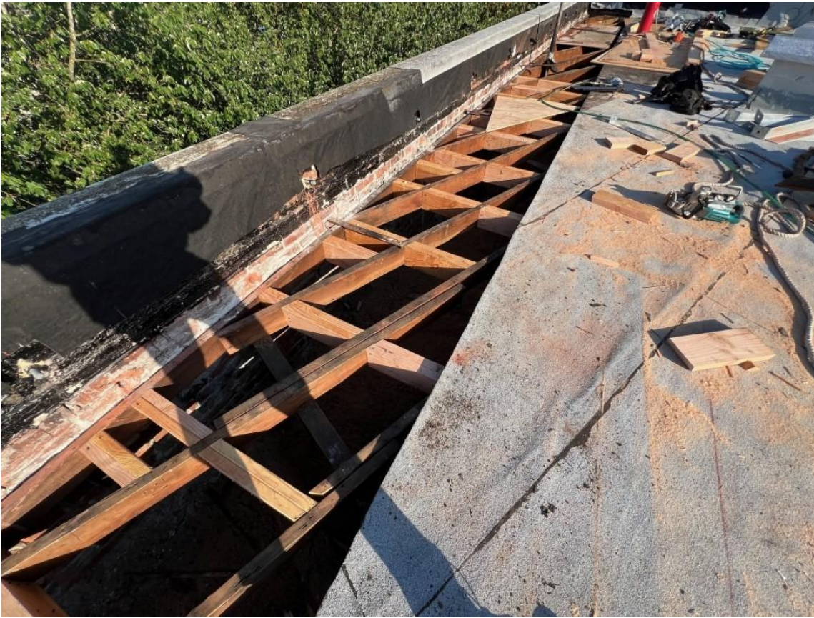
New bracing and blocking for parapet bracing on the west wall.
