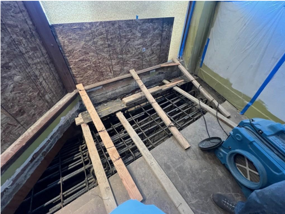
New rebar for grade beam support.
