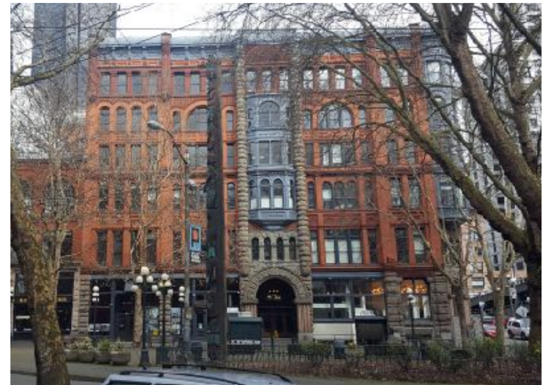
Pioneer Building (1892, Elmer Fisher, alt. 1973-74, Ralph Anderson)
