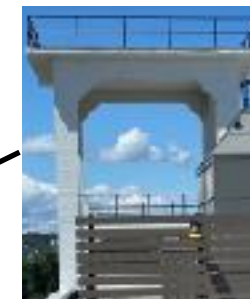
1916 WATERTOWER PLATFORM concrete structure
