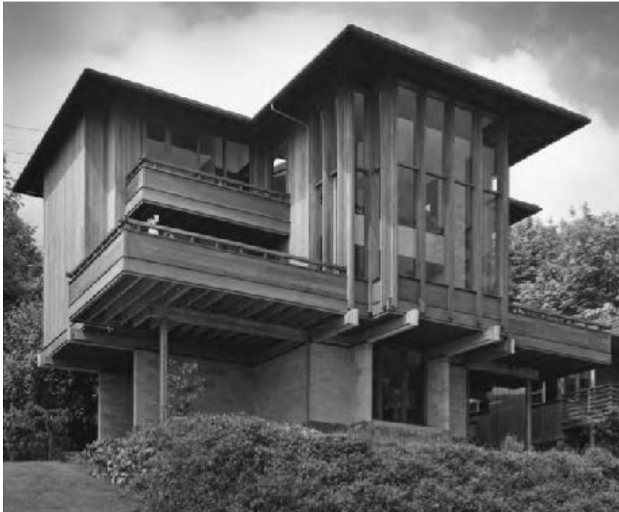
Gordon K. Schowe Residence (1965, Ralph Anderson)
