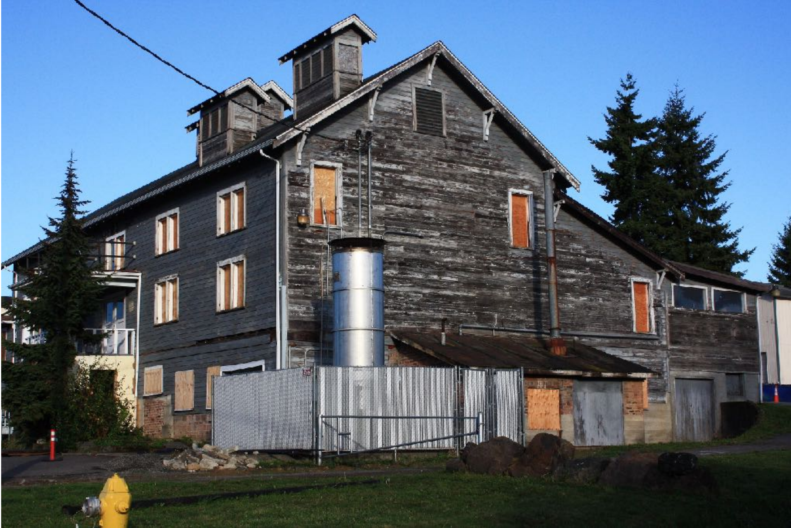
Kirkland Cannery 1936, Works Progress Administration
