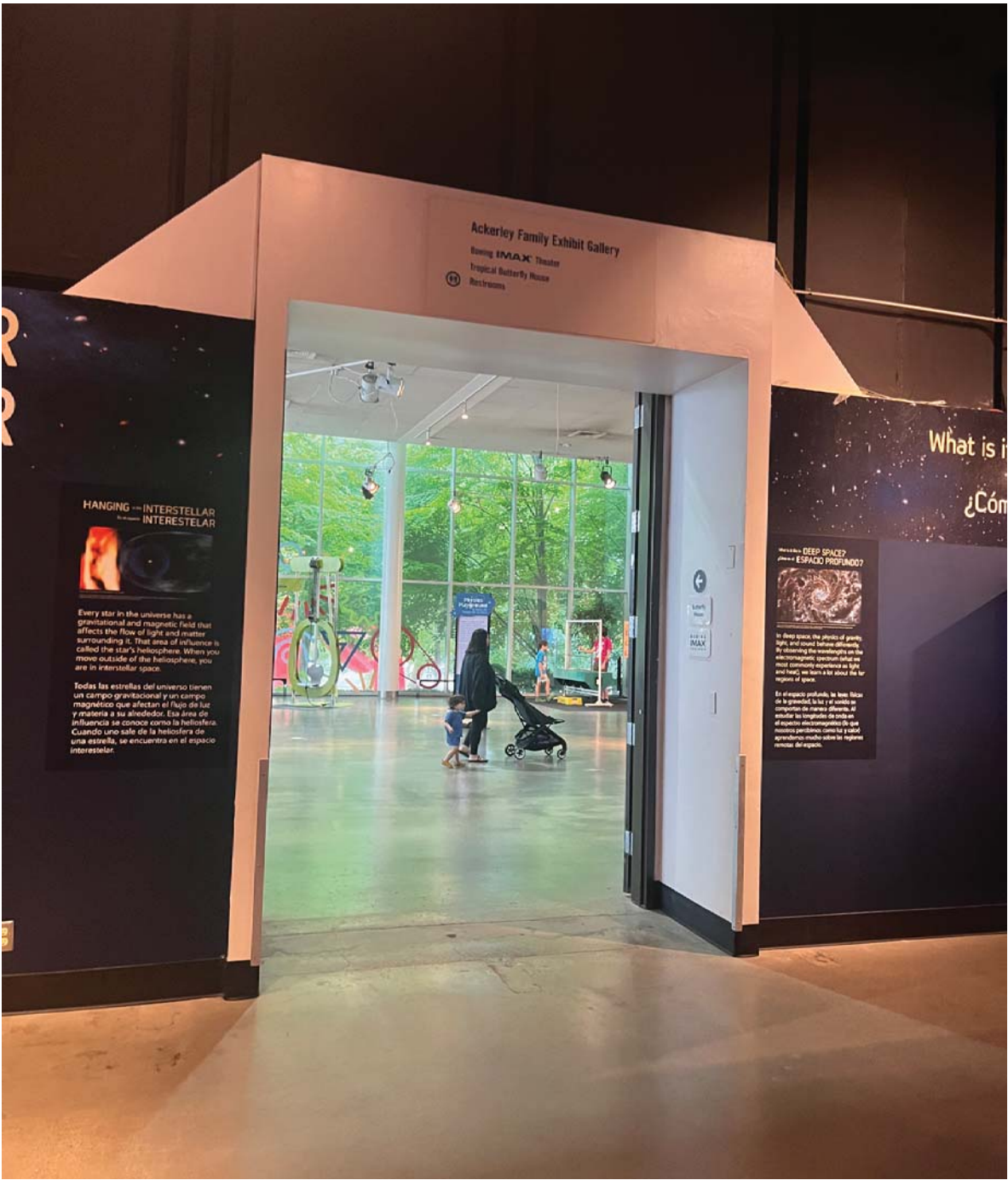
EXISTING DOORS BETWEEN BUILDING 2 AND ACKERLEY PAVILION, PHOTO FROM BUILDING 2 SIDE
