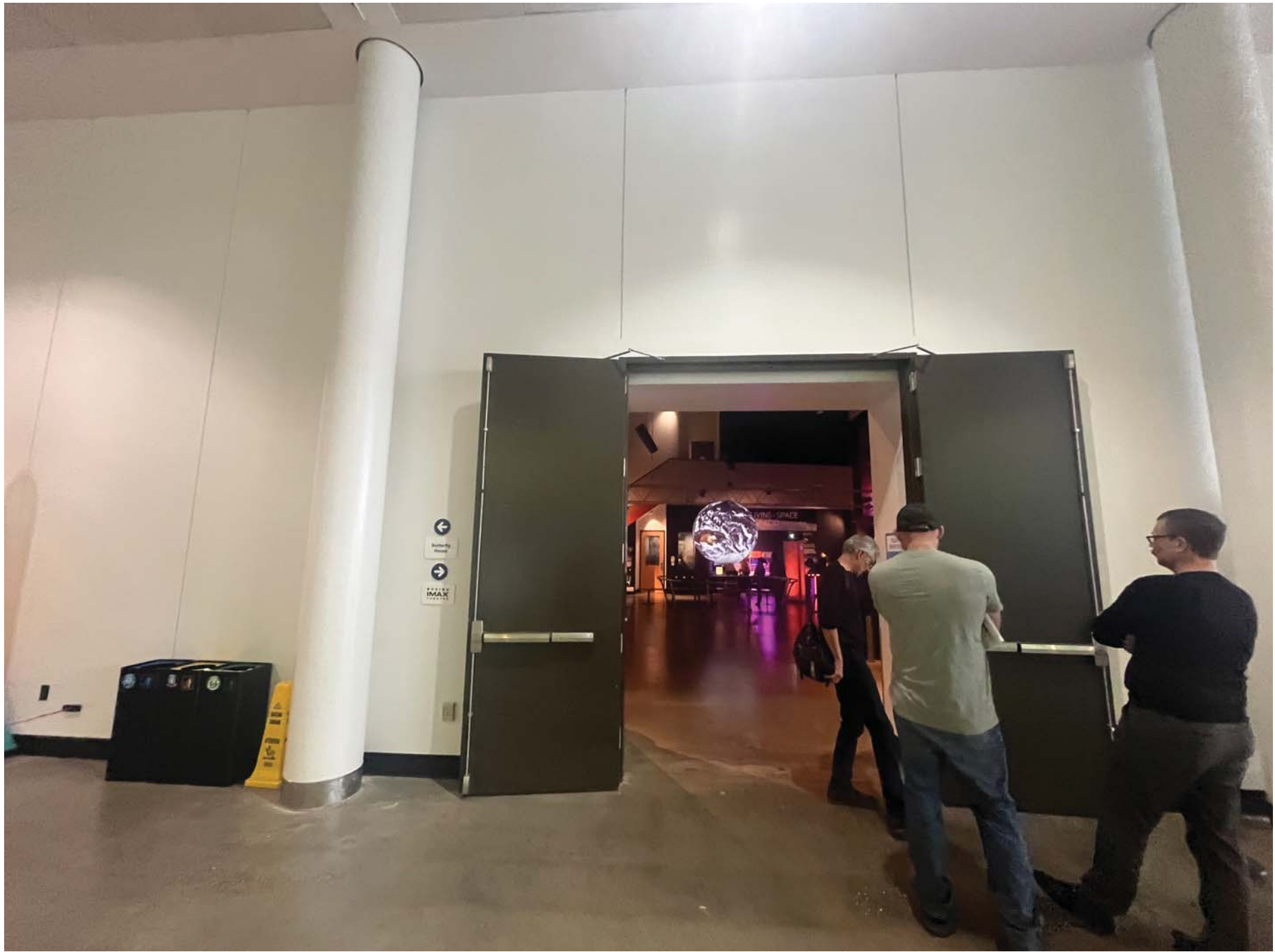
EXISTING DOORS BETWEEN BUILDING 2 AND ACKERLEY PAVILION PHOTO FROM ACKERLEY SIDE
