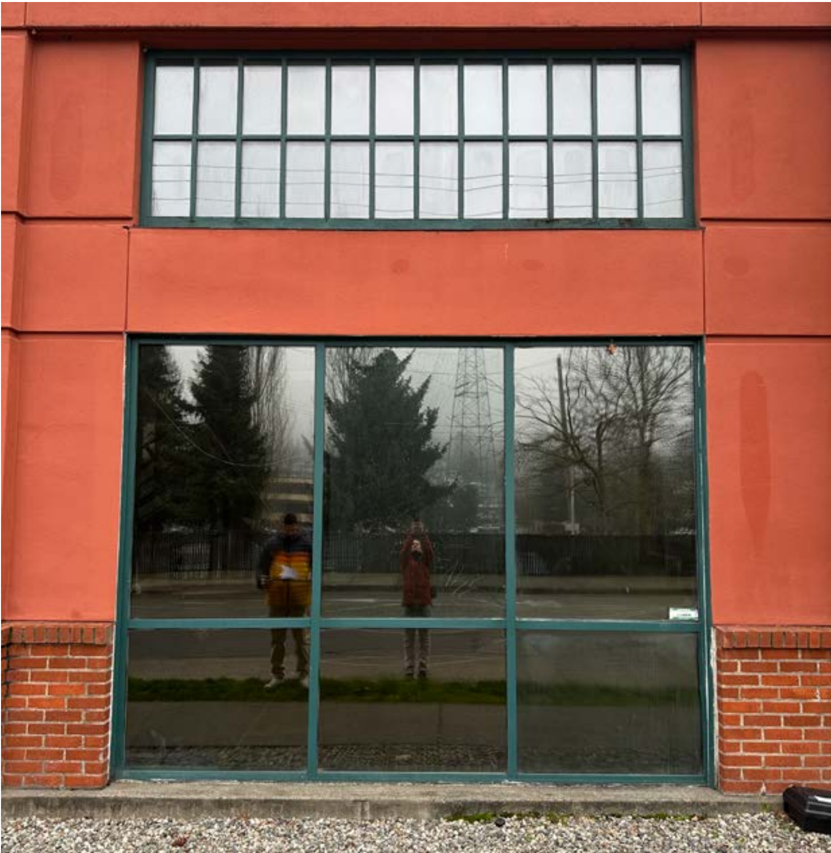
MODERN WINDOW - METAL, BELOW; MODERN WINDOW - WOOD, ABOVE
