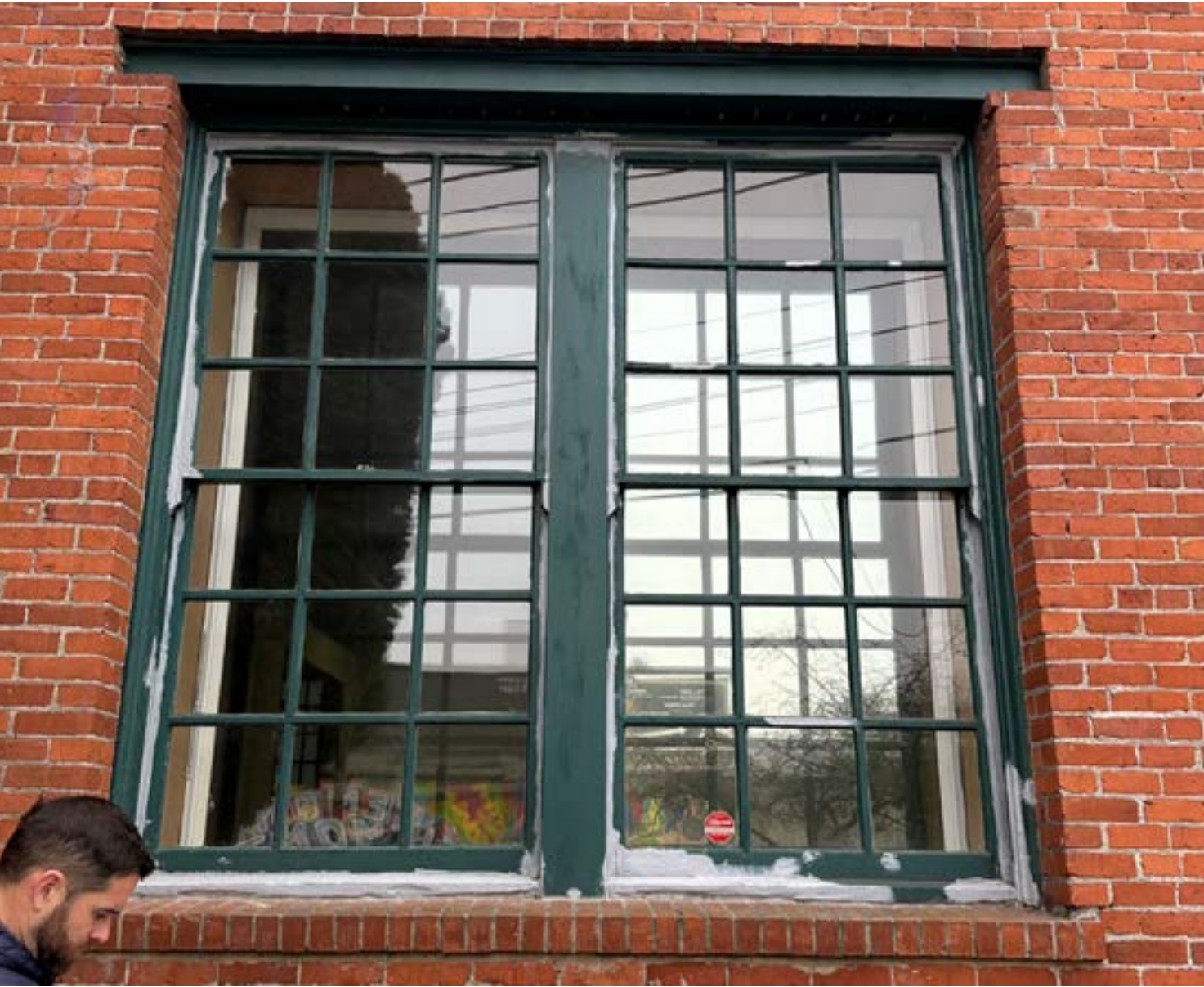
HISTORIC WINDOW - WOOD WITH ADDED INTERIOR VINYL WINDOW
