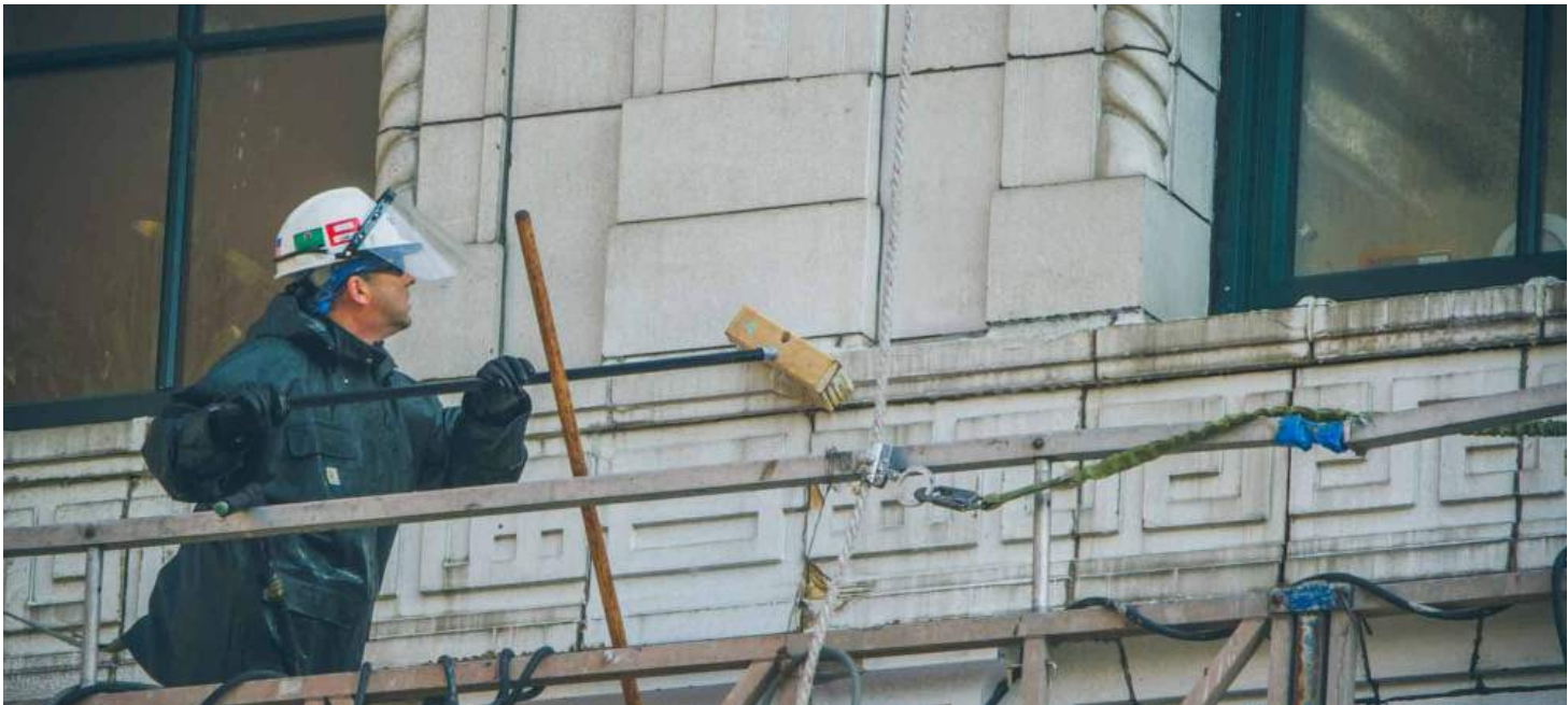
EXAMPLE OF WORKER CLEANING TERRA COTTA FACADE
