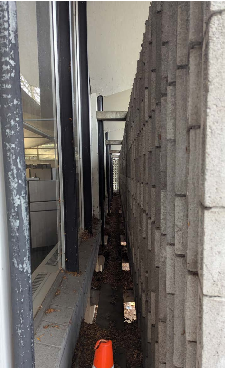
BLOCK WALL SEPARATION FROM BUILDING
