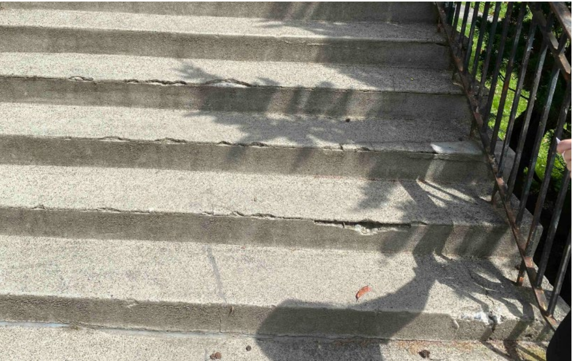
Stair photos taken during construction by DLR Group, April 2024
