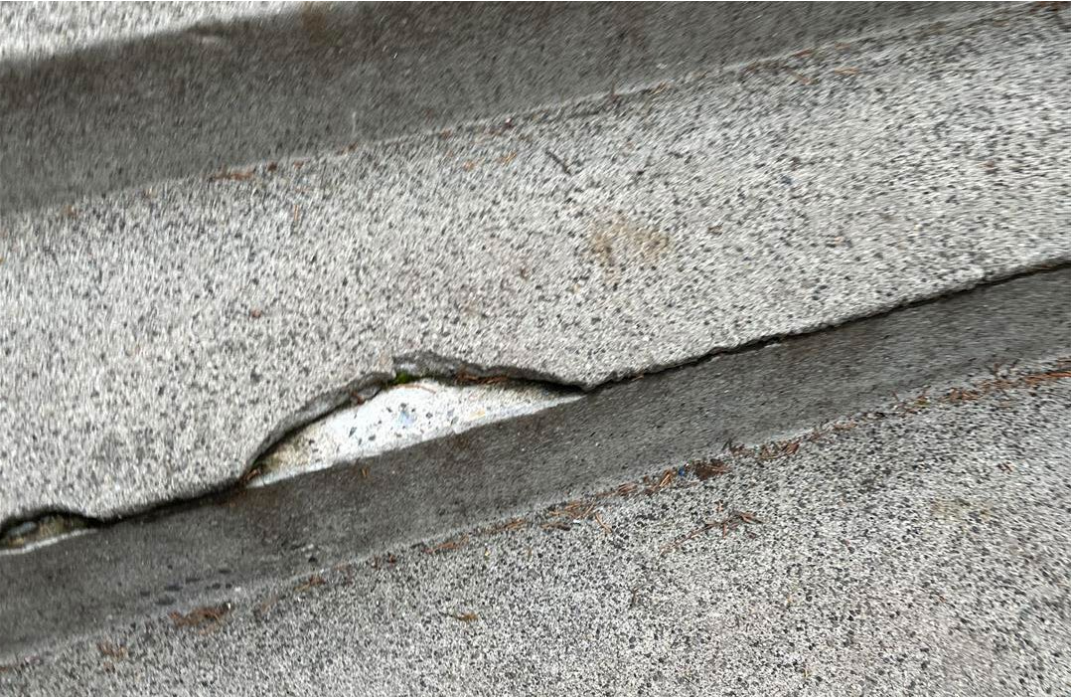
Stair photos taken before construction by DLR Group. November 2021
