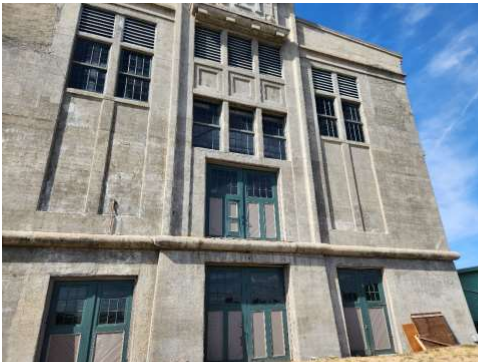
South façade before coating removal
