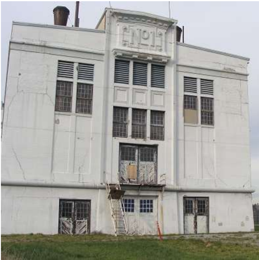
South façade before coating removal
