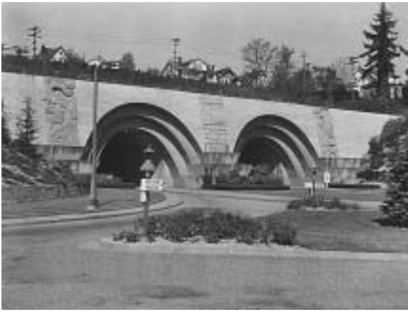
1945 photograph of the tunnels leading to the Lake Washington floating bridge. Source: PEMCO Webster & Stevens Collection, Museum of History and Industry, Seattle. All Rights Reserved.
