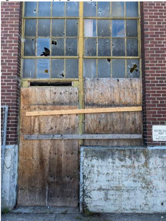
Fig 2.0c: Existing entrance of Building 12, exterior
