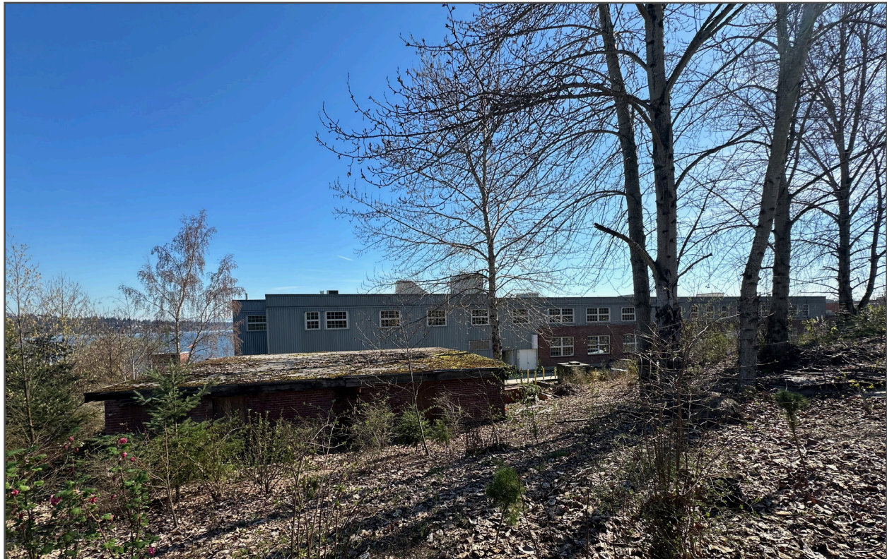
Figure 22 • View of western facade from upper trail
