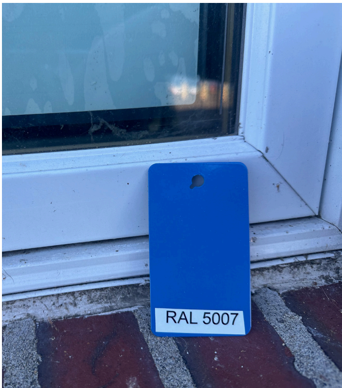
in proximity to other materials on building
