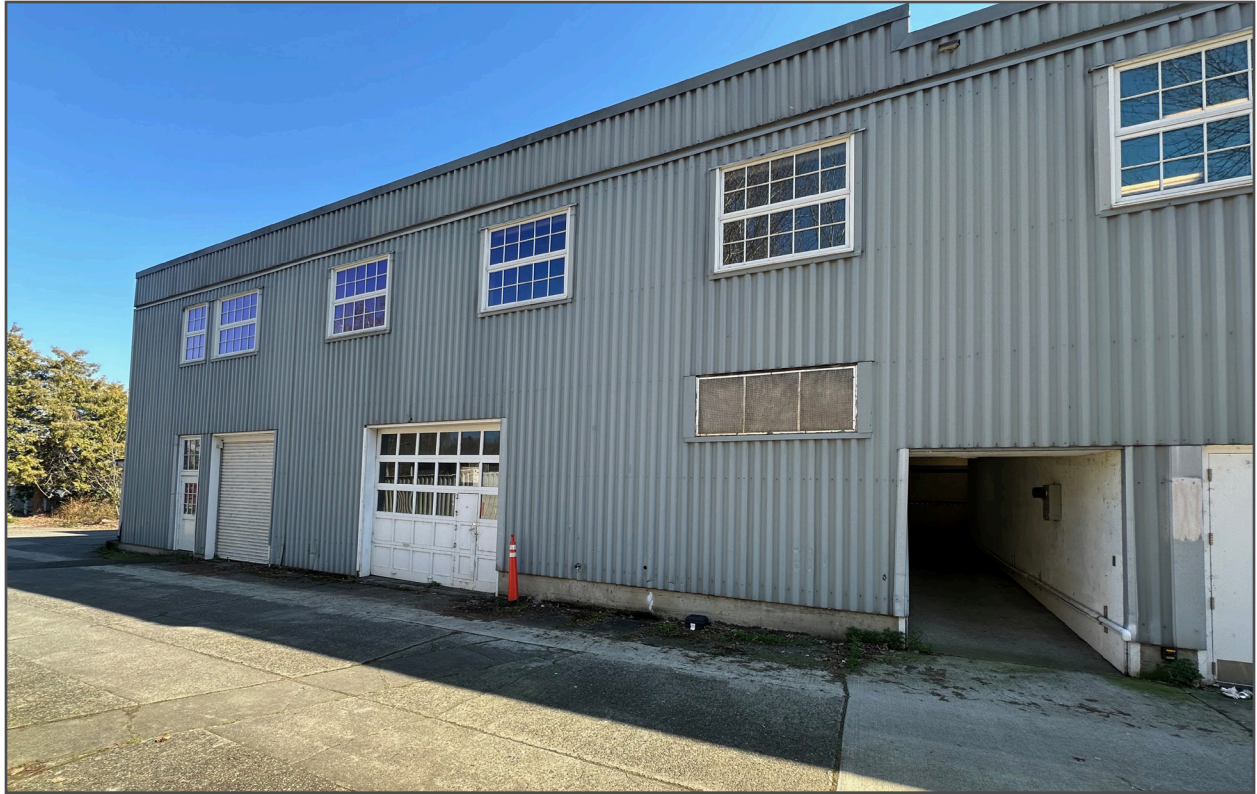
Figure 17 • Western facade, northern end
