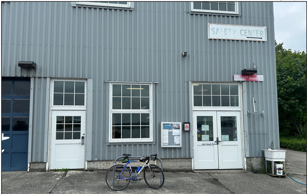
Figure 12 • Eastern facade, detail of northern doors at Sail Sandpoint
