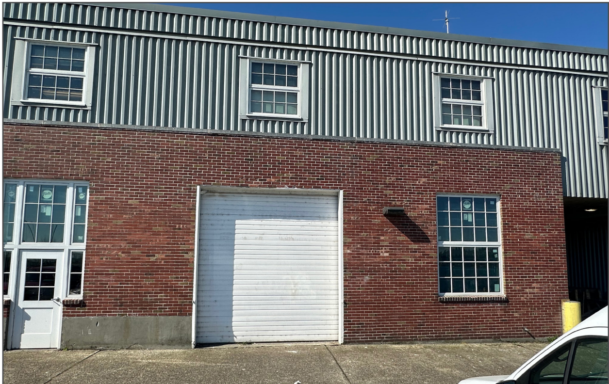
Figure 8 • Eastern facade detail of area for proposed new door
