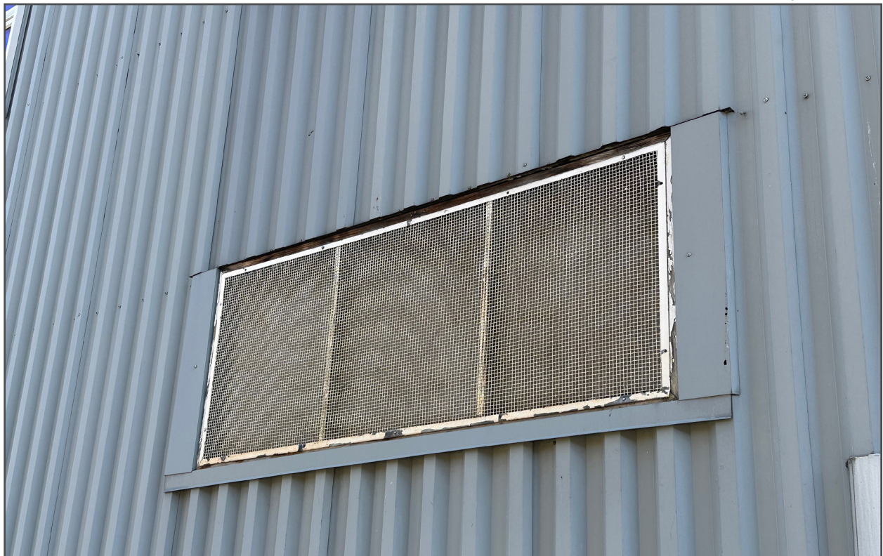
Figure 20 • Detail of screen vent to be re-used
