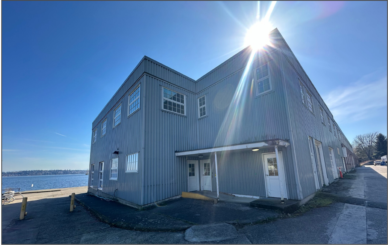
Figure 15 • Northern facade viewing southeast
