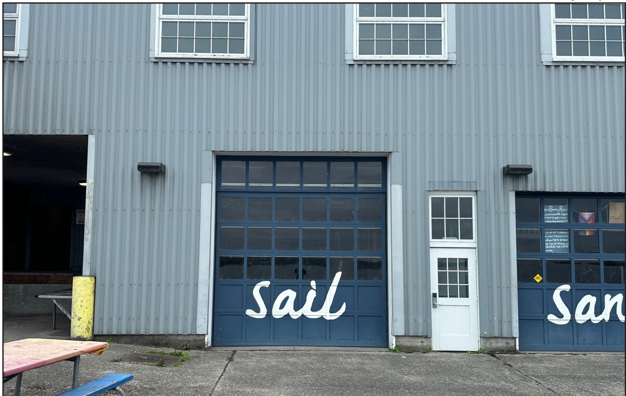
Figure 10 • Eastern facade, detail of Sail Sandpoint doors, southernmost roll-up door and mandoor
