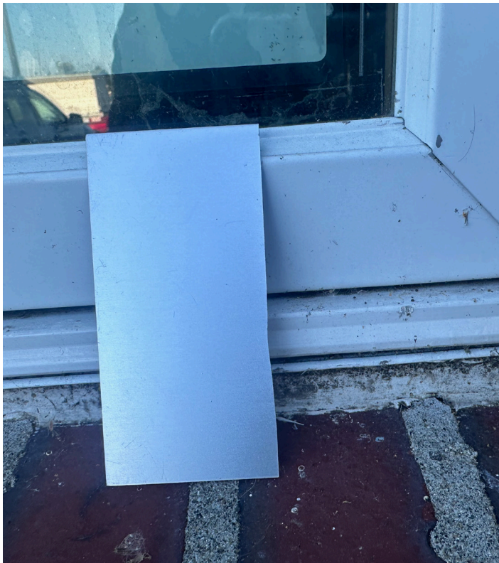
in proximity to other materials on building
