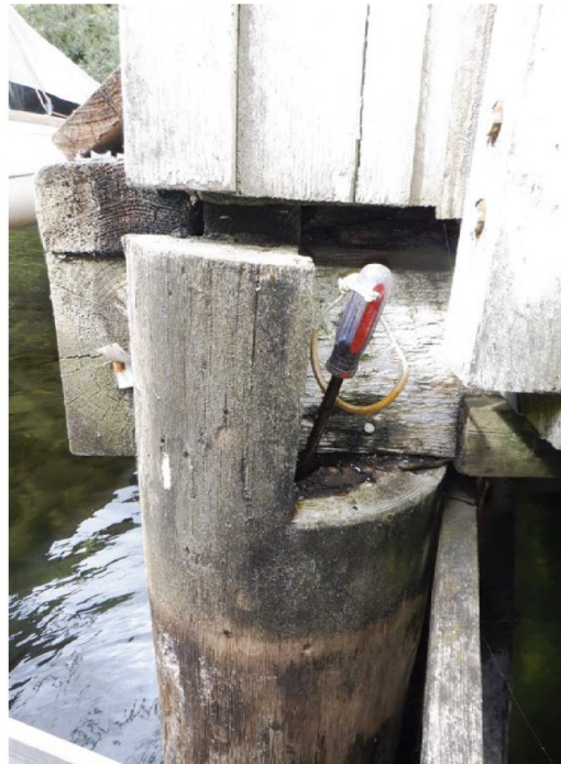
PHOTO No. 25: Building 31, Bent 1, Row A Pile - Note the screwdriver inserted into an ~90% fungal cavity in this pile top. The notching of the pile to provide bearing for the superstructure has exposed the interior of the pile to moisture and subsequent fungal decay.
