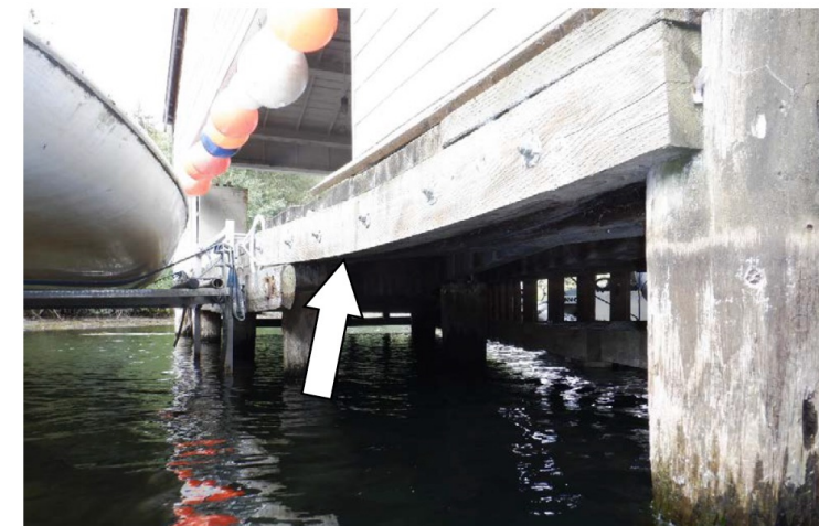
PHOTO No. 16: Building 31, Bent 1, Row A - B Cap - Note the original cap has sustained 90% loss of section due to fungal decay. A temporary repair has been attempted by the installation of two members, one on each side of the heavily damaged member, and thru-bolted. As evidenced by the bowing of the member, this repair appears inadequate for the imposed loads.
