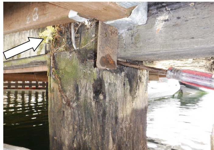
PHOTO No. 26: Building 31, Bent 9, Row A Pile - Note the screwdriver inserted into an area of significant fungal decay. Probing of the area estimated the section loss to be ~50%. Also note the vegetation in the cap timber which provides support for the east building edge (refer to arrow) and the newer treated members supporting the ramp access above.
