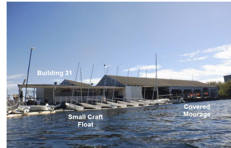
PHOTO No. 15: Building 31 and Covered Moorage, Looking Southeast - This structure is built on untreated timber piles with superstructure of various vintages. The facility also has a Small Craft Float used for moorage of small sailboats.
