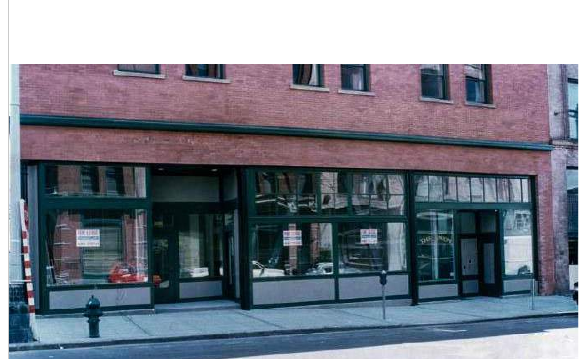
WEST ELEVATION 1994 AFTER RENOVATION
