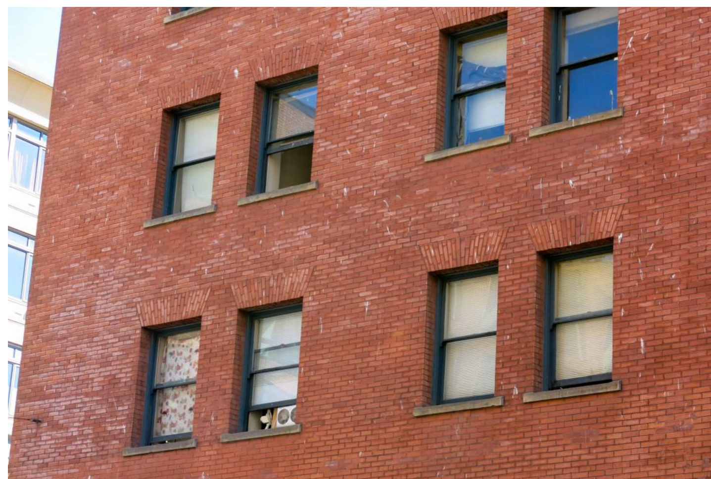
WEST ELEVATION UPPER WINDOWS 2021
