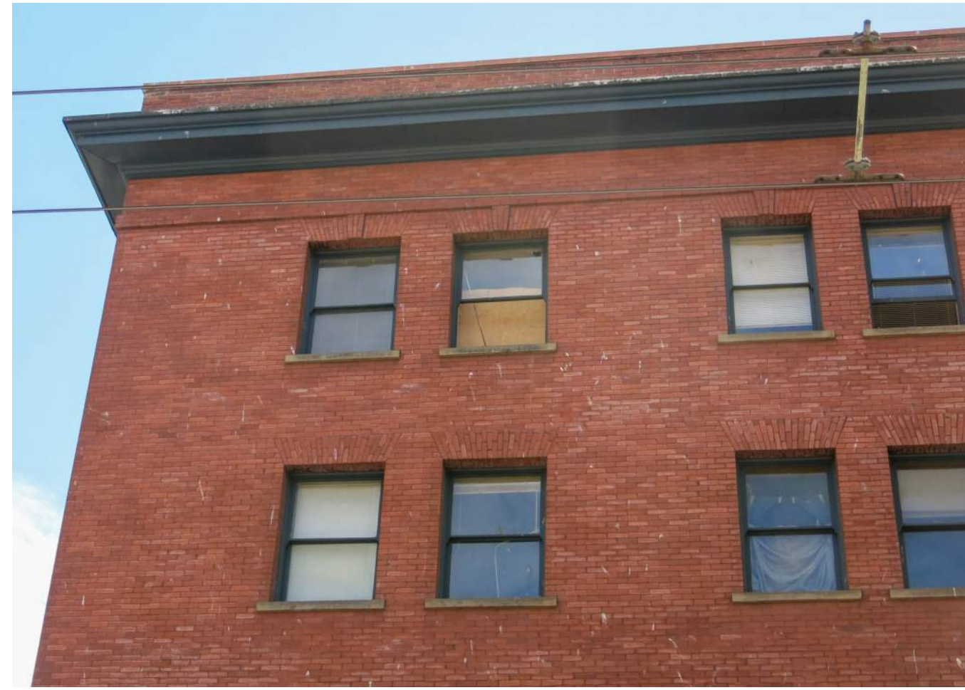
NORTH ELEVATION UPPER WINDOWS 2021
