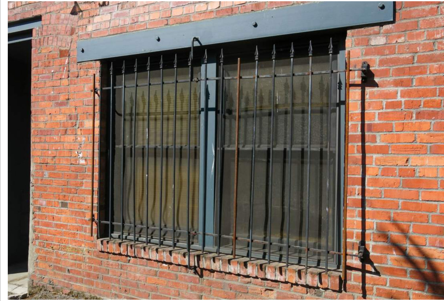
EAST ELEVATION LOWER WINDOWS 2021
