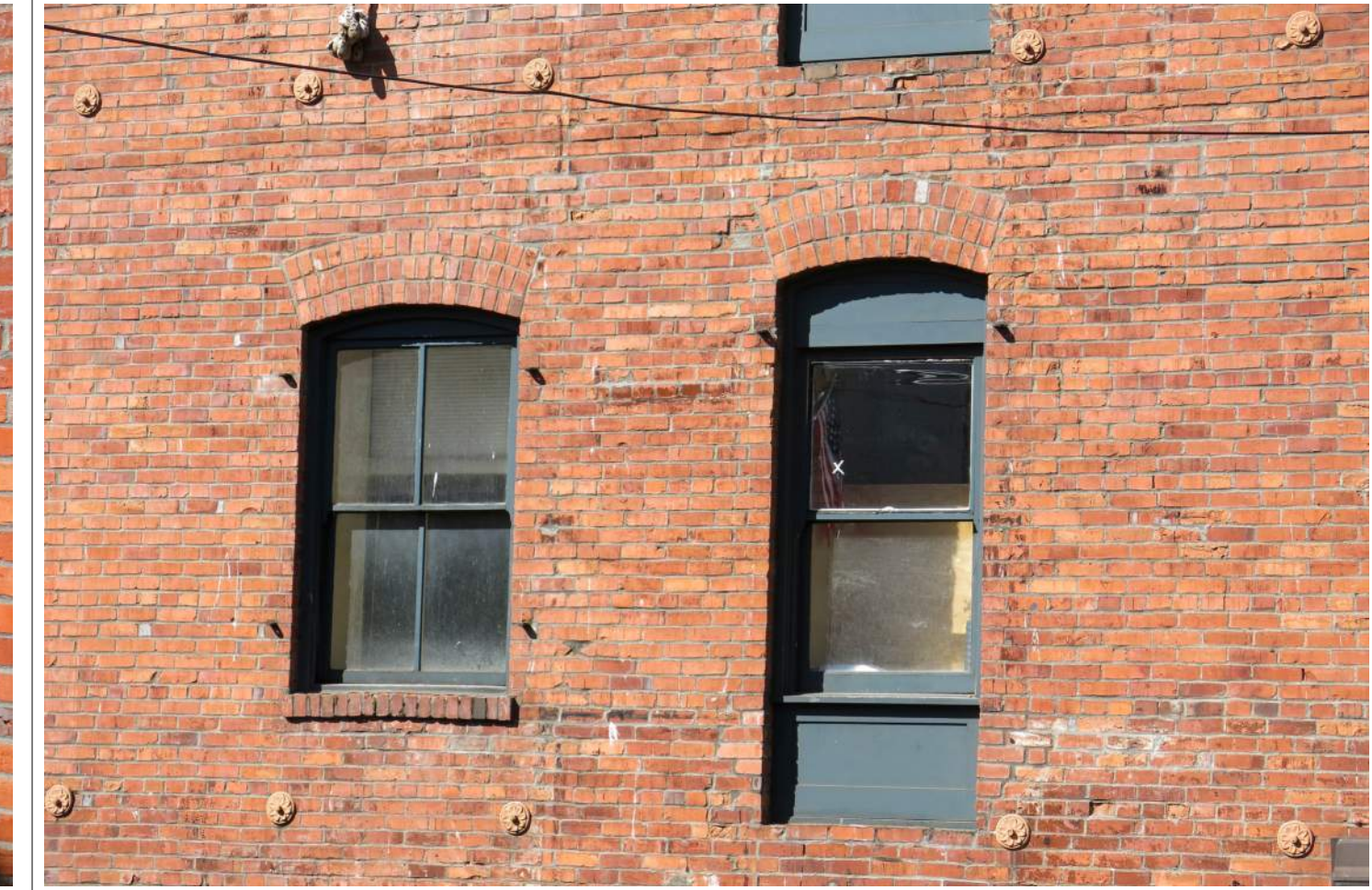
EAST ELEVATION UPPER WINDOWS 2021
