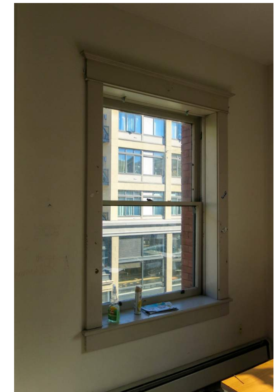
UNIT 411 WINDOW INTERIOR 2021
