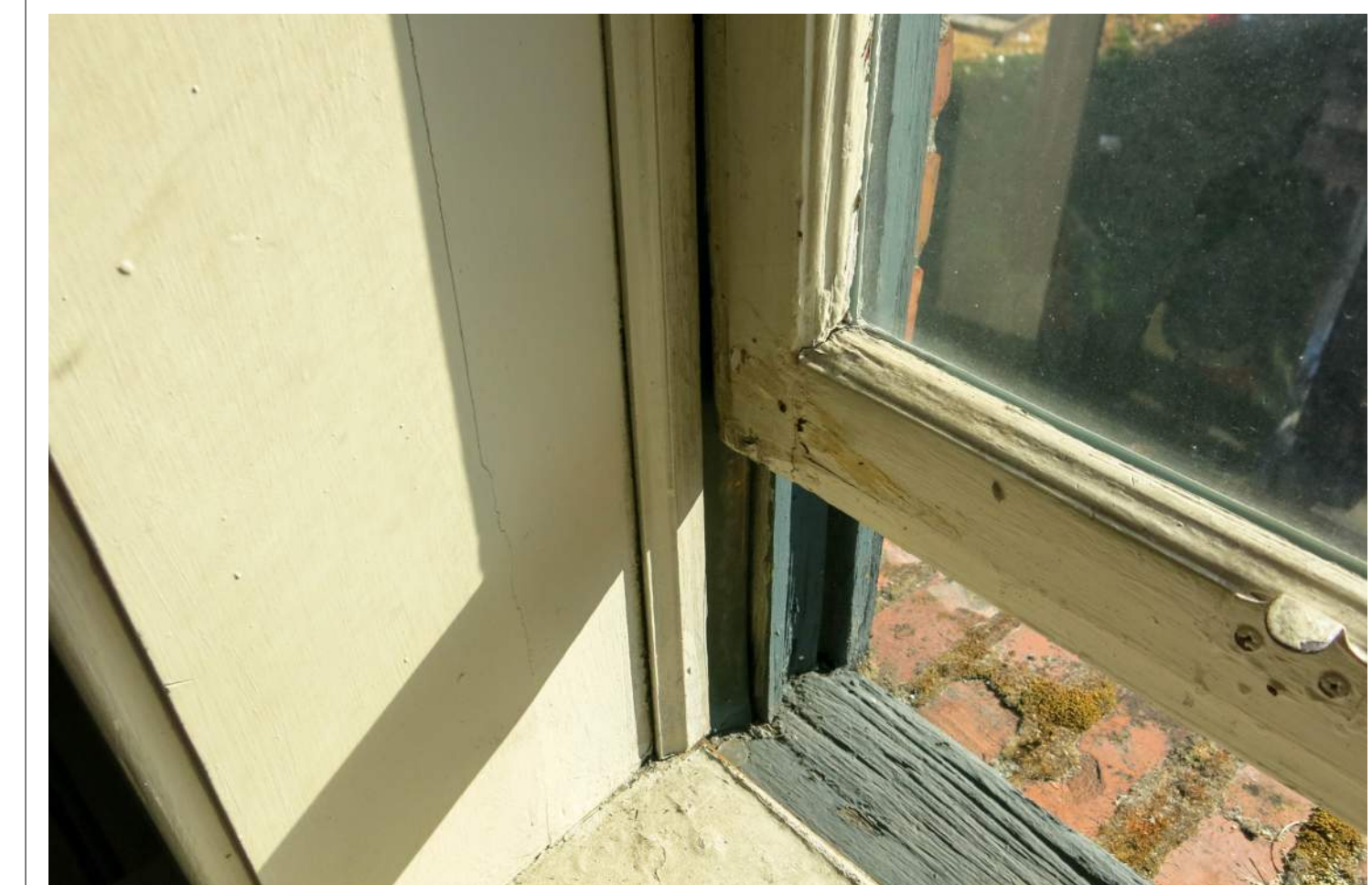
UNIT 407 WINDOW INTERIOR 2021
