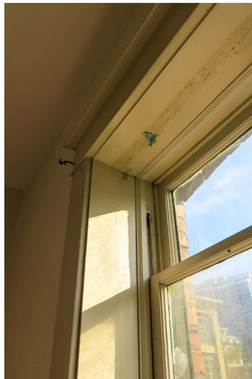
UNIT 411 WINDOW INTERIOR 2021
