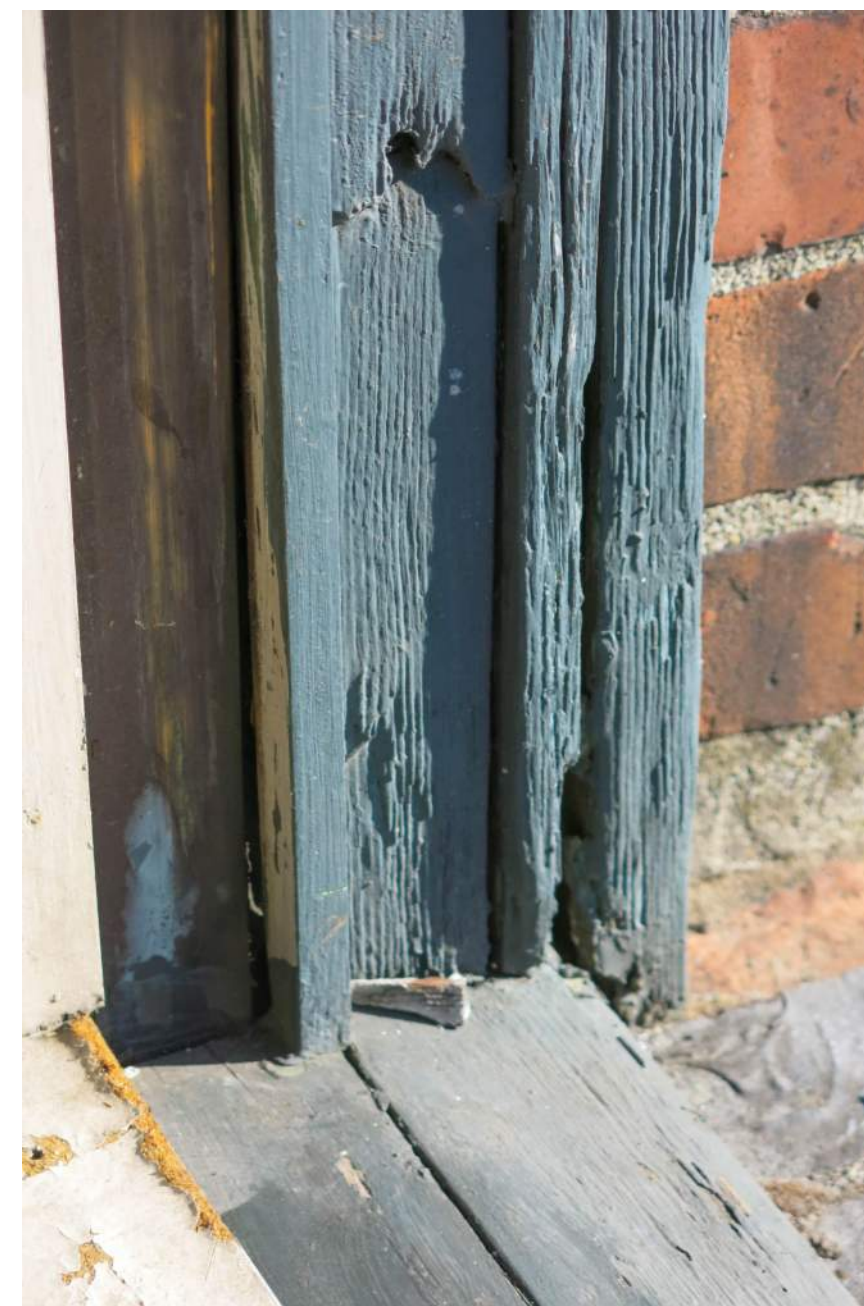
UNIT 411 WINDOW INTERIOR 2021
