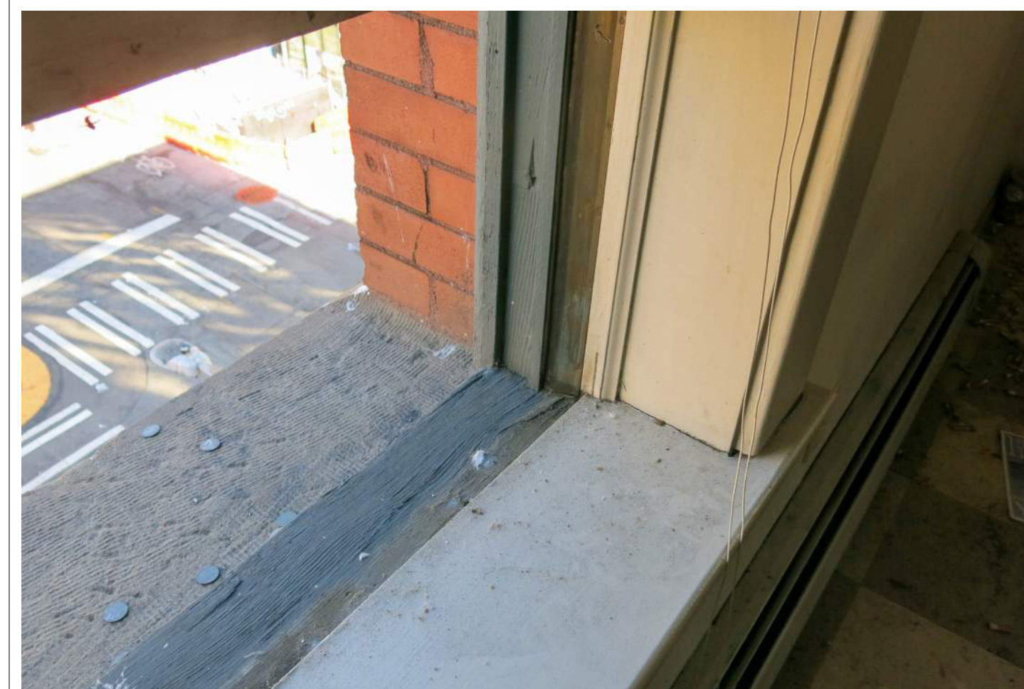
UNIT 401 WINDOW INTERIOR 2021
