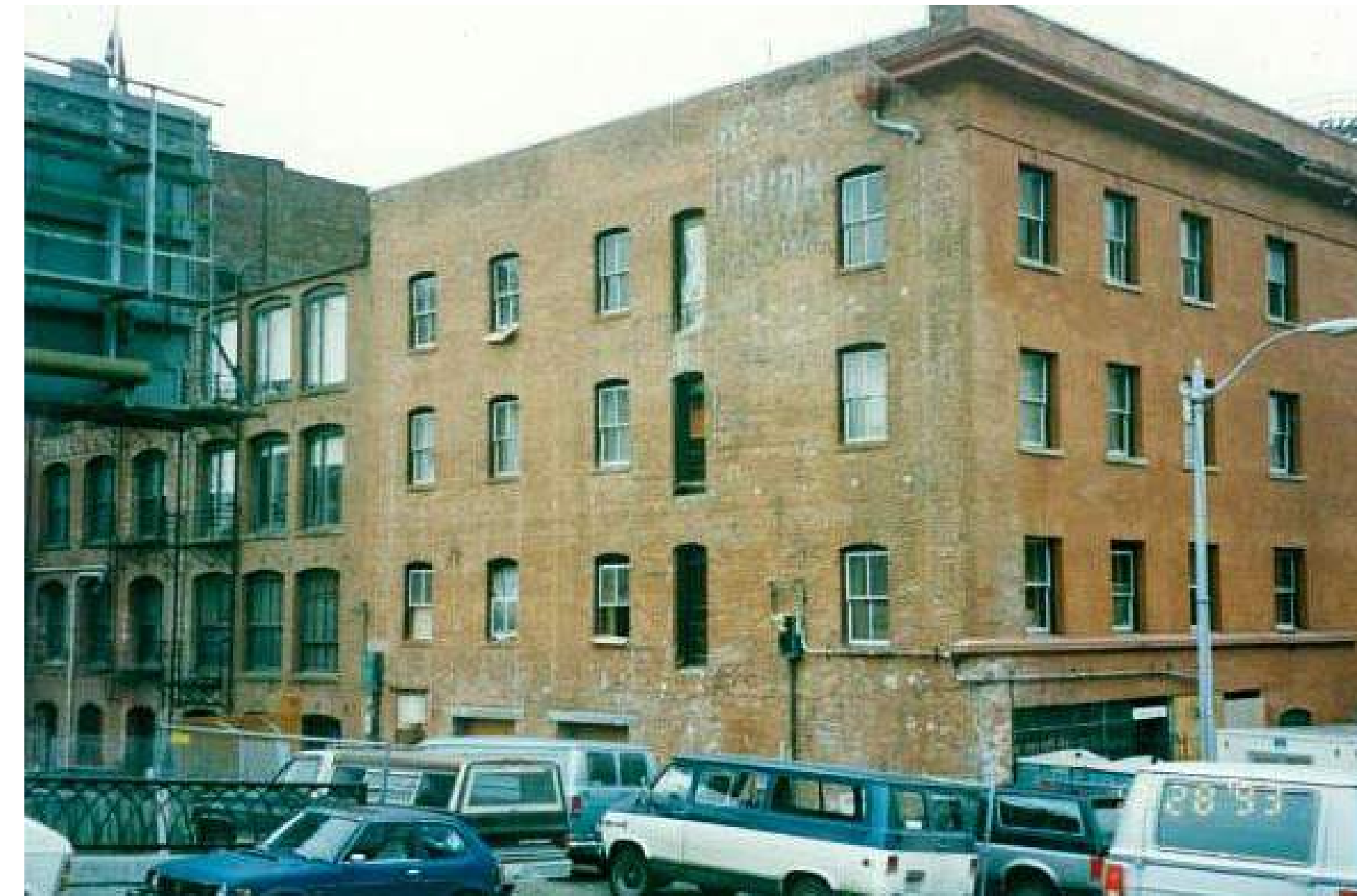
EAST/NORTH ELEVATIONS DURING RENOVATION 1993
