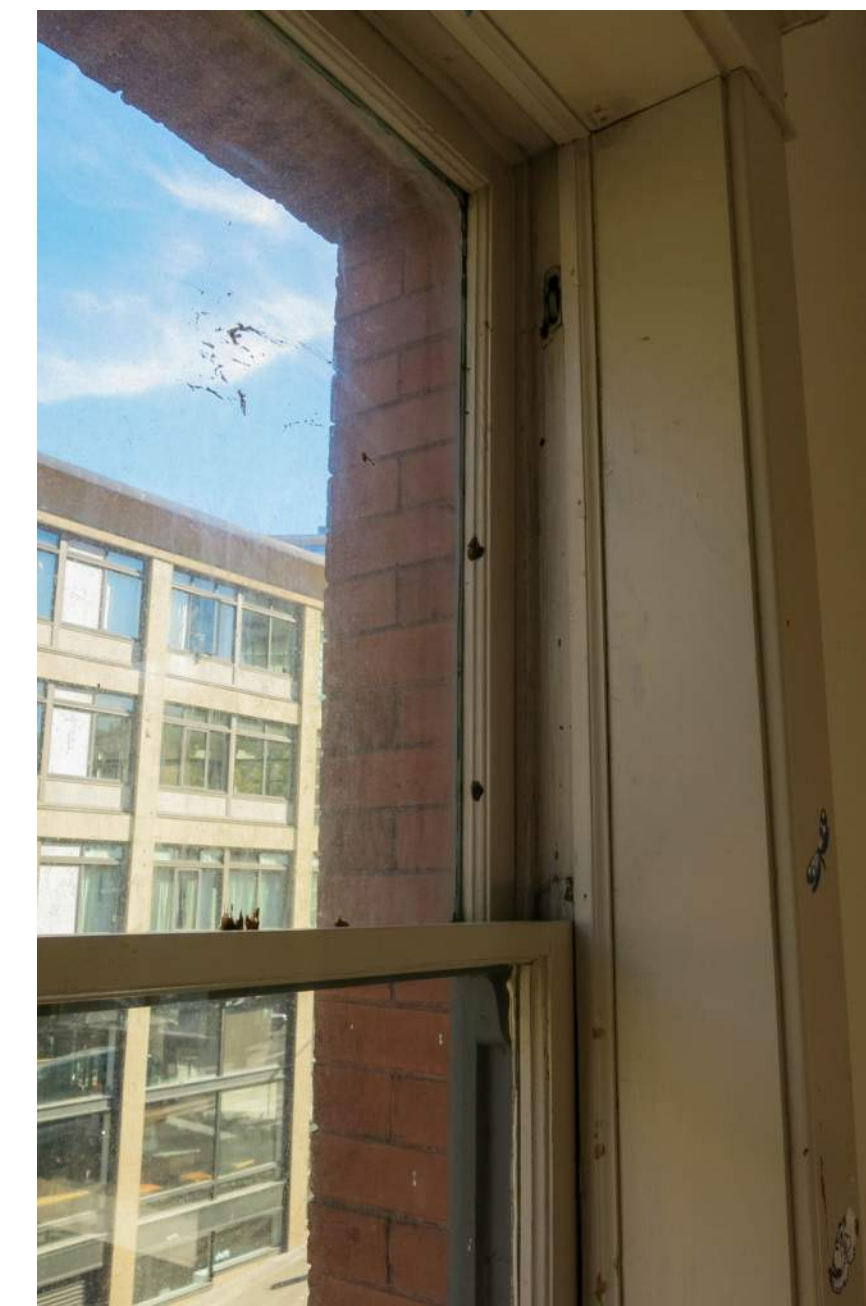
UNIT 411 WINDOW INTERIOR 2021
