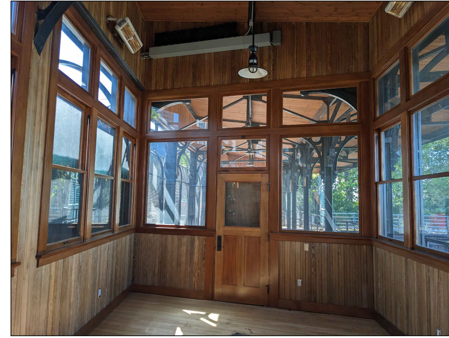
8 INTERIOR - FACING SOUTH NTS
