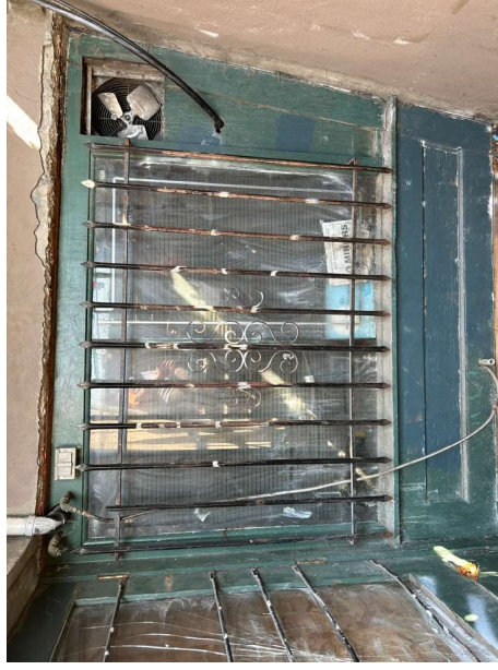
DOOR AND WINDOW WALL AT BOTTOM OF STEPS AT AREAWAY
