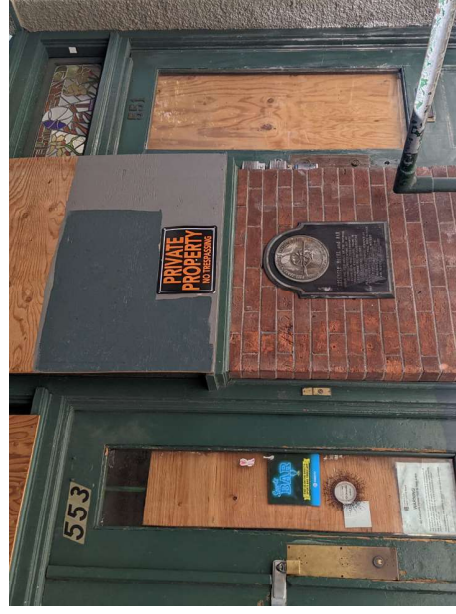
ENTRY TO PUB (LEFT) AND RESIDENCES (RIGHT) WITH STAINED GLASS TRANSOM
