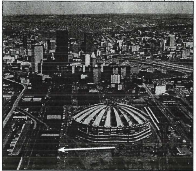
Figure 32 • Aerial View of Kingdome during construction, ca. 1975
