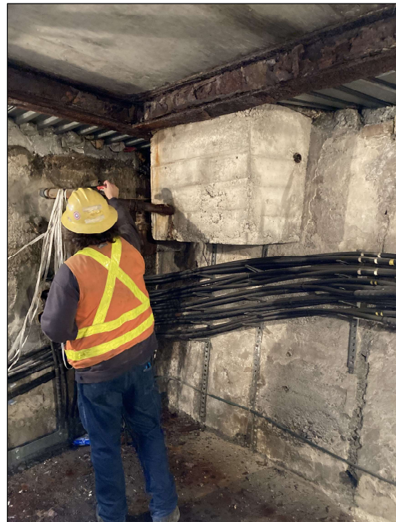
Photo 8 – Northwest corner detail. The ceiling concrete panel has on the exterior surface the small round glass pavers. (Source: SCL, 2022.)
