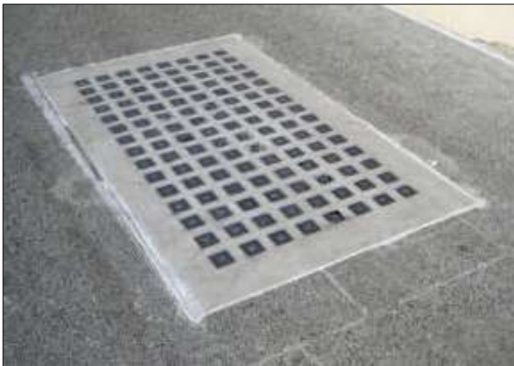
Photo 11 – Examples of vault panels within the Pioneer Square area with square glass pavers. (Source: Seattle City Light, 2023)
